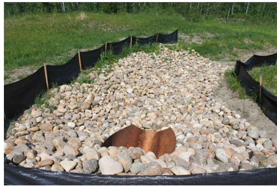
Photo 7. New 1200 mm SWSP culvert outlet installed in June 2021.
