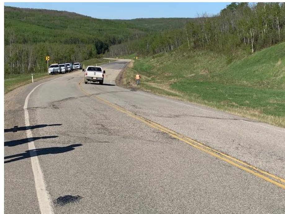
Photo 1. Looking southwest along Hwy (former north slide)
