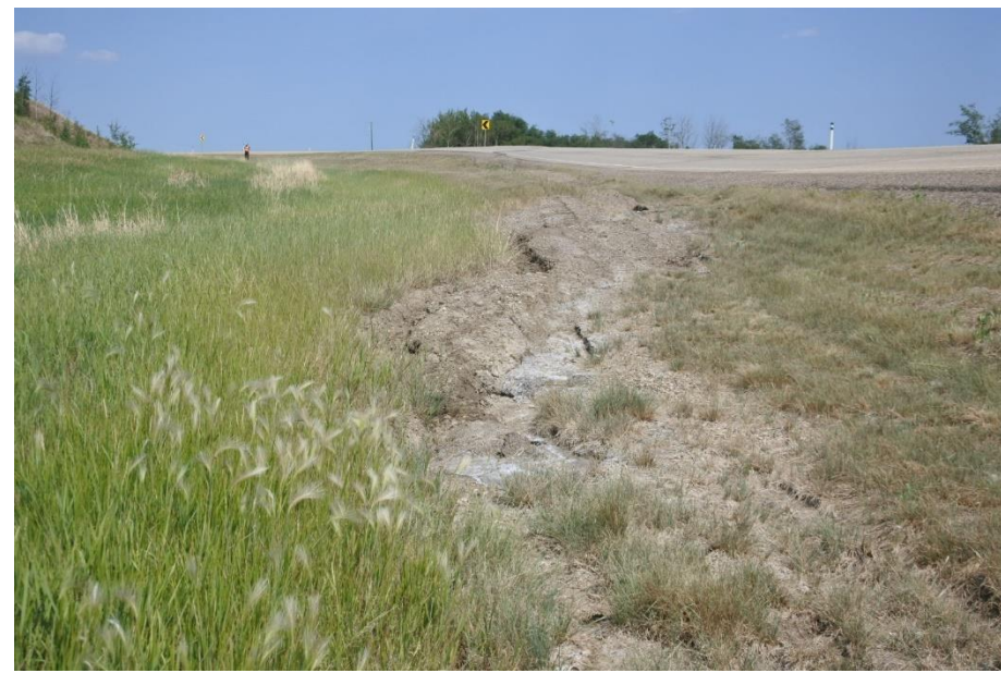
Photo 11. Looking east at what appears to be the scarp meandering off on the northwest side of the highway
