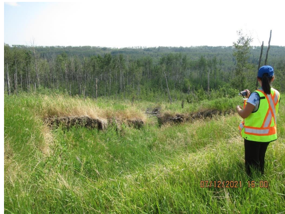
Photo 12. Looking south at erosion gully.
