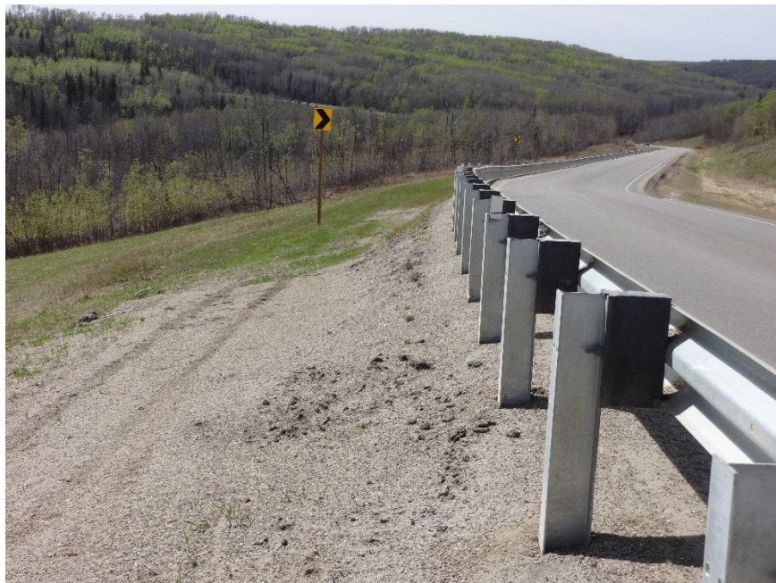
Photo 4. Looking southwest at where gravel had been placed to flatten steep drop off.
