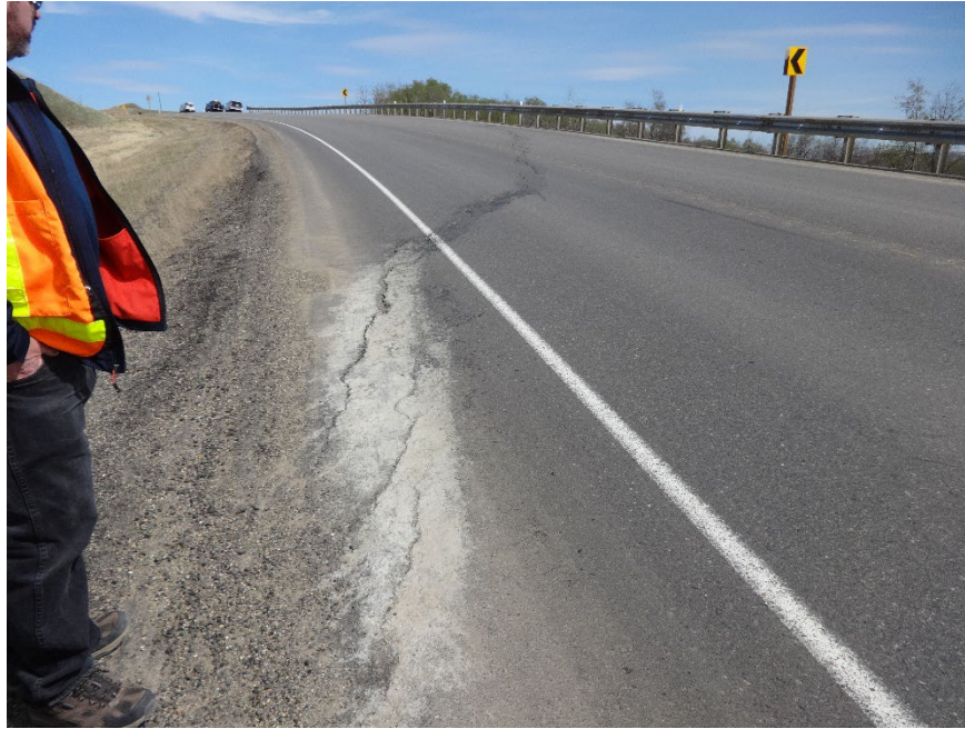
Photo 5. Looking northeast along Hwy 733 at scarp crack
