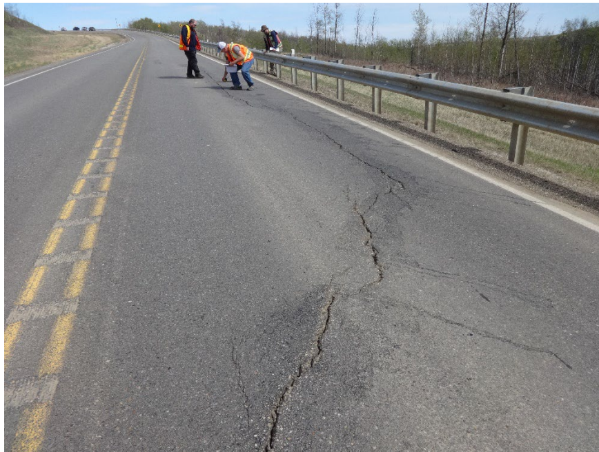
Photo 12. Looking east at scarp crack that was 40 mm wide and had a 20 mm drop.
