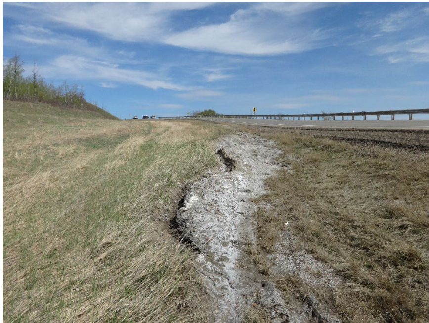
Photo 6. Looking east at scarp crack in the highway ditch with white residue.
