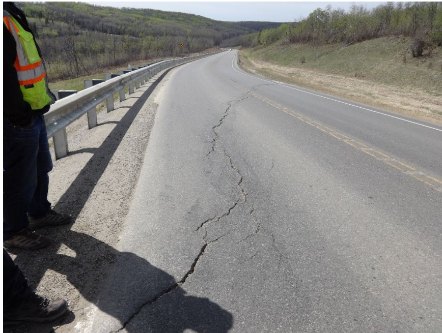
Photo 3. Looking southwest at northmost scarp crack showing through overlay.
