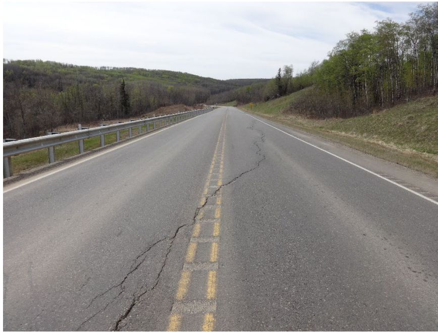
Photo 13. Looking southwest at scarp crack near the westmost part of the site.
