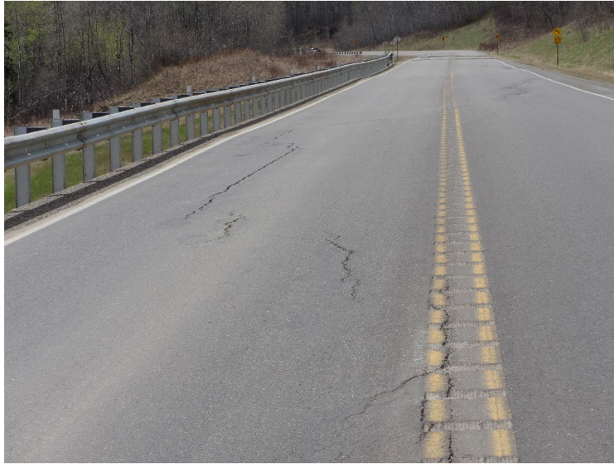
Photo 11. Looking southwest at scarp crack showing through overlay
