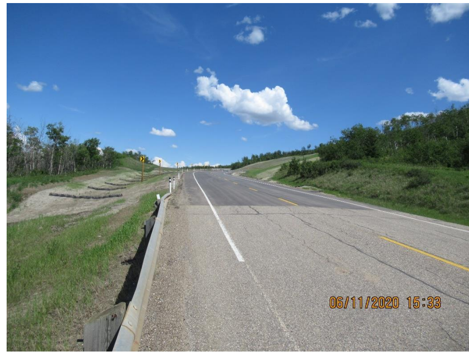
Photo 8. Looking east along Hwy 740 at repaired slide site.
