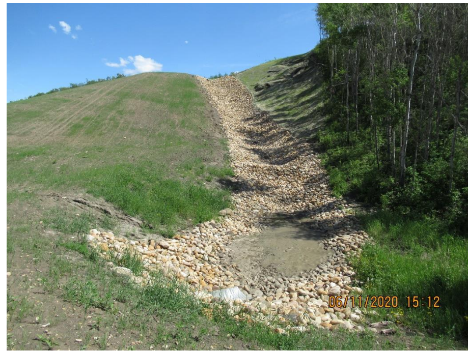
Photo 6. West Riprap Channel. A small slump has formed in the cut slope above the curve of the channel
