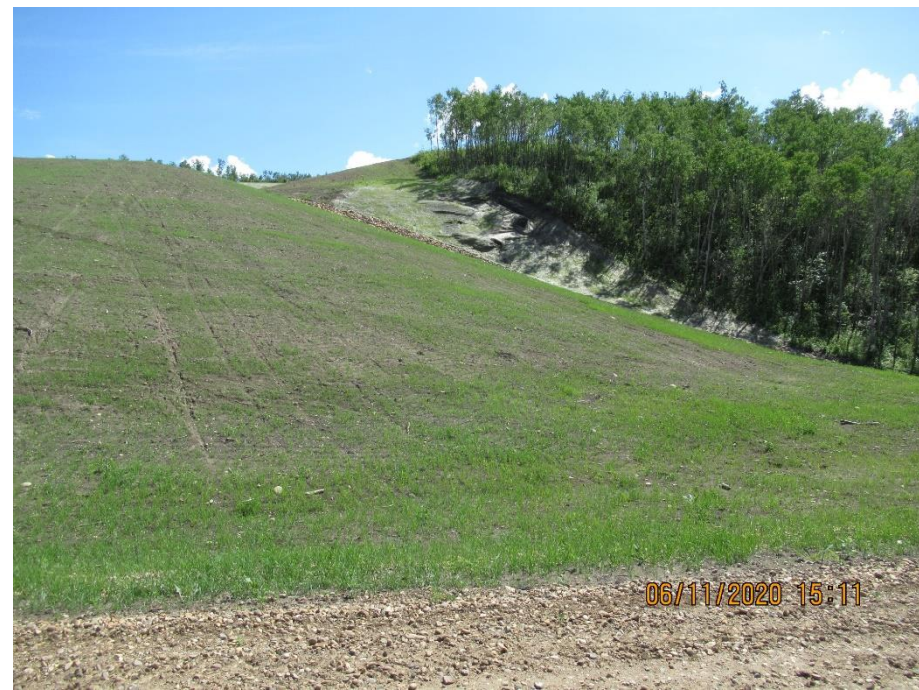
Photo 7. View of slump above channel.
