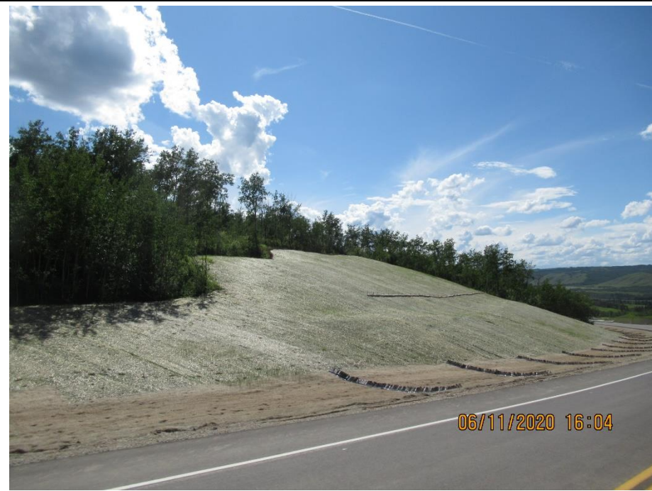
Photo 16. Looking southwest at realigned backslope.
