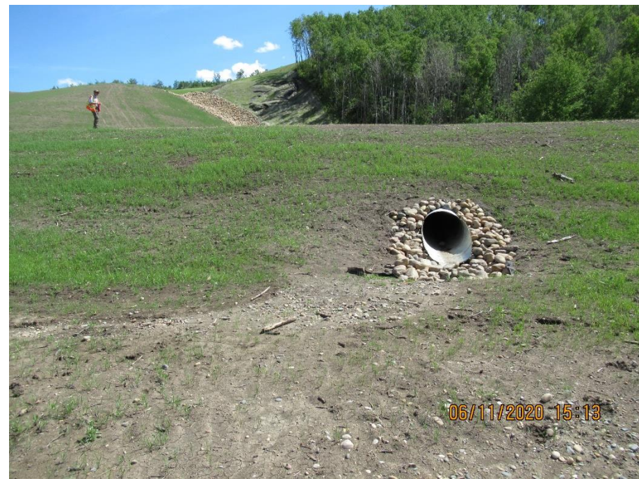
Photo 5. Outlet of culvert draining end of West Riprap Channel.
