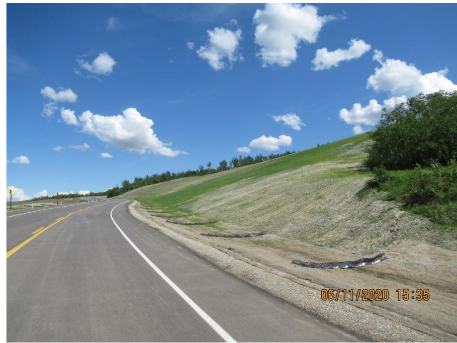
Photo 10. Looking east at new highway realignment.
