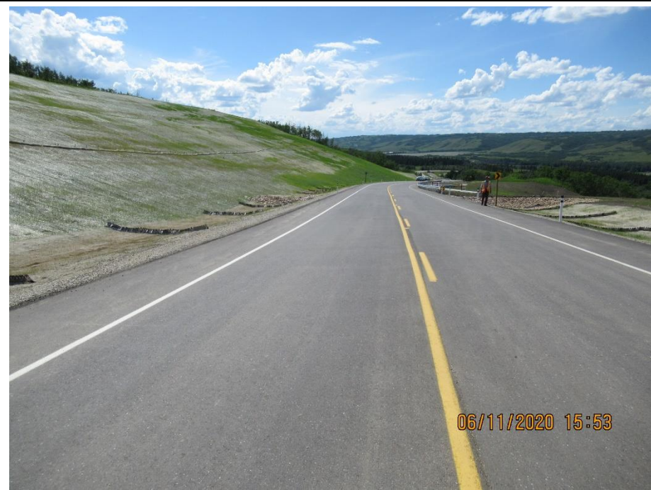
Photo 15. Looking west at realigned highway and backslope.
