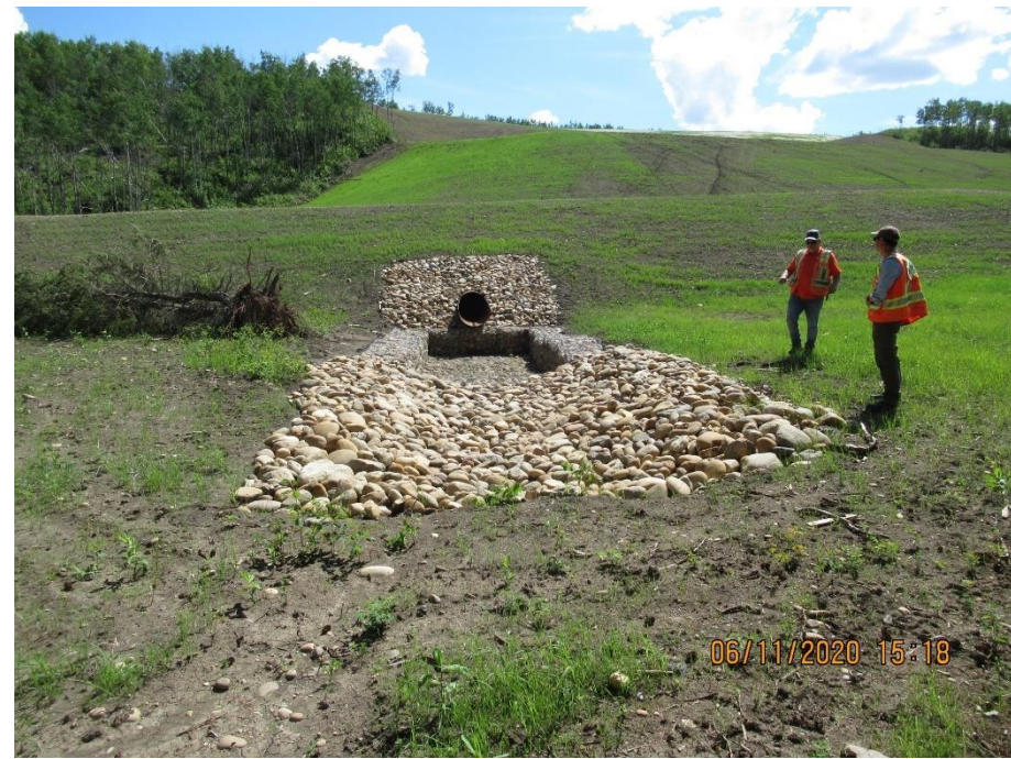
Photo 2. Outfall for SWSP drop pipe performing well to date.
