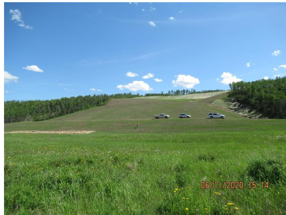
Photo 1. Looking south at the repaired landslide area from the terrace level.
