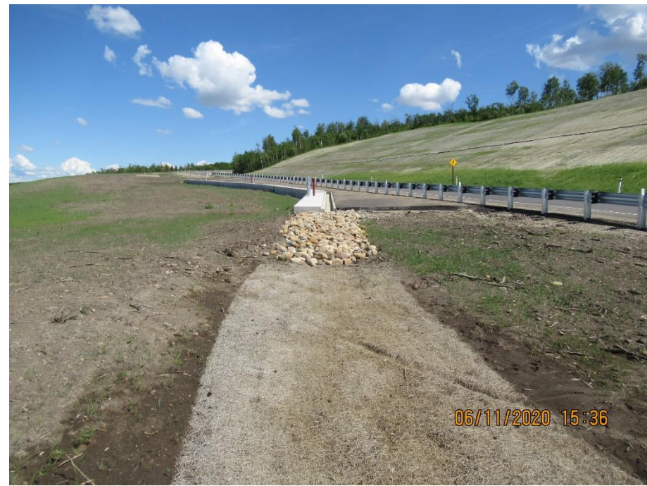
Photo 12. Looking east at pile wall.
