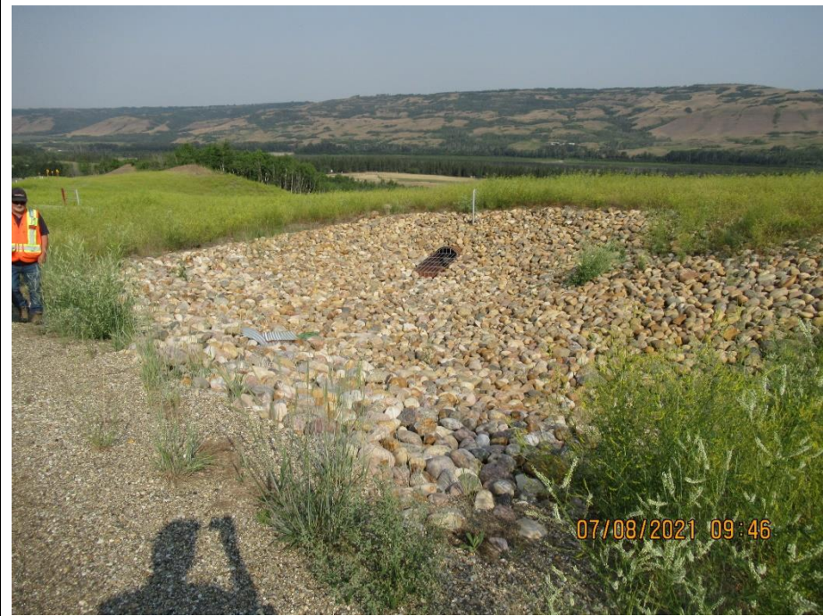
Photo 4. Riprap area at culverts.
