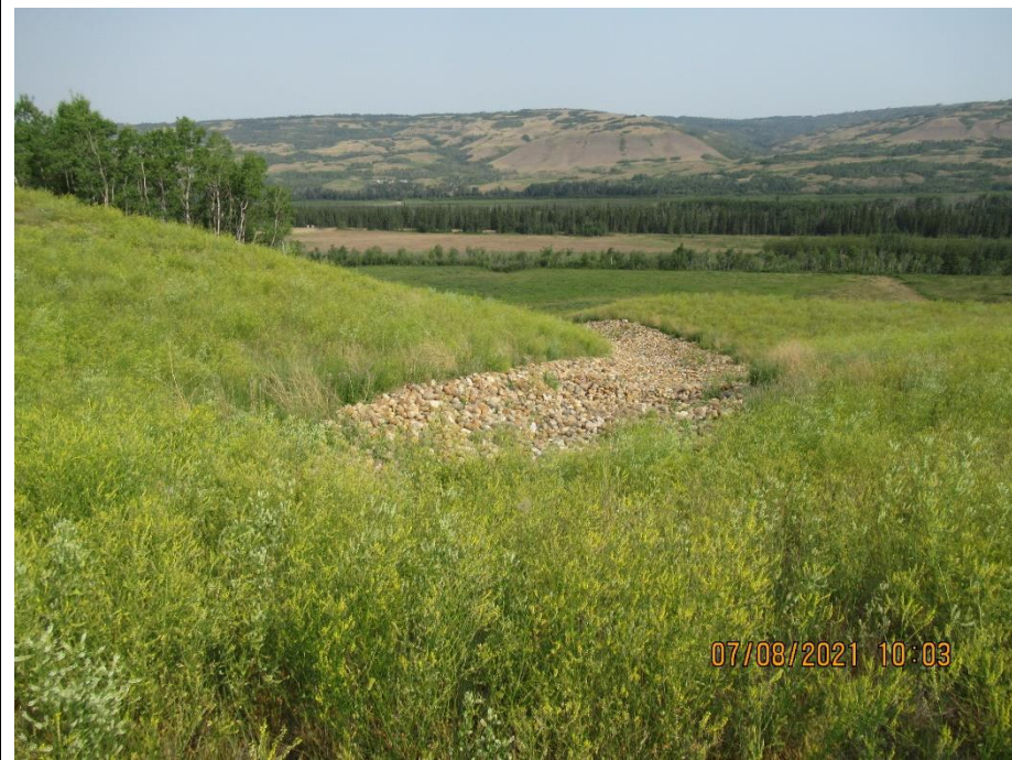
Photo 5. Looking north at West Riprap Channel.
