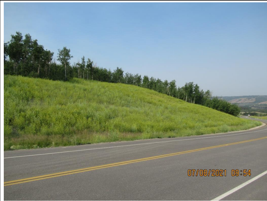
Photo 12. Looking southwest at realigned backslope.
