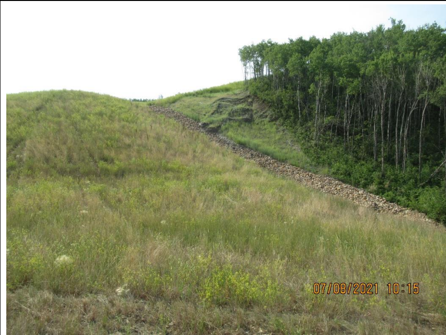
Photo 7. View of slump above West Riprap Channel, looking south.
