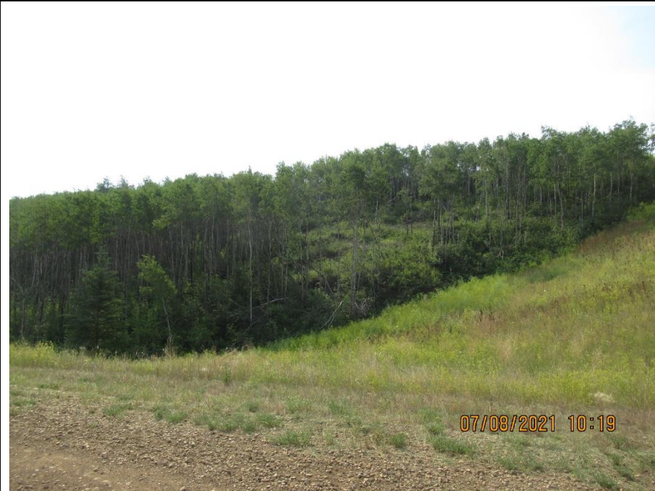
Photo 10. Looking southeast at landslide in natural forested slope.
