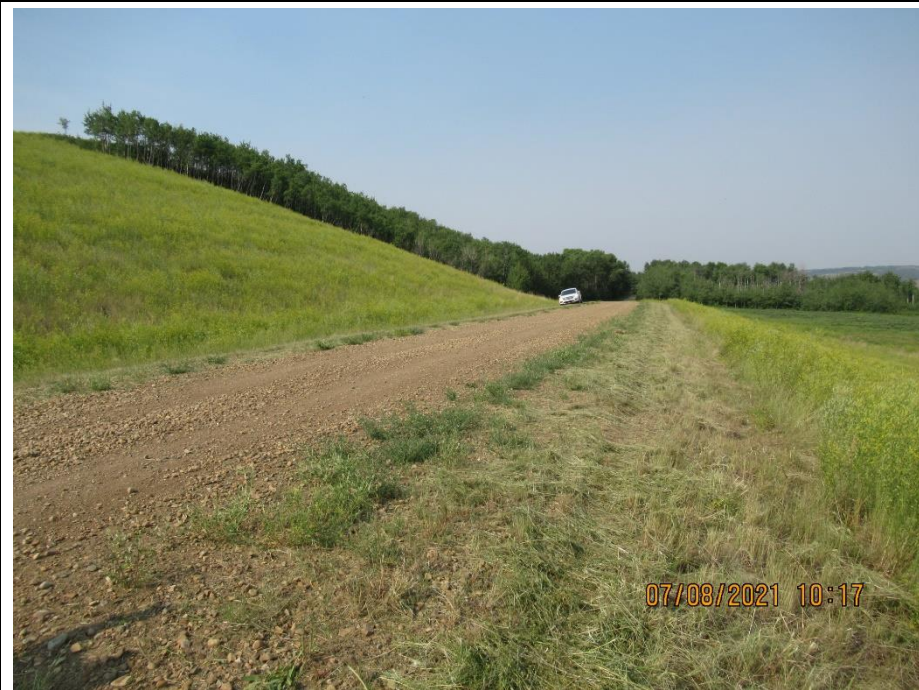
Photo 8. Looking west along County road over toe berm.
