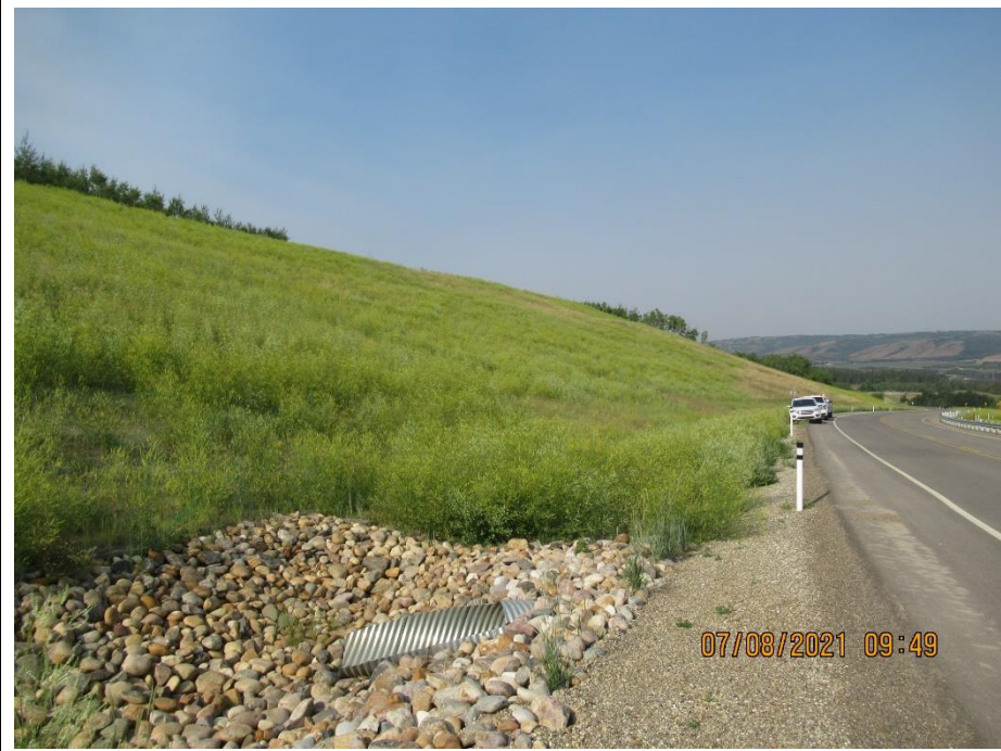
Photo 1. Looking west at the backslope of the repaired landslide area.
