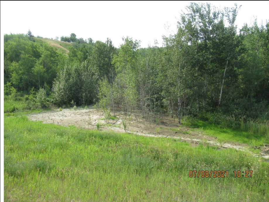
Photo 11. Silty runoff accumulating in low area south of highway. Not related to the landslide repairs
