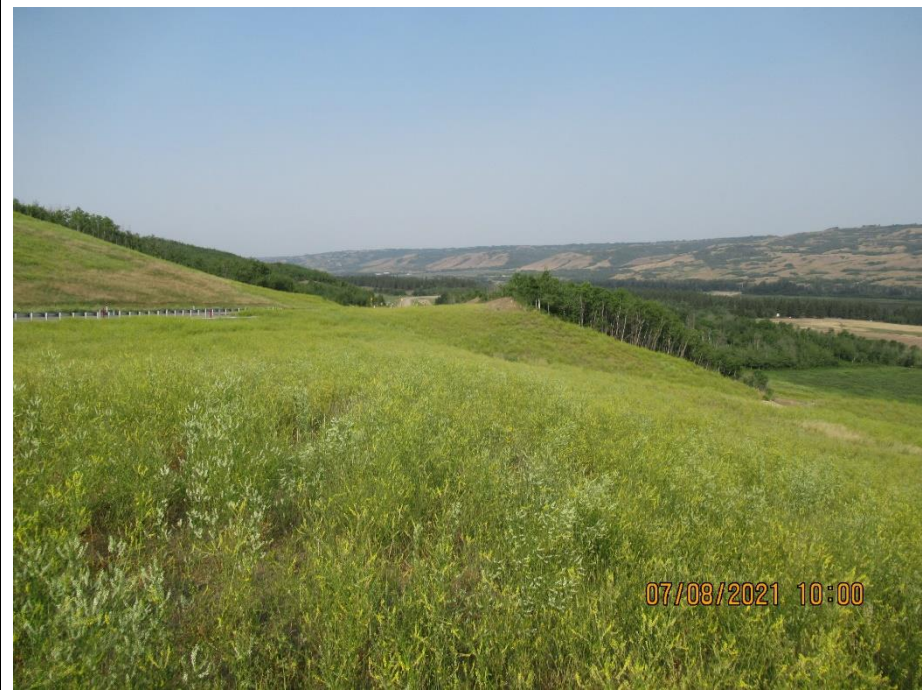
Photo 3. Looking west at the grass covered slope below the pile wall.
