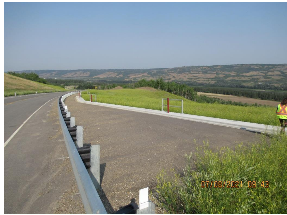
Photo 2. Looking west at the pile wall.
