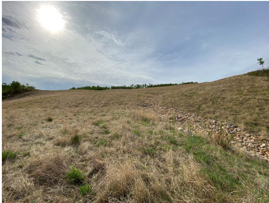
Photo 11. Looking south at upper slope and west riprap channel. No change in the shallow slump condition. It is grassed over.
