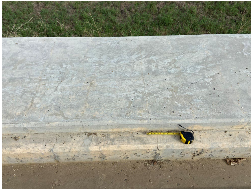
Photo 9. Thermal cracks in the top of the concrete waler of the pile wall.
