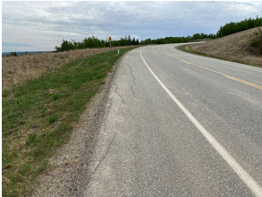
Photo 6. Looking east at the cracks in the north shoulder of the road pavement.
