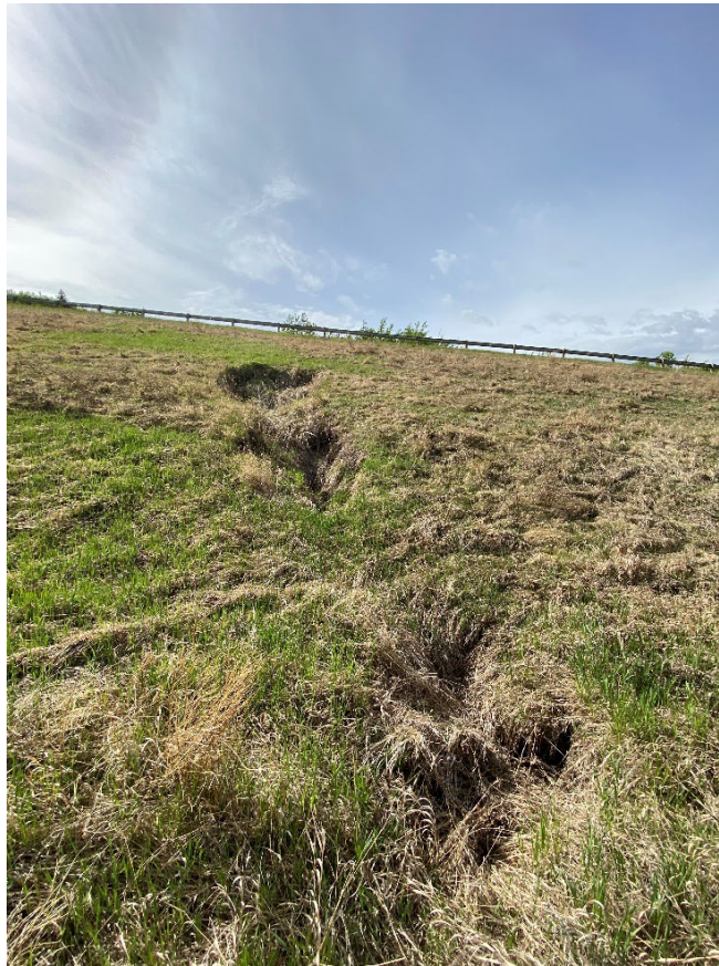
Photo 15. Looking south at the erosion gully downslope of the culvert outlet.
