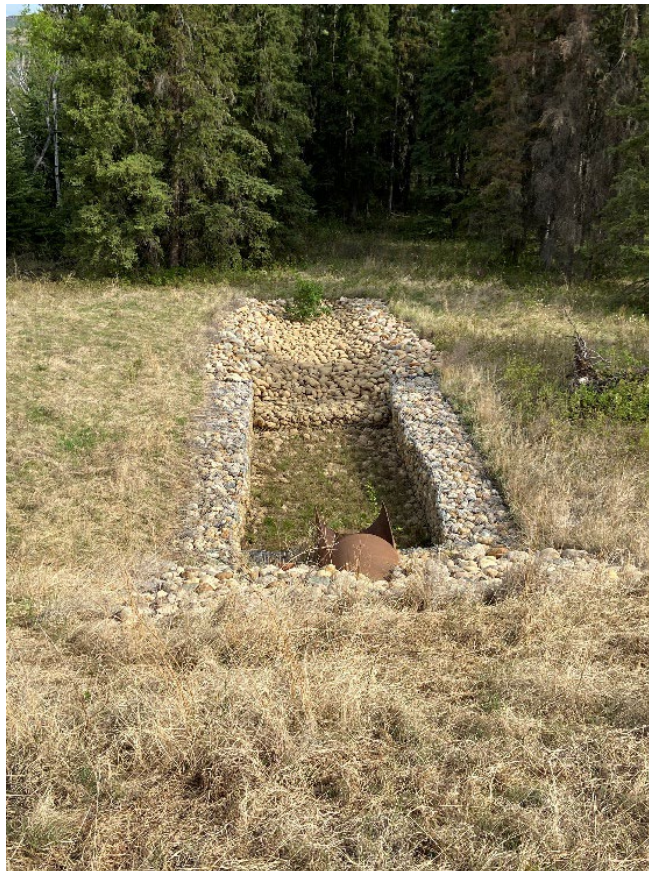
Photo 12. Looking north at drop pipe outlet – in good condition.
