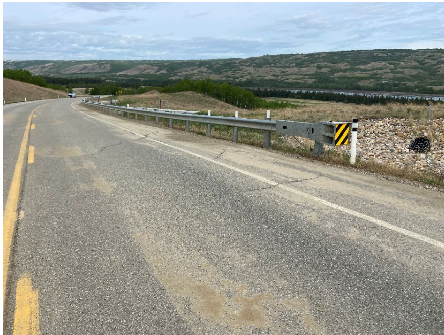
Photo 3. Looking west at cracks in road beyond east end of pile wall.
