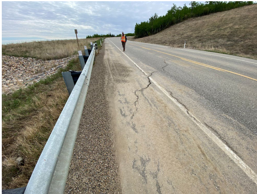
Photo 4. Looking east at cracks in pavement beyond east end of pile wall.
