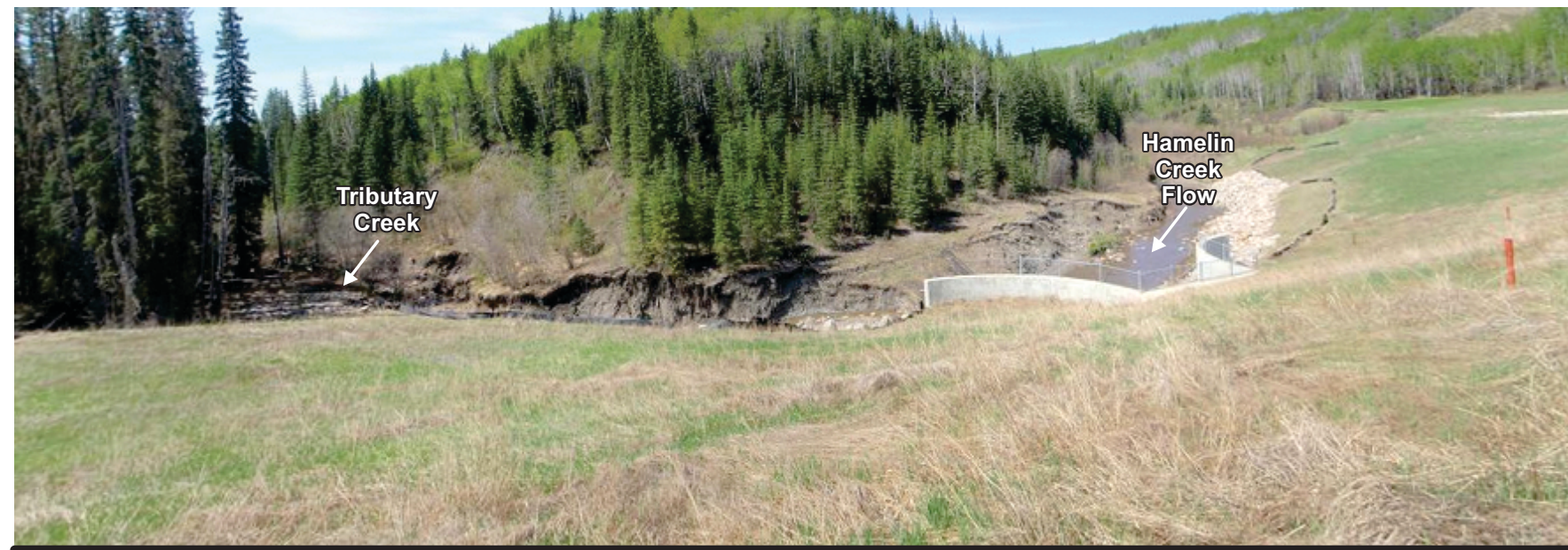
Photo 3 Looking upstream at Hamelin Creek and at Tributary Creek • Opposite bank and valley slope of Hamelin Creek was eroded steeply • Bank on highway side well protected by recent (2010) bank armouring • Previous (2010) repair work on upstream side of site still in good condition • Culvert Inlet and channel thorough-way looked unblocked
