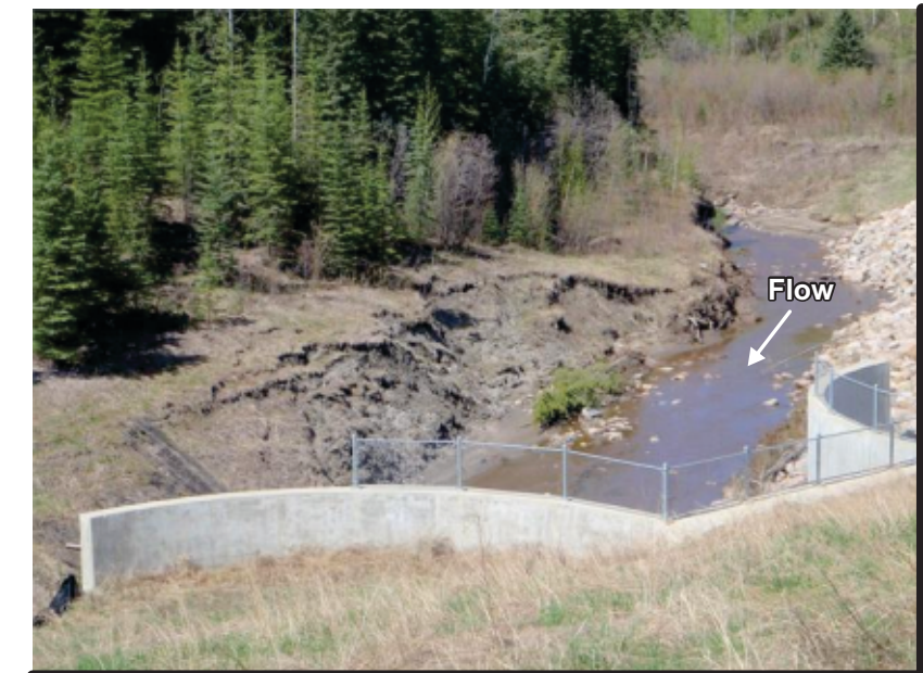
Photo 3a Looking upstream at Hamelin Creek and at Tributary Creek • Opposite bank and valley slope of Hamelin Creek was eroded steeply • Bank on highway side well protected by recent (2010) bank armouring • Previous (2010) repair work on upstream side of site still in good condition • Culvert Inlet and channel thorough-way looked unblocked
