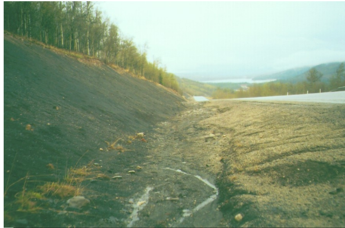
Photo 9 Looking downgrade south ditch erosion mildly severe along 3rd stretch of 100m downgrade.
