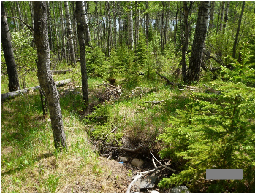
Photo 4 Erosion channel downstream of single culvert outlet on south side of Hwy 40:34. Photo taken June 2, 2025, facing southeast near WP031.
