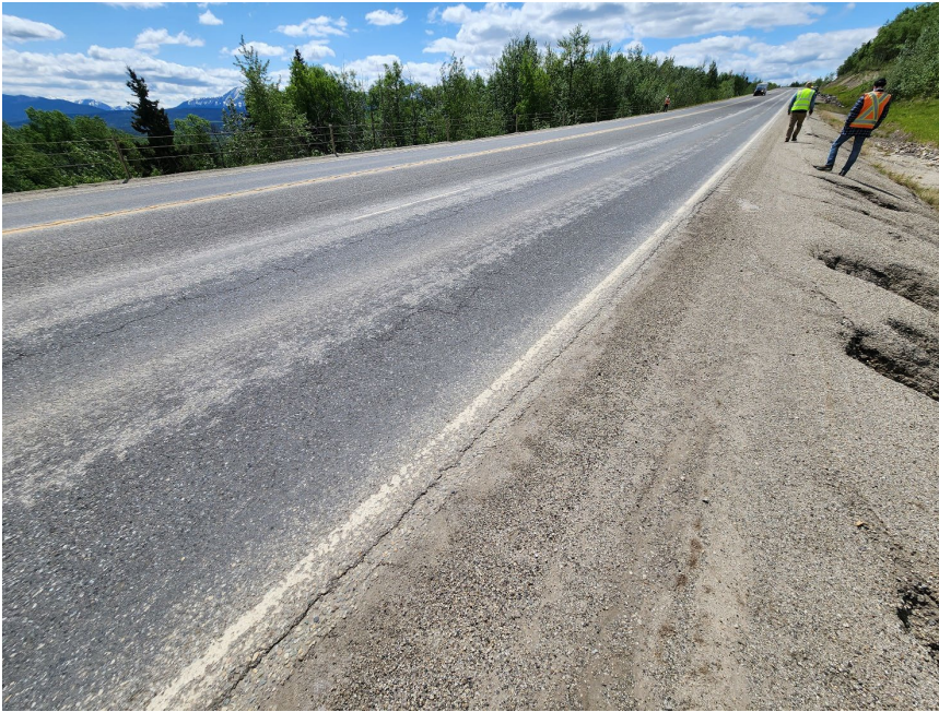
Photo 8 Ditch on north side of Hwy 40:34. Note erosion in ditch channel and twinned culvert inlets (WP028). Photo taken June 2, 2025, facing southwest.
