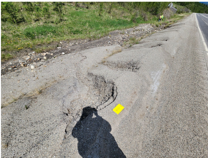
Photo 6 Ditch on north side of Hwy 40:34. Note erosion in ditch channel and erosion features along north highway shoulder at edge of pavement. Photo taken June 2, 2025, facing northeast.
