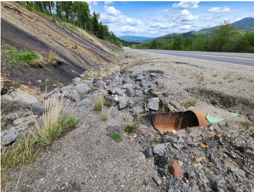
Photo 2 Ditch on north side of Hwy 40:34. Note deterioration of riprap in ditch channel, and erosion / material in ditch channel that appears to divert flow around single culvert inlet (WP030). Photo taken June 2, 2025, facing northeast.
