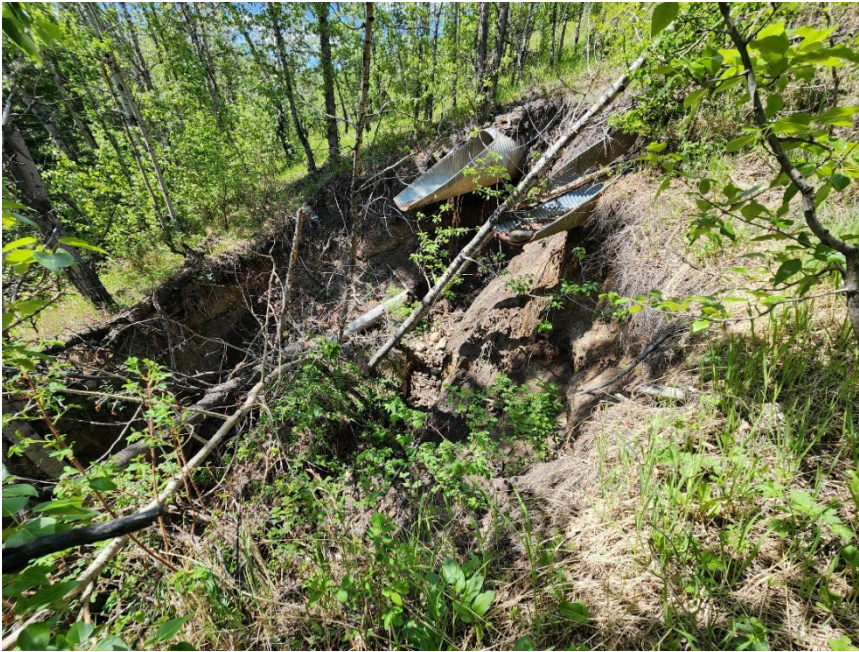
Photo 10 Erosion channel downstream of twinned culvert outlets on south side of Hwy 40:34. Photo taken June 2, 2025, facing southwest.
