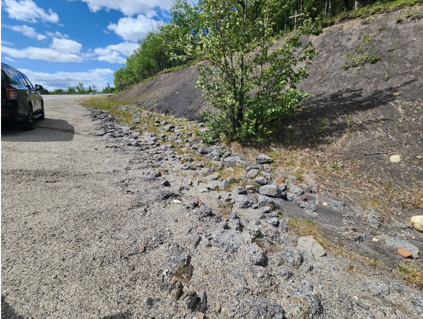
Photo 2 Ditch on north side of Hwy 40:34. Note deterioration of riprap in ditch channel, and erosion / material in ditch channel that appears to divert flow around single culvert inlet (WP030). Photo taken June 2, 2025, facing northeast.
