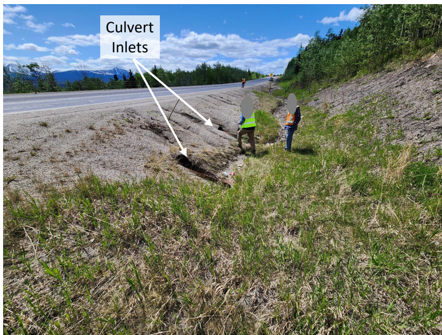
Photo 8 Ditch on north side of Hwy 40:34. Note erosion in ditch channel and twinned culvert inlets (WP028). Photo taken June 2, 2025, facing southwest.
