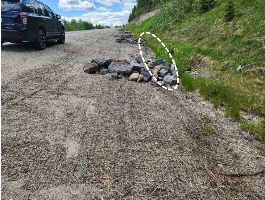
Photo 6 Ditch on north side of Hwy 40:34. Note erosion in ditch channel and erosion features along north highway shoulder at edge of pavement. Photo taken June 2, 2025, facing northeast.
