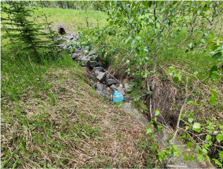
Photo 4 Erosion channel downstream of single culvert outlet on south side of Hwy 40:34. Photo taken June 2, 2025, facing southeast near WP031.
