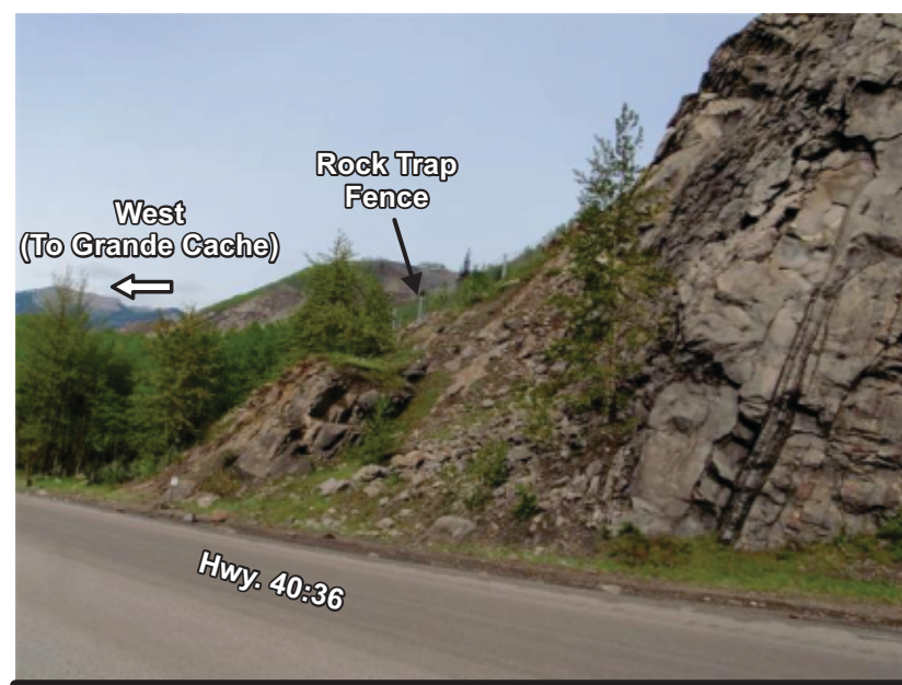
Photo 2b Close up of rock trap fence
