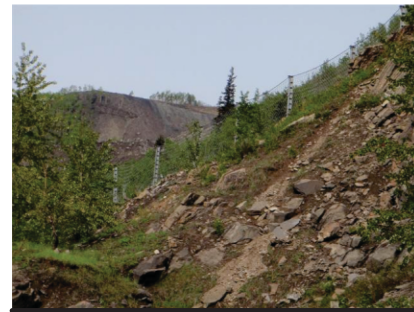
Photo 2c Close up of rock trap fence
