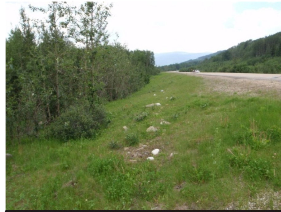
Photo 5 Looking south along sideslope (towards Grande Cache direction) - 1.5m high sidehill embankment fill along verge of Smoky River Valley slope
