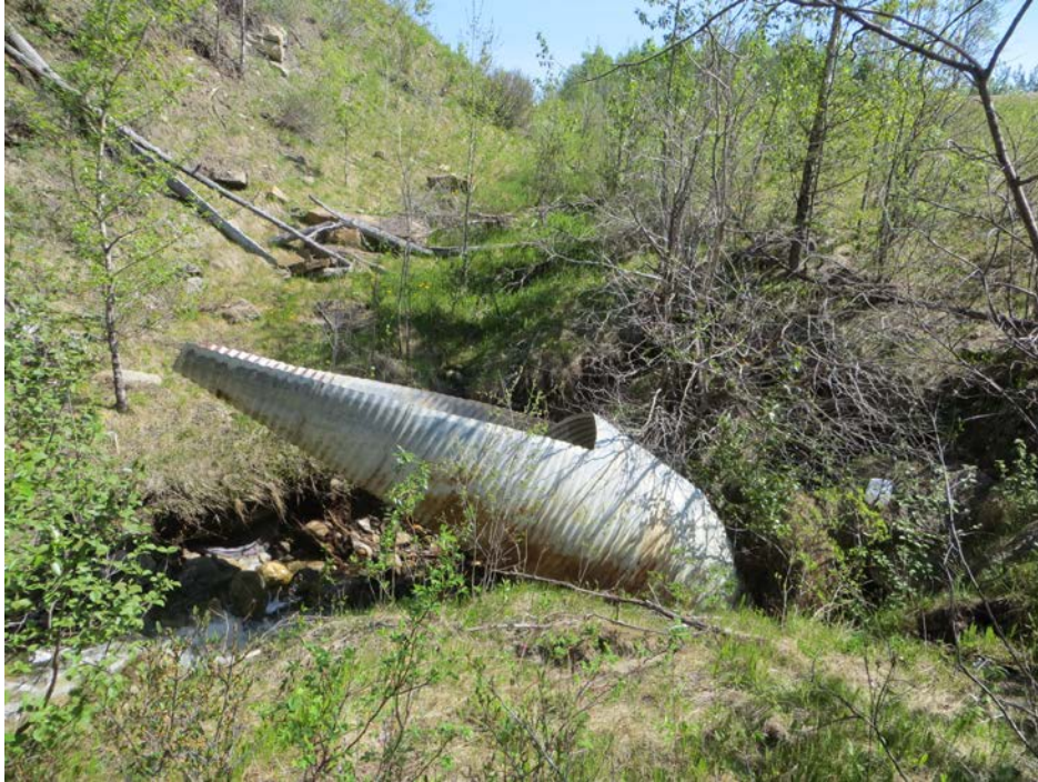
Photo 3 – Looking northeast at the culvert inlet and northwest highway runoff ditch.
