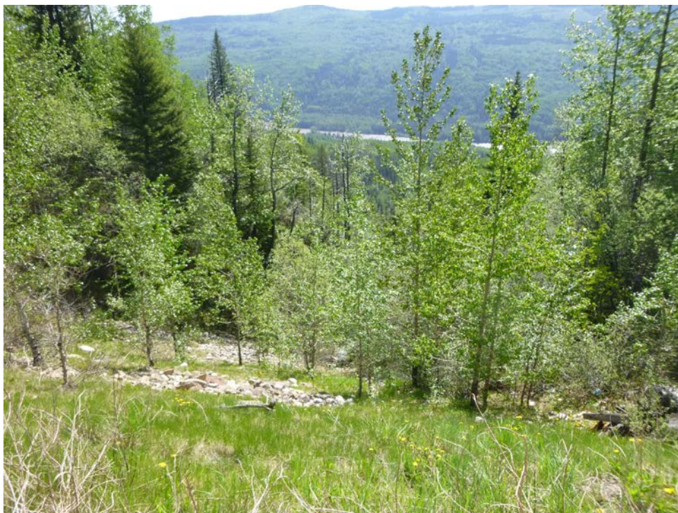
Photo 6 – Looking east at the downstream highway embankment towards the culvert outlet.
