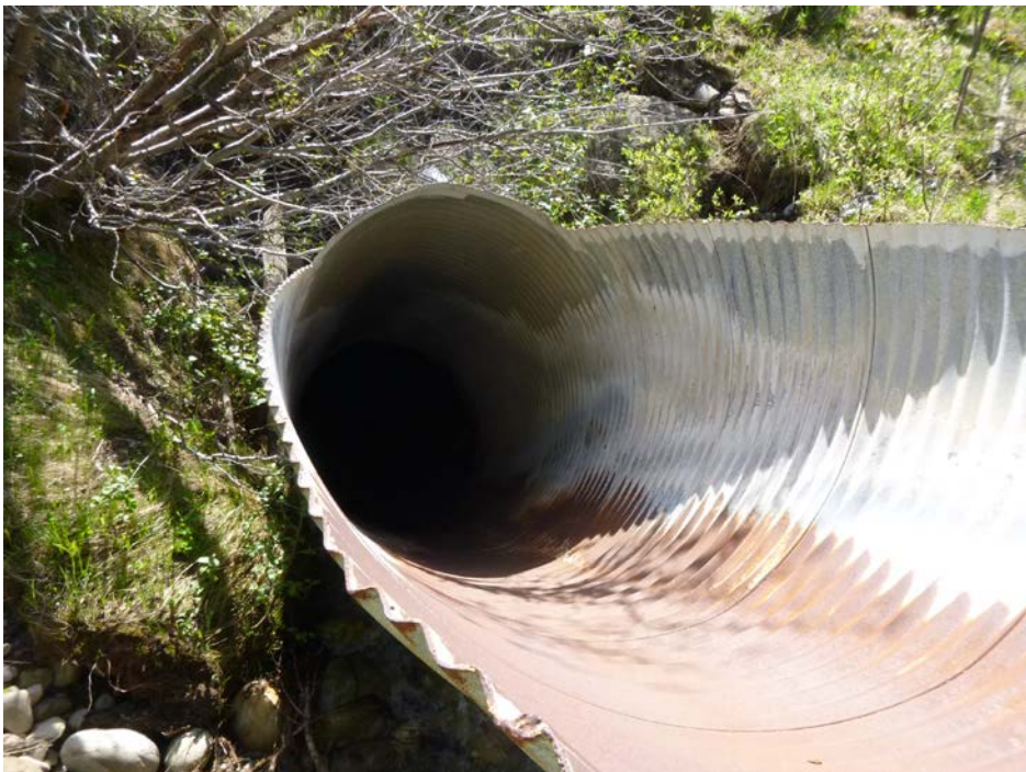
Photo 4 – Close-up view looking down at the culvert inlet.
