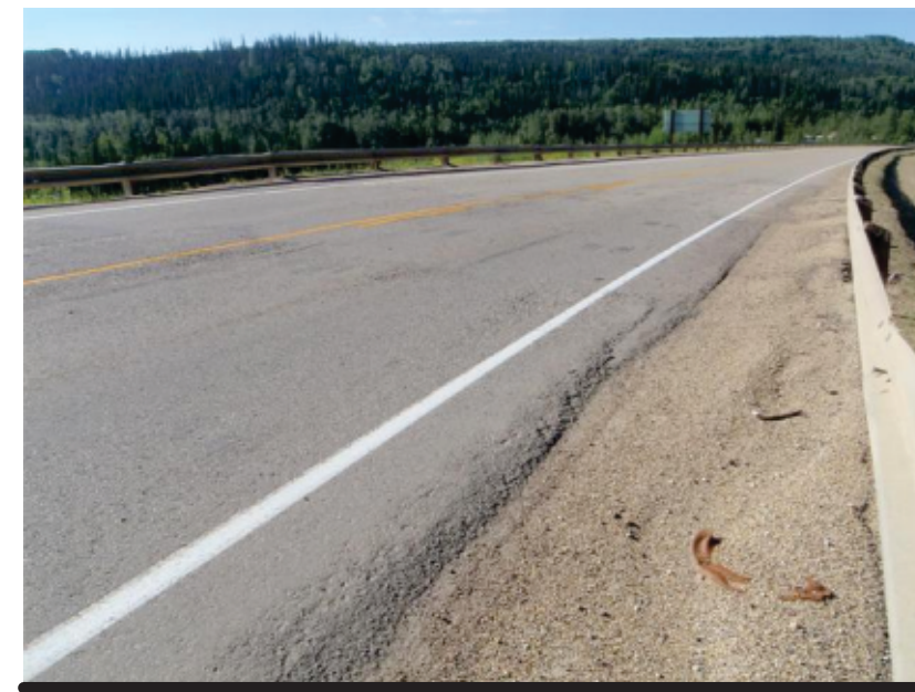
Photo 1e Patched area of headscarp crack (Looking south towards Cutbank River and bridge) • at downgrade side
