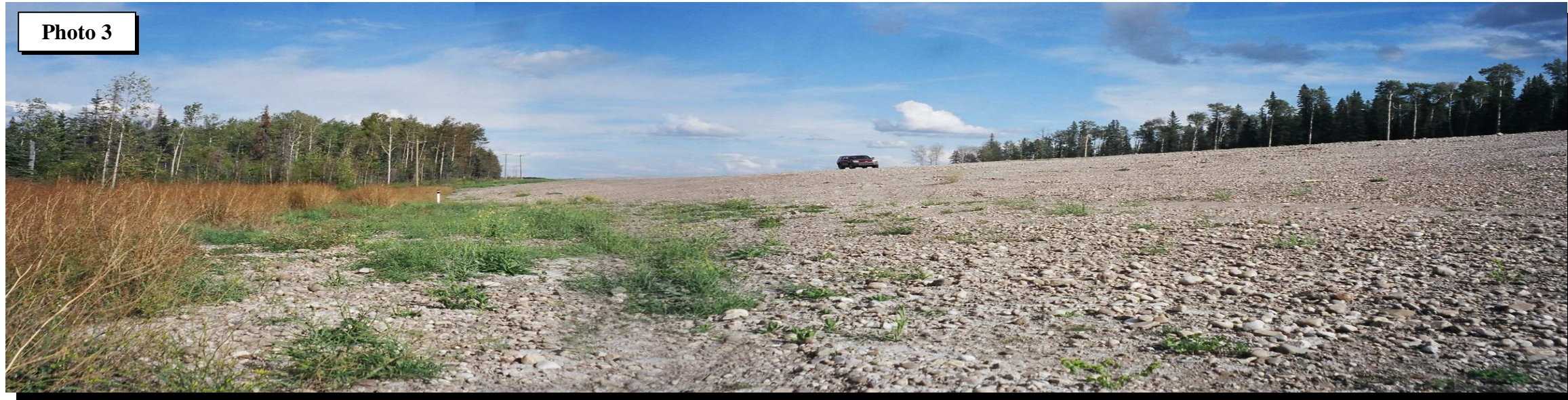
Looking east along toe of reconstructed slope
