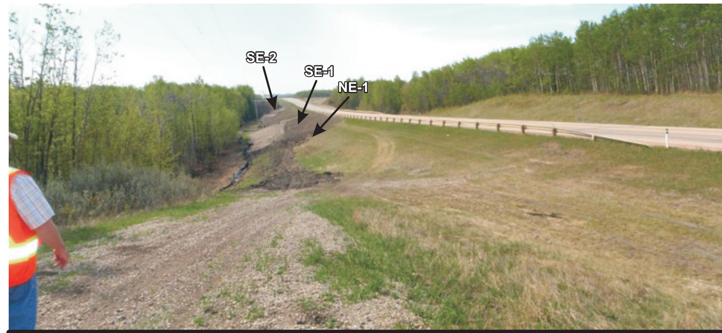
Photo 1 Looking south along east (downstream) sideslope Repaired Slides NE-1, SE-1 and SE-2. General view along east ditch
