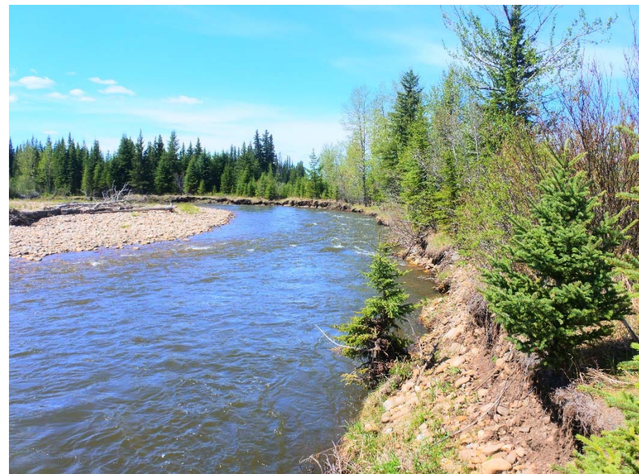
Photo 7. Looking west along the river bank at active toe erosion.
