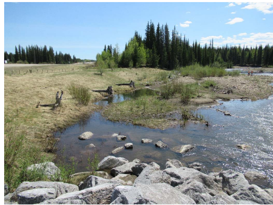
Photo 1. Looking east from the Class 3+ rock riprap spur at the root wads protruding from the embankment.
