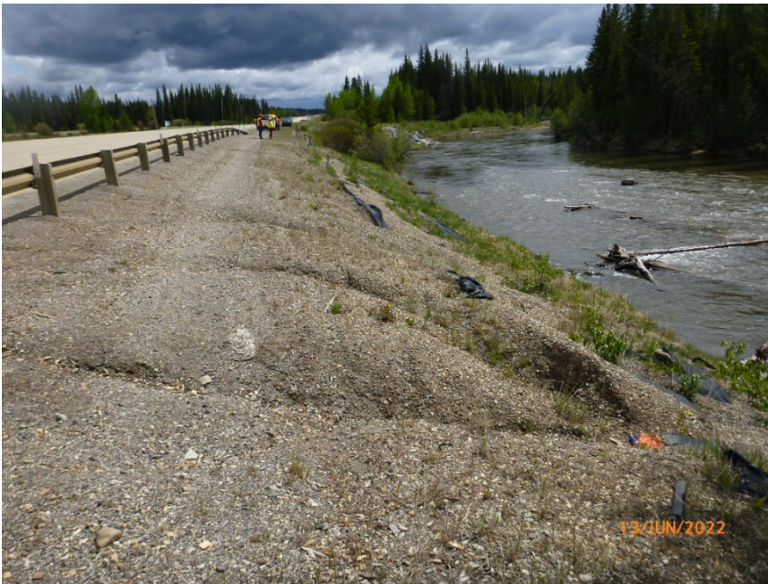
Photo 4 Erosion along north bank of Lone Teepee Creek along south toe of Hwy 40:32 embankment. Note conglomerate riprap particles and exposed geotextile. Photo taken June 13, 2022, facing west.
