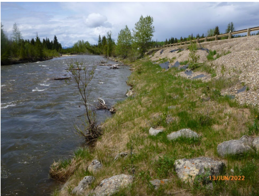
Photo 4 Erosion along north bank of Lone Teepee Creek along south toe of Hwy 40:32 embankment. Note conglomerate riprap particles and exposed geotextile. Photo taken June 13, 2022, facing west.
