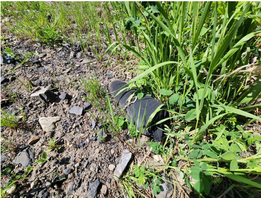
Photo 6 Outlet of drainpipes along toe berm crest installed in 2024 to convey flow from within the slide zone. Photo taken June 2, 2025.
