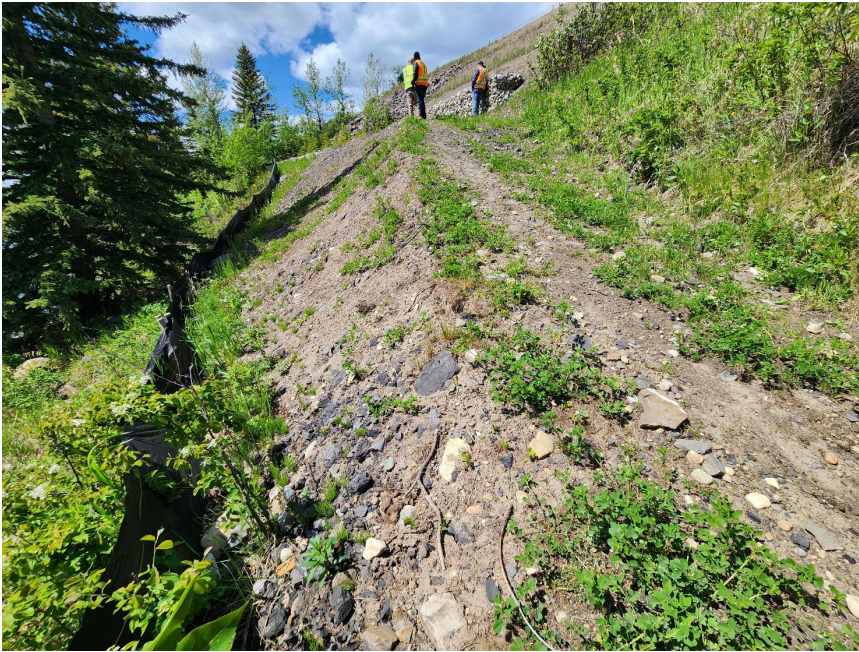
Photo 6 Outlet of drainpipes along toe berm crest installed in 2024 to convey flow from within the slide zone. Photo taken June 2, 2025.
