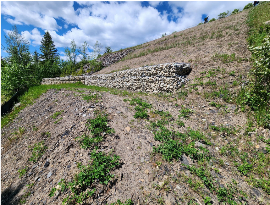
Photo 4 Repaired slide and erosion on south side of Hwy 40:34. Note extension of existing gabion baskets and toe berm from previously repaired section. Photo taken June 2, 2025, facing northwest.
