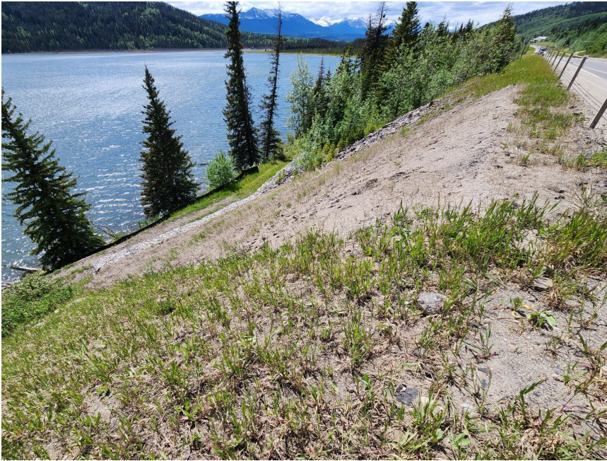
Photo 4 Repaired slide and erosion on south side of Hwy 40:34. Note extension of existing gabion baskets and toe berm from previously repaired section. Photo taken June 2, 2025, facing northwest.
