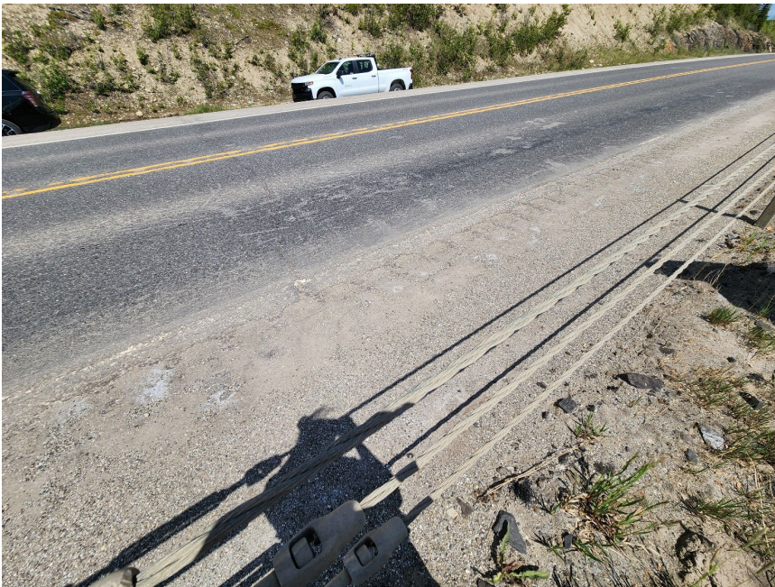
Photo 2 Distress in pavement surface of Hwy 40:34 above repair completed in 2024. Photo taken June 2, 2025, facing northeast.
