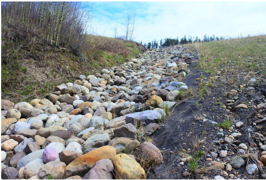
Photo 23. Looking southeast at the east crotch ditch.
