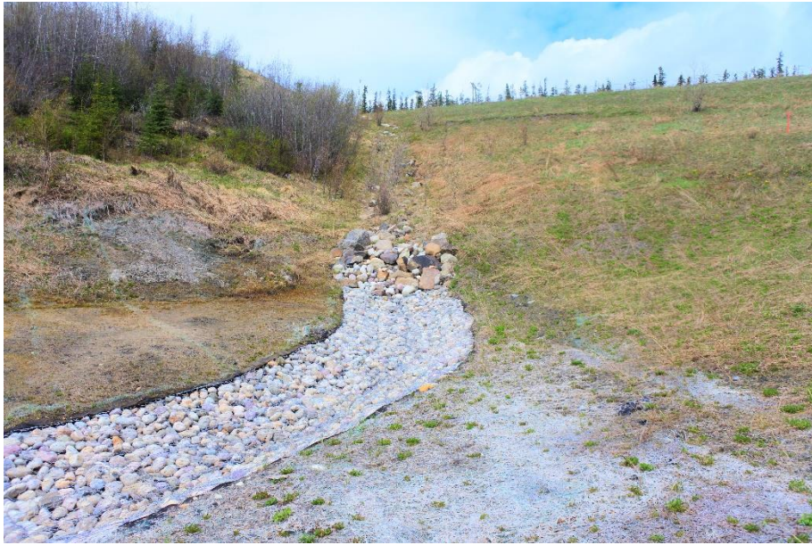
Photo 19. Looking northwest at west crotch ditch.
