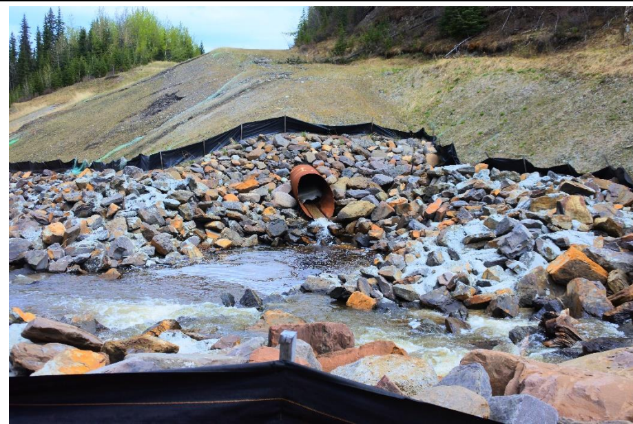
Photo 11. Looking at outlet of 1200 mm diam. SWSP culvert into dissipation bowl.
