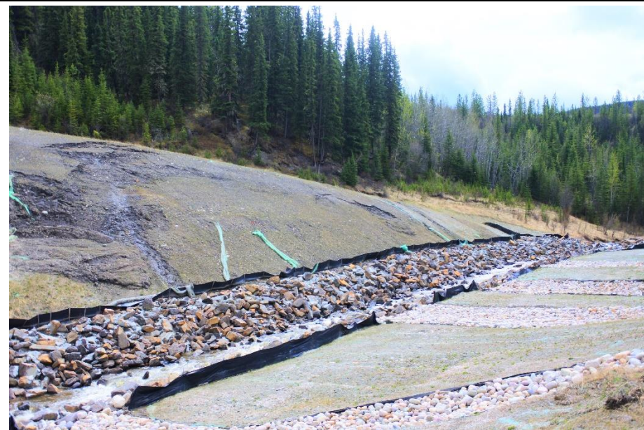
Photo 14. Looking southeast at the main channel.
