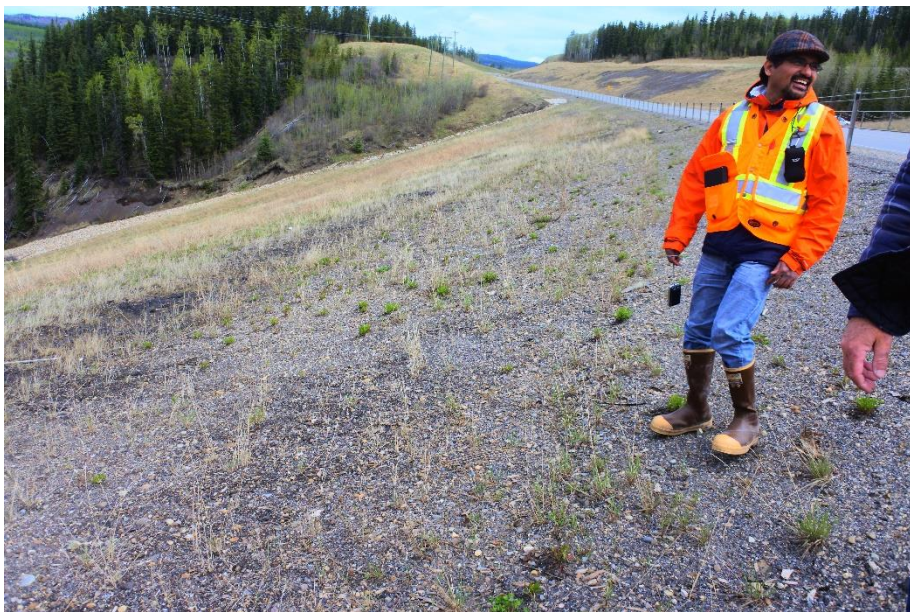
Photo 20. Looking northeast at slope north of the highway. Some grass is growing from broadcast seeding.
