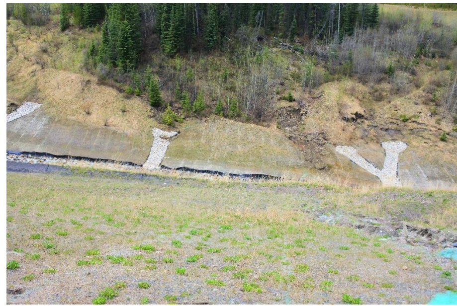
Photo 8. Looking west towards slope on west side of main channel.
