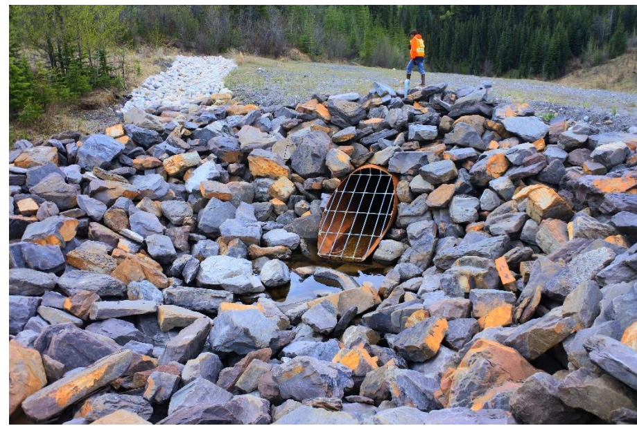
Photo 3. Looking southwest at 1200 mm Diam. SWSP inlet and surrounding rip rap.
