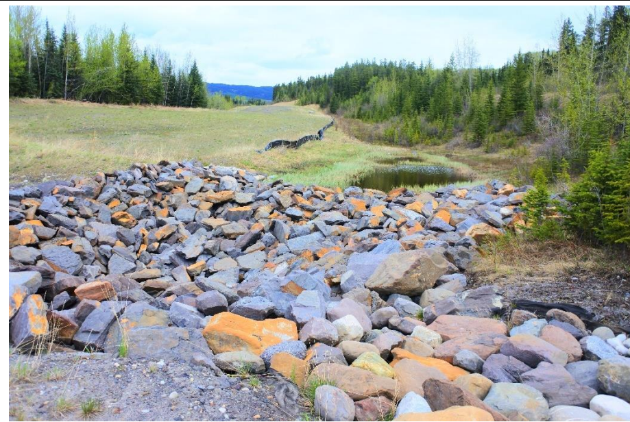
Photo 2. Looking east at the pond area above the culvert inlet.
