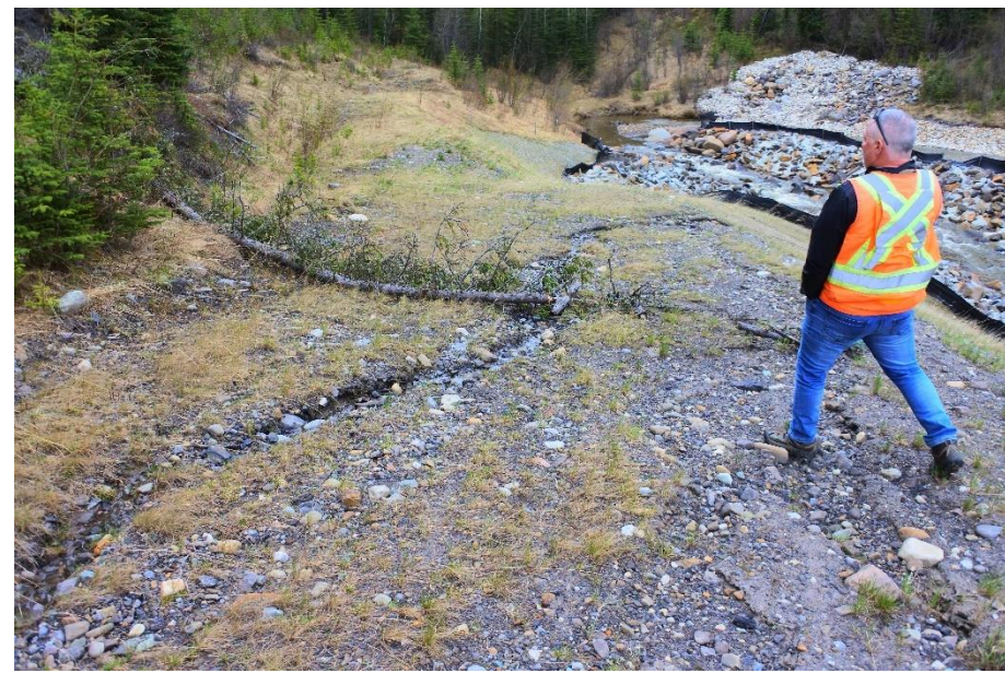
Photo 9. Looking southwest at the buried SWSP culvert path.
