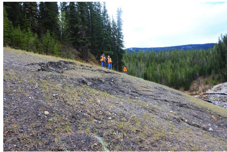
Photo 7. Looking south at slumped area. Note ground seepage.
