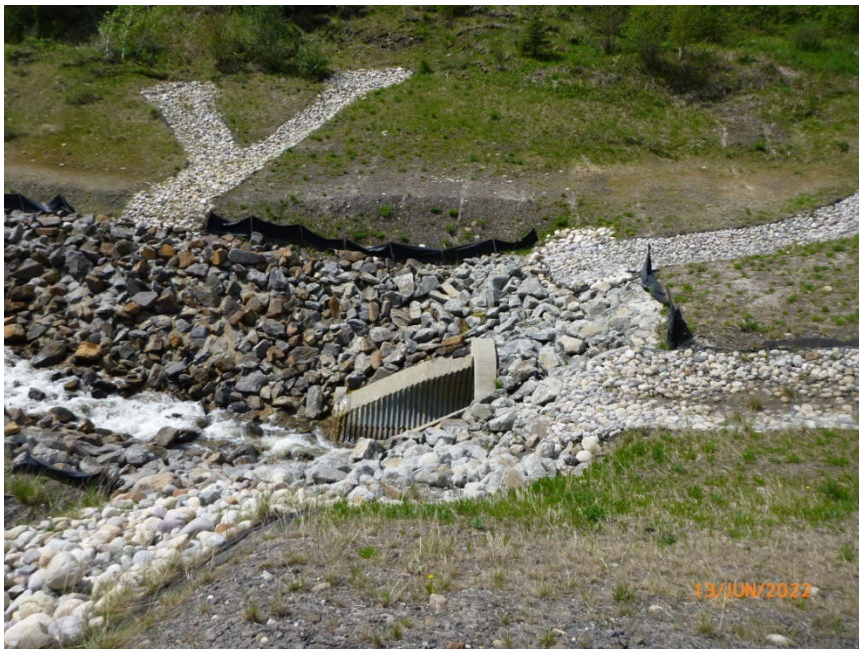
Photo 5 Inlet of 3000-mm diameter CSP culvert at upstream/south toe of Hwy 40:34 embankment. Photo taken June 13, 2022, facing west.
