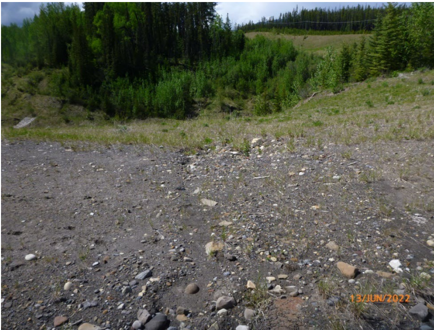
Photo 15 Erosion between catch basin and crest of east valley slope indicates catch basin may have previously overflowed. Photo taken June 13, 2022, facing west.
