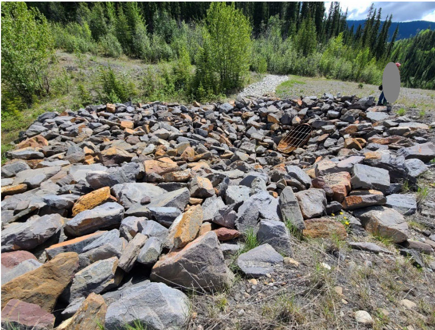
Photo 13 Riprap-lined catch basin and buried slope drain inlet. Photo taken June 13, 2022, facing south.
