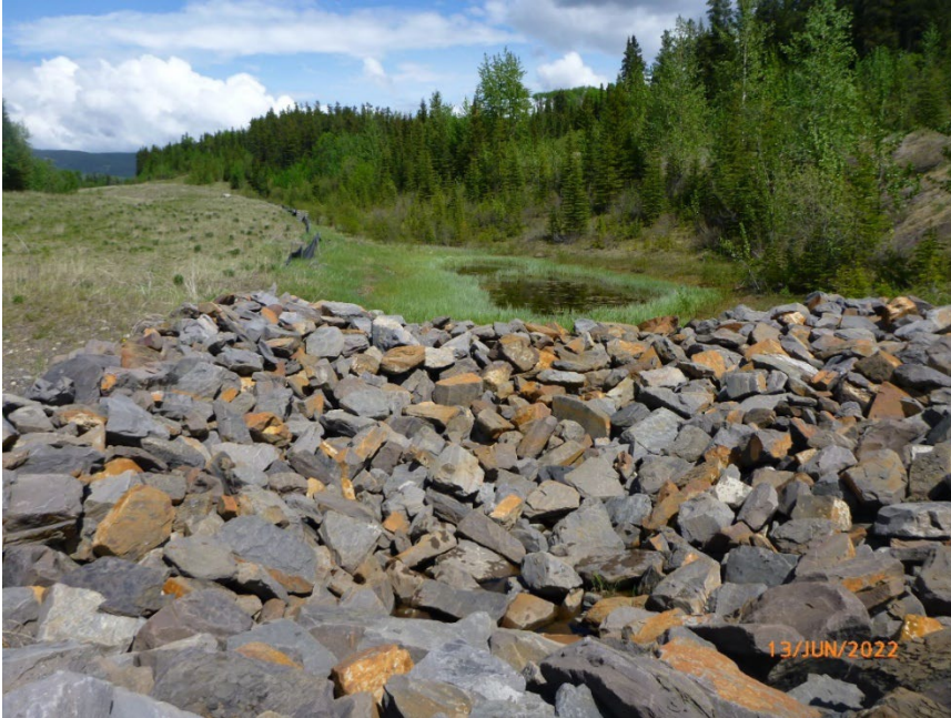
Photo 15 Erosion between catch basin and crest of east valley slope indicates catch basin may have previously overflowed. Photo taken June 13, 2022, facing west.
