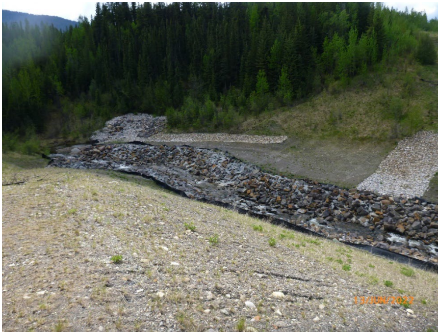
Photo 7 Upstream/south extent of riprap-lined channel. Note rill erosion on east valley slope. Photo taken June 13, 2022, facing southwest.
