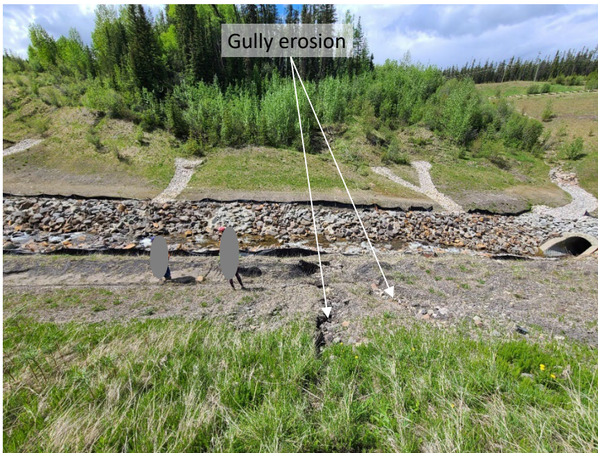
Photo 9 Erosion gullies on east valley slope at WP184. Photo taken June 13, 2022, facing west.
