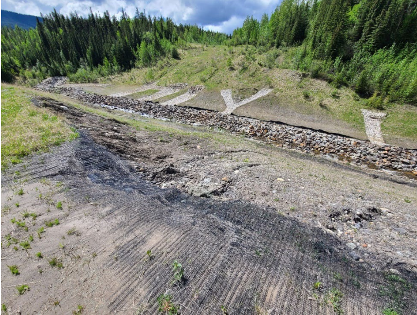
Photo 13 Riprap-lined catch basin and buried slope drain inlet. Photo taken June 13, 2022, facing south.
