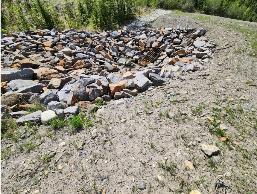
Photo 16 Buried slope drain outlet at toe of east valley slope, near south end of site. Photo taken June 2, 2025.
