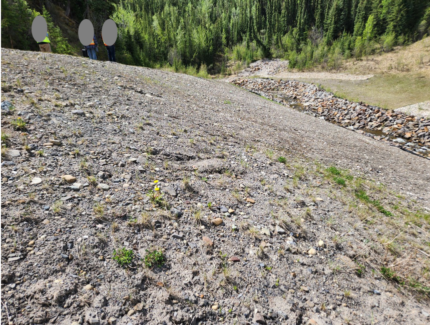
Photo 12 South slide area on east valley slope repaired in 2024. Note erosion down center and drainpipe outlets (circled in black). Photo taken June 2, 2025, facing east.
