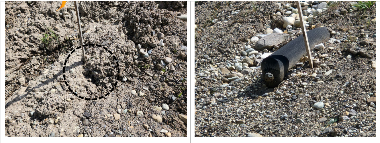
Photo 8 Drainpipe outlets in middle slide area. Photos taken June 2, 2025.
