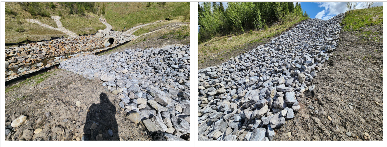
Photo 4 Riprap-lined trapezoidal channel constructed in 2024 on east valley slope. Photo taken June 2, 2025, facing northwest and northeast, respectively.
