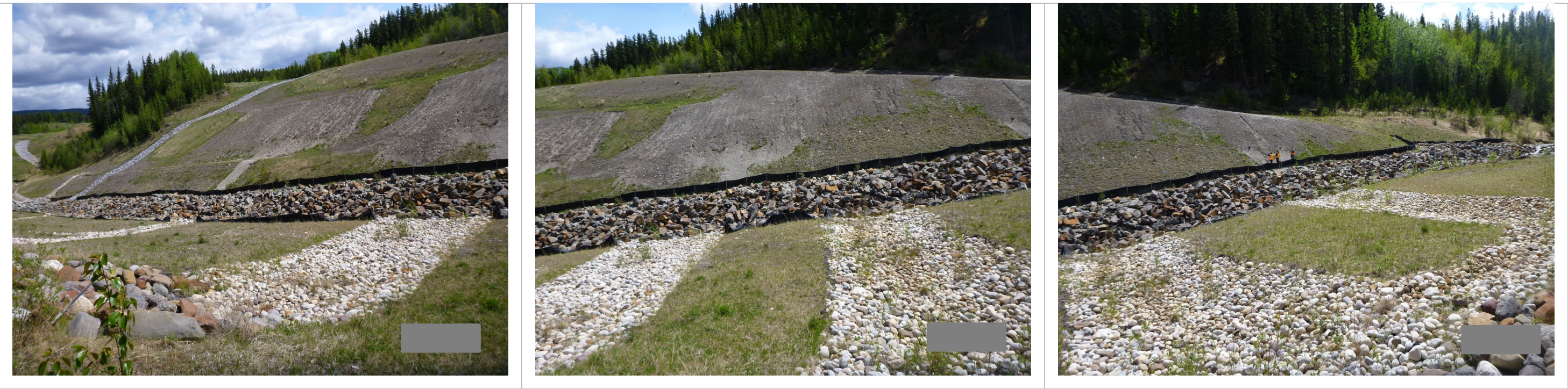
Photo 2 West slope previously repaired in 2017/2018. Note slope failures/slumps above finger drains (indicated with white lines) and inlet of 3-m diameter culvert at south toe of Hwy 40:34 embankment. Photos taken June 2, 2025, facing southwest, west, and northwest, respectively.
