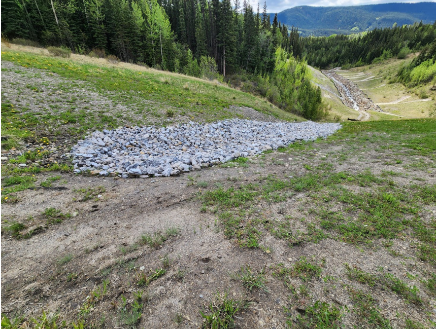
Photo 14 Riprap-lined cross ditch along east abutment of highway embankment, at north end of site. Note portion of ditch is not lined with riprap. Photo taken June 2, 2025, facing northeast.
