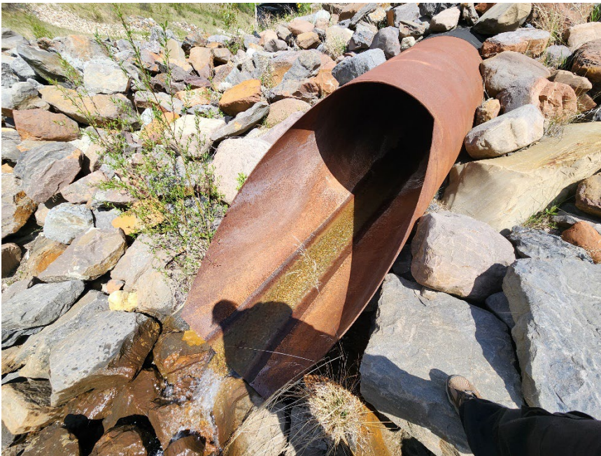
Photo 16 Buried slope drain outlet at toe of east valley slope, near south end of site. Photo taken June 2, 2025.
