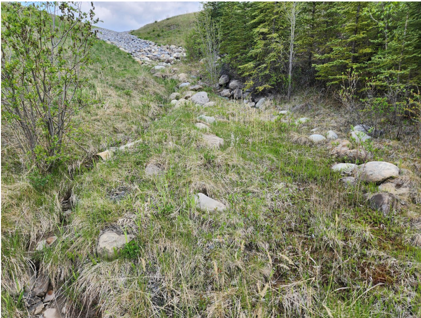
Photo 14 Riprap-lined cross ditch along east abutment of highway embankment, at north end of site. Note portion of ditch is not lined with riprap. Photo taken June 2, 2025, facing northeast.
