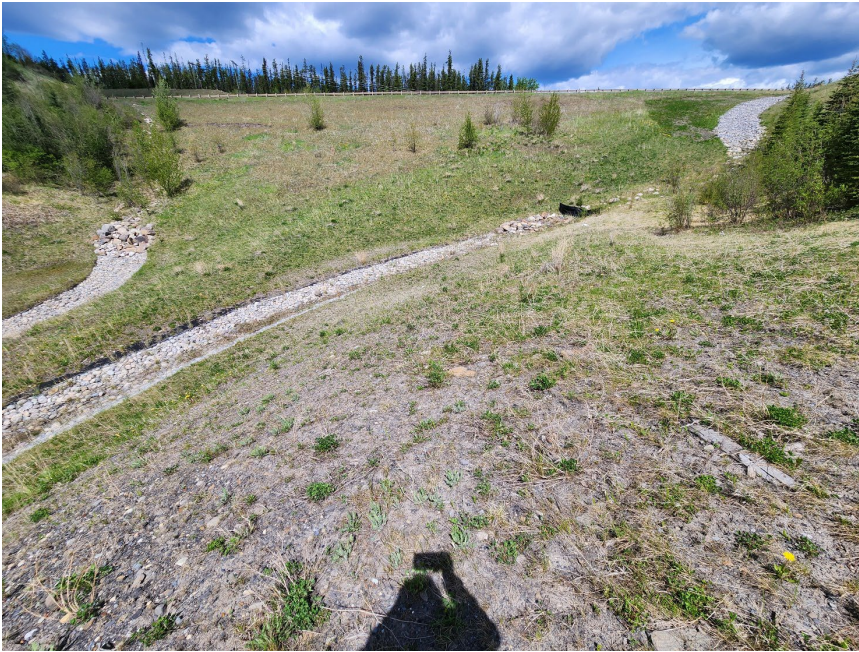
Photo 4 Riprap-lined trapezoidal channel constructed in 2024 on east valley slope. Photo taken June 2, 2025, facing northwest and northeast, respectively.
