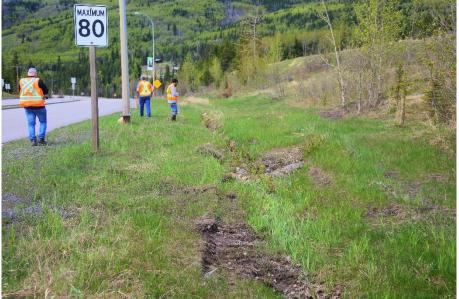
Photo 10. Looking north from the beginning of the erosion gully in the grassed ditch (near the south end).
