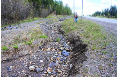
Photo 2. Looking south at further eroded gully in ditch.
