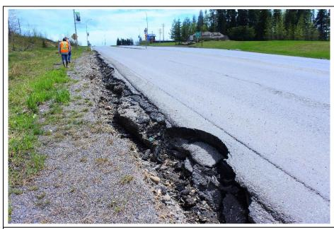
Photo 11. Looking south at new erosion that runs near highway pavement.
