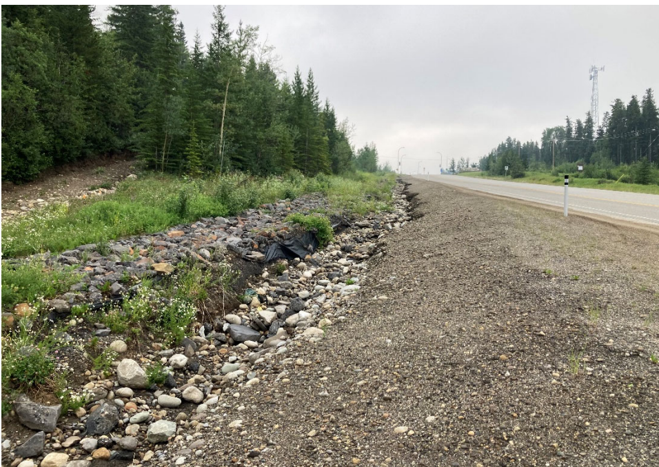
Photo 2 Exposed geotextile from a previous repair, on the east edge of the ditch erosion. Photo taken July 21, 2021 facing south.
