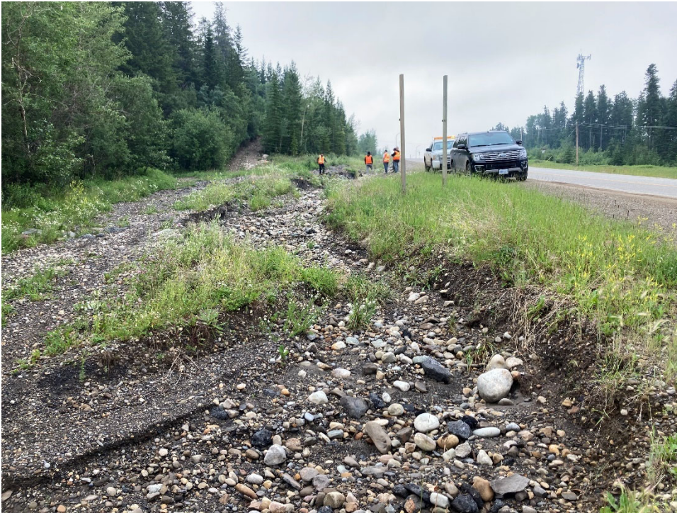
Photo 2 Exposed geotextile from a previous repair, on the east edge of the ditch erosion. Photo taken July 21, 2021 facing south.
