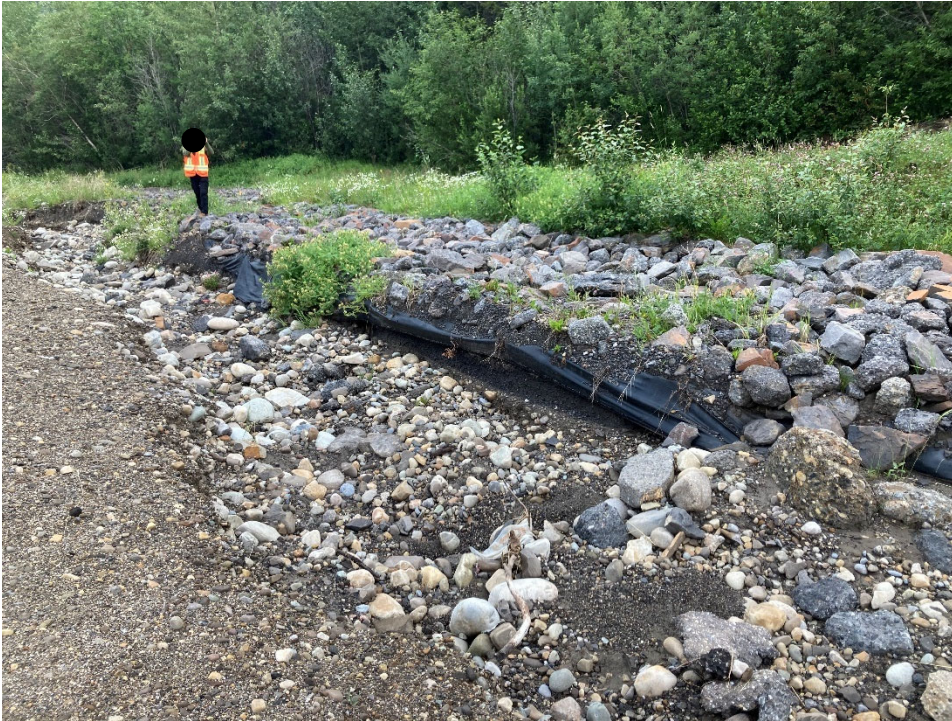
Photo 4 The ditch erosion has retrogressed to the east edge (southbound lane) of Hwy 40 and is beginning to impact the shoulder of the highway. Photo taken July 21, 2021 facing south.
