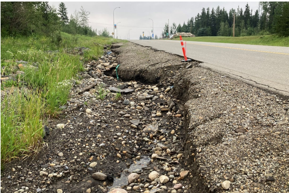
Photo 4 The ditch erosion has retrogressed to the east edge (southbound lane) of Hwy 40 and is beginning to impact the shoulder of the highway. Photo taken July 21, 2021 facing south.
