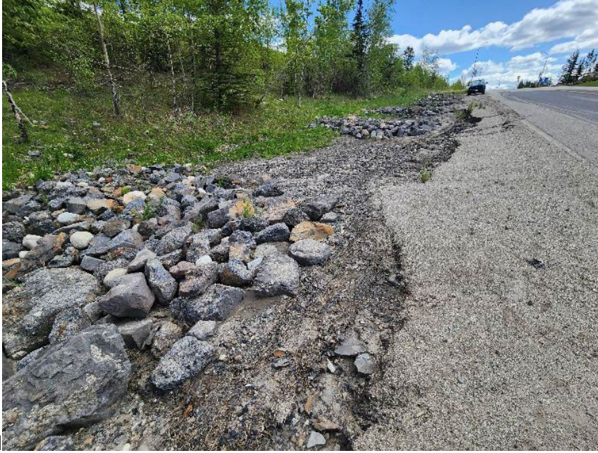
Photo 2 Ditch on east side of Hwy 40:34. Note erosion between highway shoulder and ditch from flow bypassing check dams. Photo taken June 2, 2025, facing northwest.
