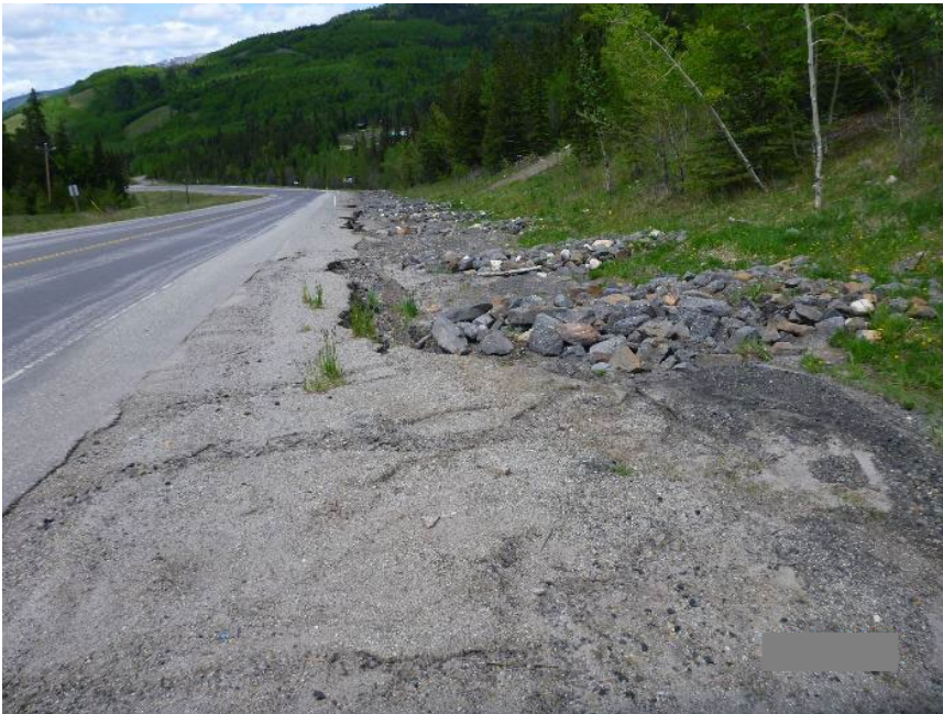
Photo 2 Ditch on east side of Hwy 40:34. Note erosion between highway shoulder and ditch from flow bypassing check dams. Photo taken June 2, 2025, facing northwest.
