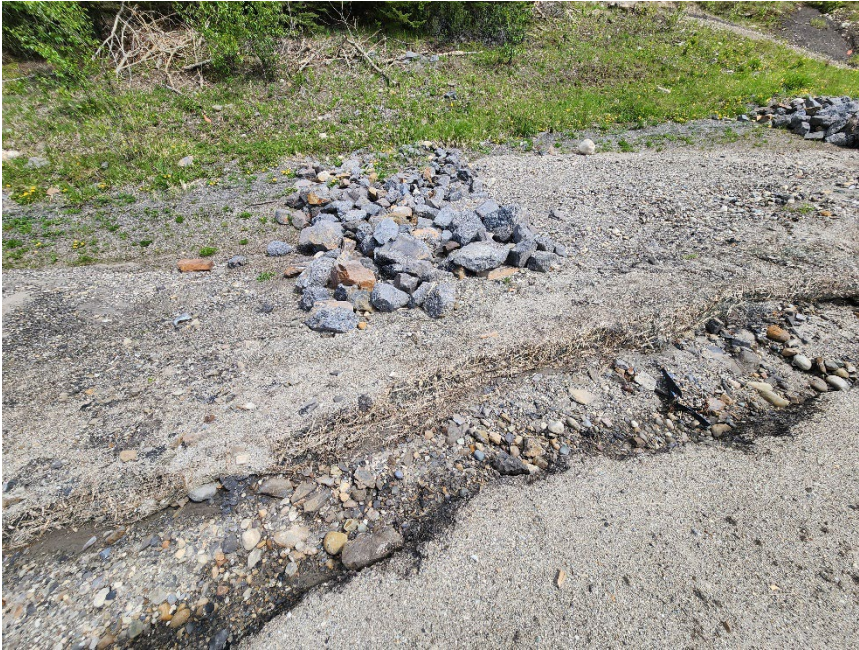
Photo 6 Ditch on east side of Hwy 40:34. Note erosion between highway shoulder and ditch from flow bypassing check dams, deterioration and undermining of turf reinforcement mat, and quality of riprap particles in ditch, some of which are composed of conglomerate. Photo taken June 2, 2025, facing southeast.
