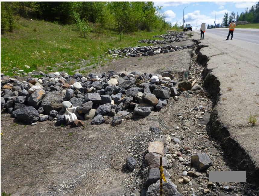
Photo 6 Ditch on east side of Hwy 40:34. Note erosion between highway shoulder and ditch from flow bypassing check dams, deterioration and undermining of turf reinforcement mat, and quality of riprap particles in ditch, some of which are composed of conglomerate. Photo taken June 2, 2025, facing southeast.
