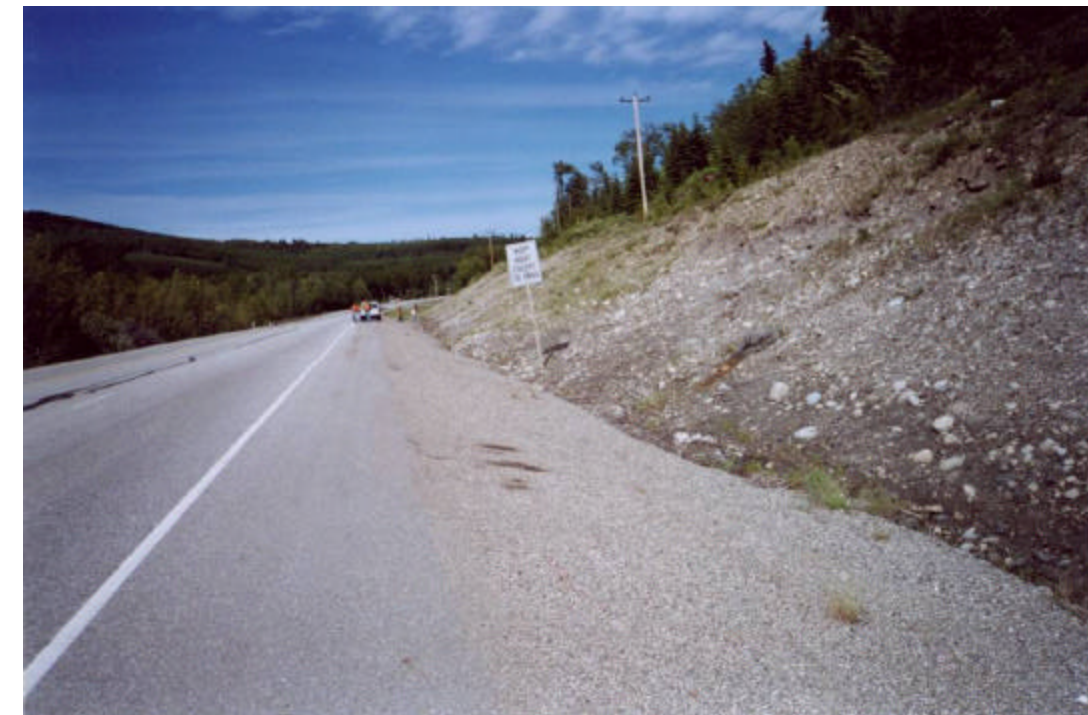
Photo 4 Close up - Looking upgrade (towards Grande Cache)
