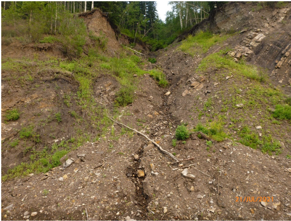
Photo 6 Erosion gully located at the south end of the GP036 site at debris flow location (WP 106). Photo taken July 21, 2021 facing west.
