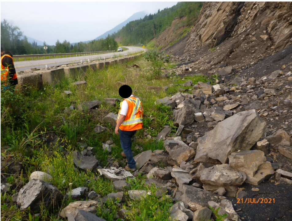
Photo 3 Rockfall debris observed in the west (southbound) ditch at WP105. Photo taken July 21, 2021 facing southwest.
