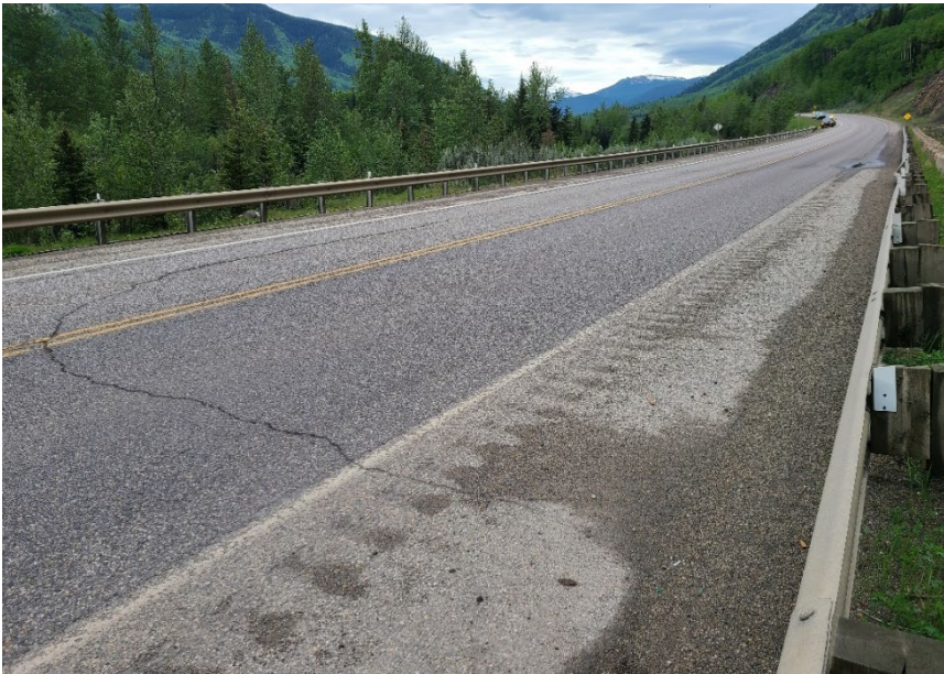
Photo 8 Some rockfall particles on east side of Hwy 40:36 between guardrail and railway tracks. These particles may have been cleaned off highway, but AT has reported rockfall particles making it across highway. Photo taken June 14, 2022, facing northeast.
