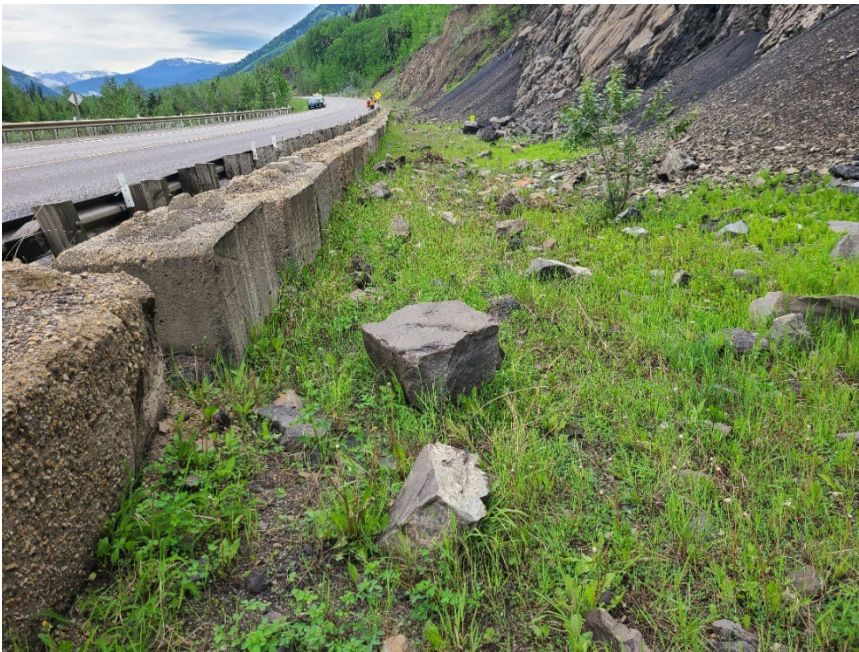
Photo 4 Talus (coal) deposits and rockfall particles in upslope/west ditch of Hwy 40:36. Note lock blocks are deteriorating. Photo taken June 14, 2022, facing southwest.
