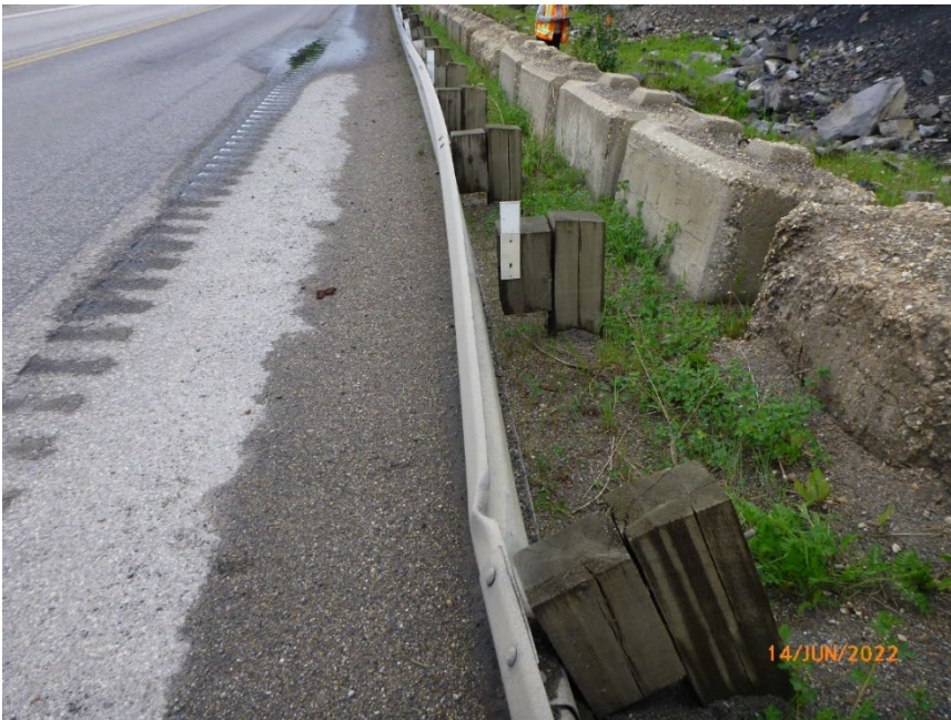
Photo 6 Segment of guardrail deflected and pushed towards southbound traffic from rockfall strike. Photo taken June 14, 2022, facing southwest.
