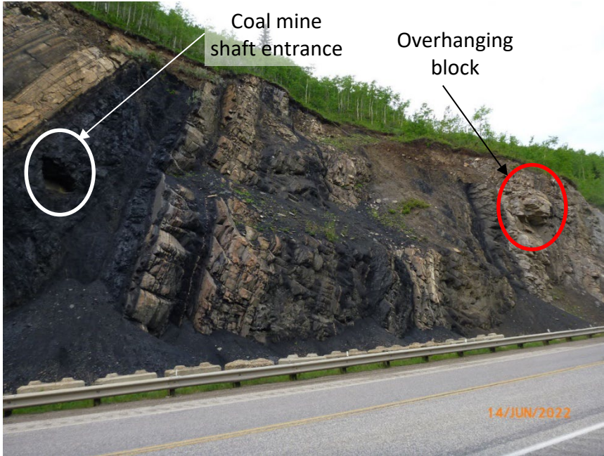
Photo 4 Talus (coal) deposits and rockfall particles in upslope/west ditch of Hwy 40:36. Note lock blocks are deteriorating. Photo taken June 14, 2022, facing southwest.
