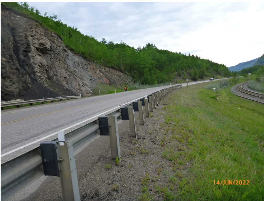
Photo 8 Some rockfall particles on east side of Hwy 40:36 between guardrail and railway tracks. These particles may have been cleaned off highway, but AT has reported rockfall particles making it across highway. Photo taken June 14, 2022, facing northeast.
