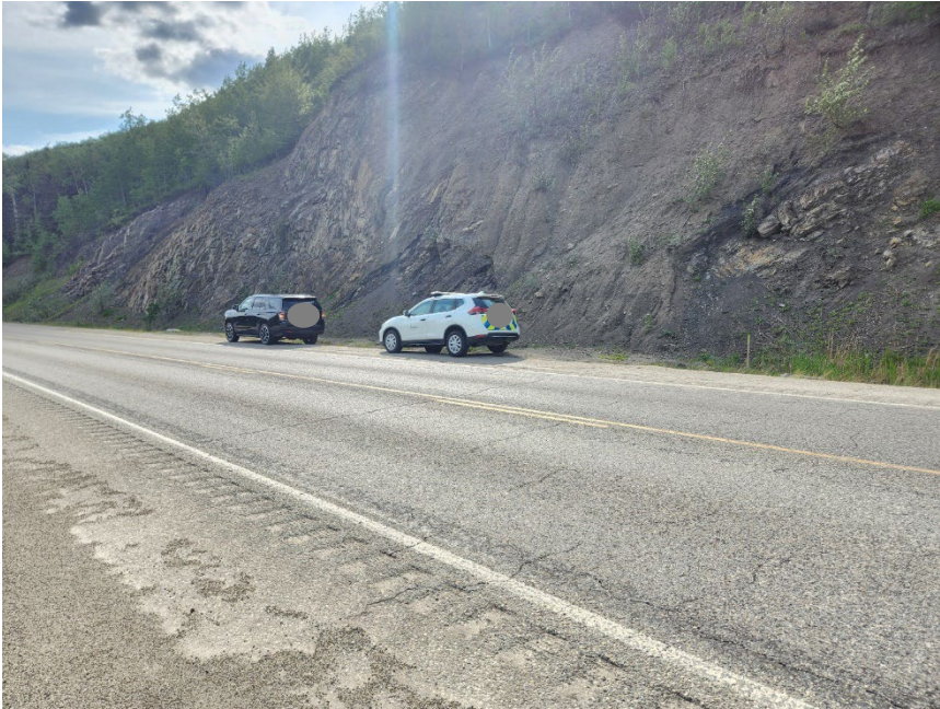
Photo 2 Rock slope along west side of Hwy 40:36, north of GP054 debris flow site. Note GP054 km 12.1 debris flow site on left. Photo taken June 2, 2025, facing northeast.
