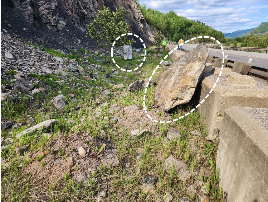
Photo 8 Rockfall particles in ditch on west side of Hwy 40:36. Additional particles appears to have fallen since 2024 inspection. Photo taken June 2, 2025, facing southwest.
