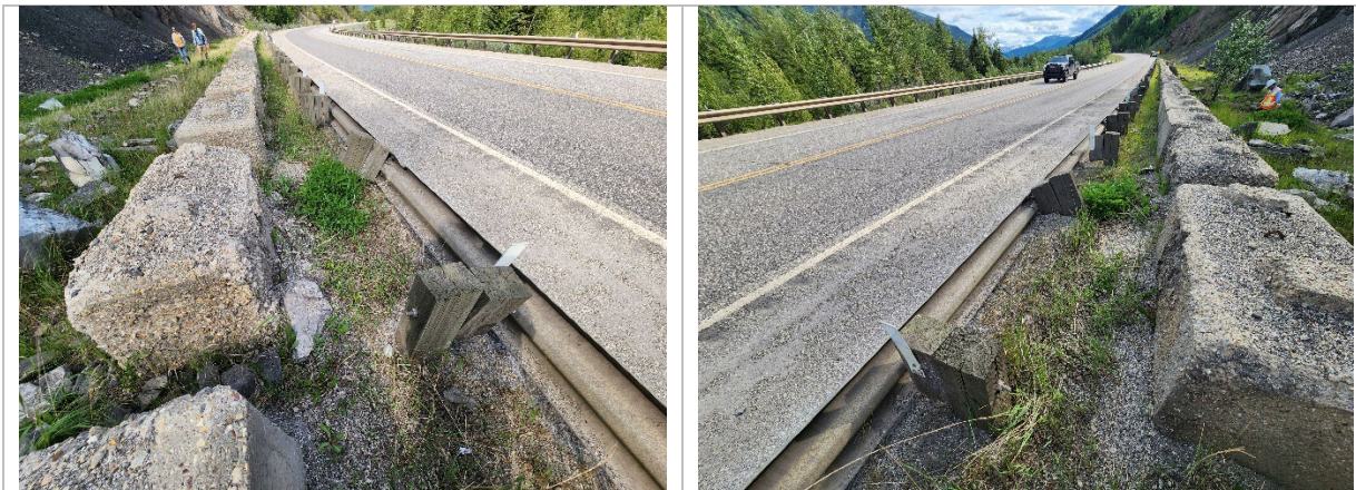
Photo 12 Pavement surface of Hwy 40:36. Note lock blocks are deteriorating and segment of guardrail deflected and pushed towards southbound lane from rock strikes. Photos taken June 2, 2025, facing northeast and southwest, respectively.
