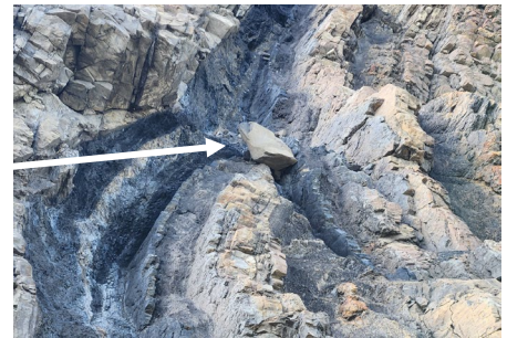
Photo 5 Rock slope along west side of Hwy 40:36. Note loose rock block (circled in white) on slope. Photo taken June 2, 2025, facing northwest.
