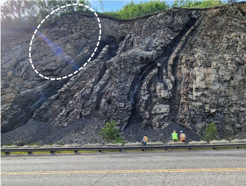
Photo 4 Potential rock block on upper slope shown in previous photo. Note dilated or open joints below rock block (indicated with white arrow), joints or shear planes to left and below rock block (circled in white), and rock and coal to right of rock block which is eroding. Photo taken June 2, 2025, facing northwest.
