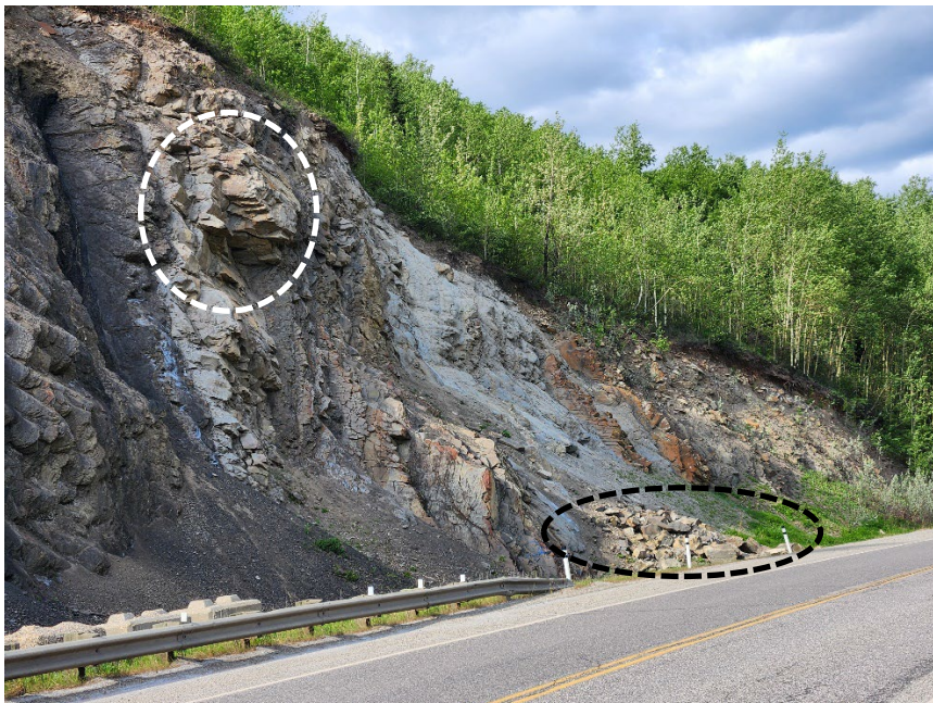
Photo 10 Rock slope along west side of Hwy 40:36 near north end of site. Note hanging rock block (circled in white) and rockfall that occurred between 2023 and 2024 inspections (circled in black). Additional material appears to have fallen since 2024 inspection. Photo taken June 2, 2025, facing north.
