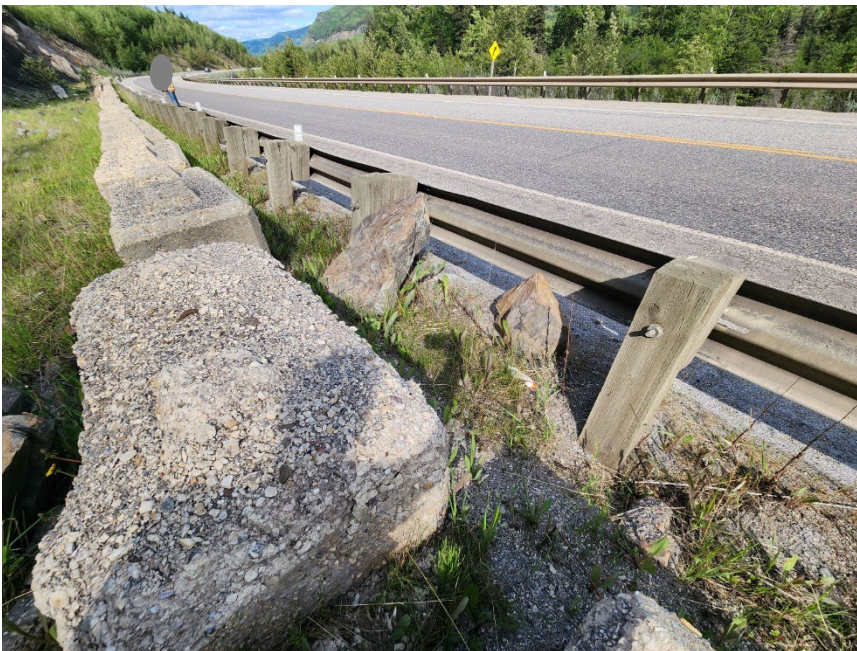
Photo 6 Rockfall particle leaning against guardrail along west shoulder of Hwy 40:36. Photo taken June 2, 2025, facing northeast.
