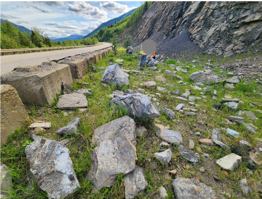
Photo 8 Rockfall particles in ditch on west side of Hwy 40:36. Additional particles appears to have fallen since 2024 inspection. Photo taken June 2, 2025, facing southwest.
