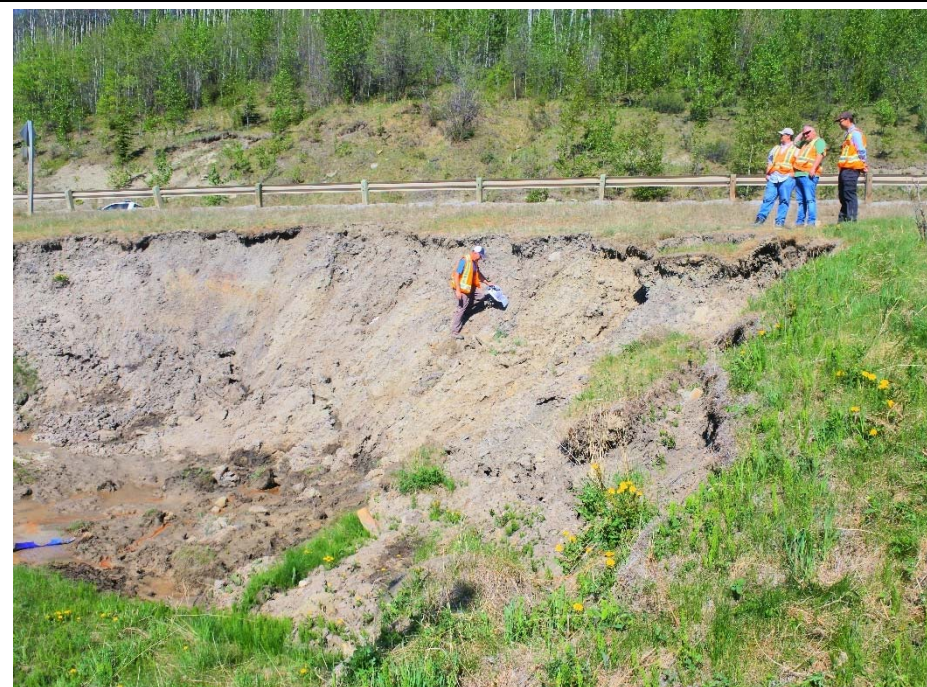
Photo 6. Looking northwest at the main scarp.
