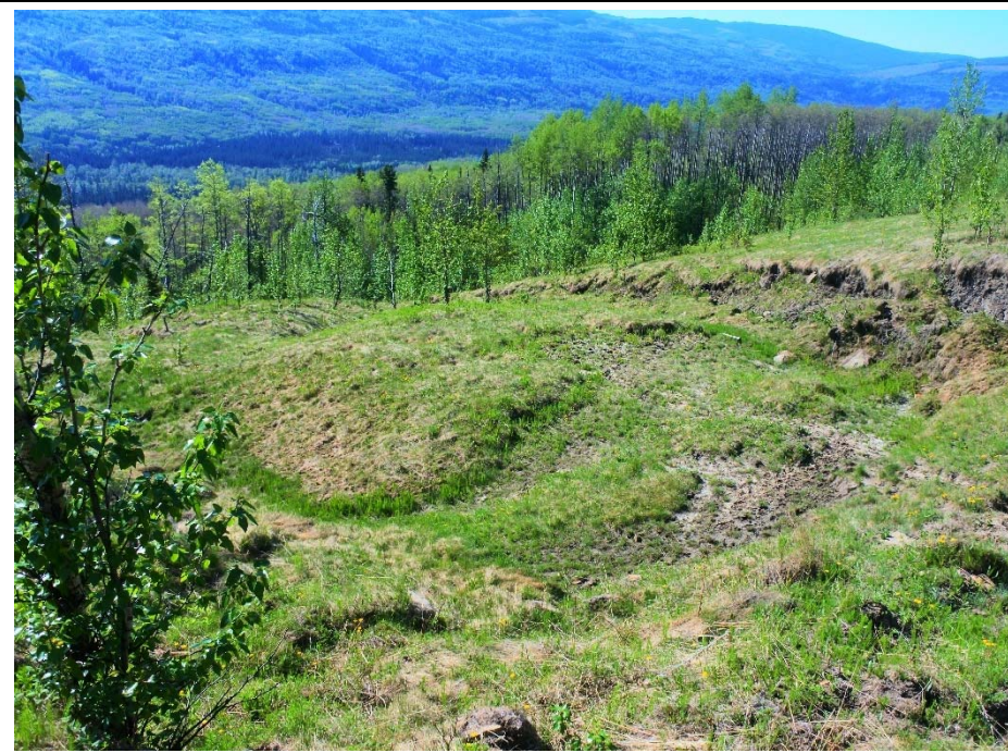
Photo 7. Looking southwest at the intermediate toe area.
