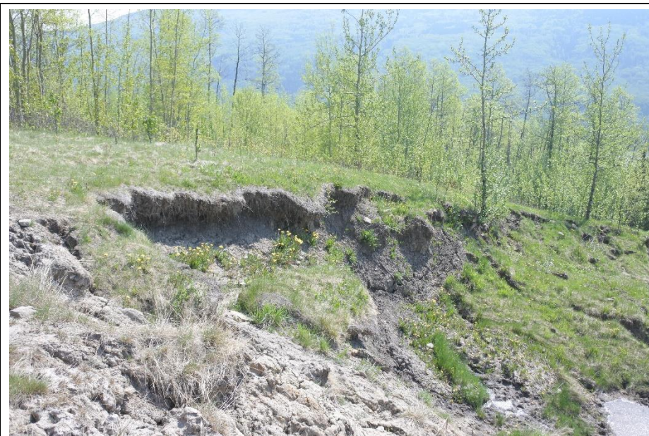
Photo 5. Looking southeast at area observed with fresh sloughing and tears.
