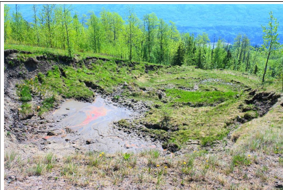
Photo 3. Looking east at the slide from above the main scarp. approached
