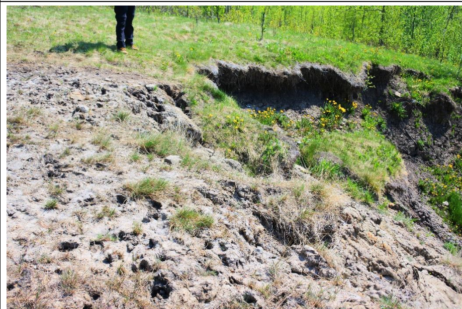
Photo 4. Looking east at recent tears and sloughed material.
