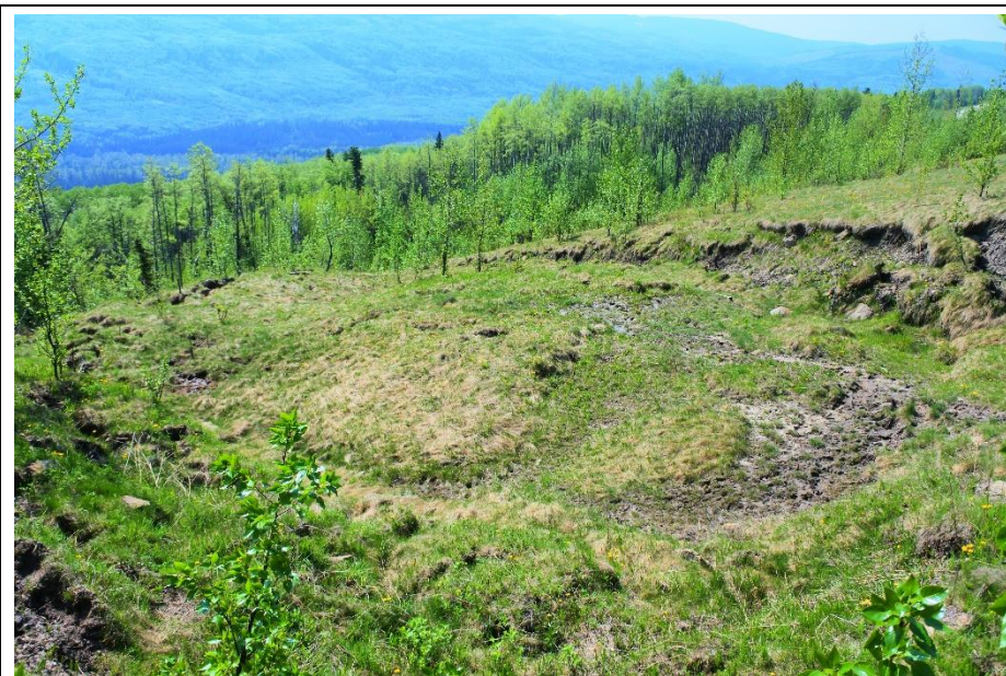
Photo 7. Looking southwest at the intermediate toe area.
