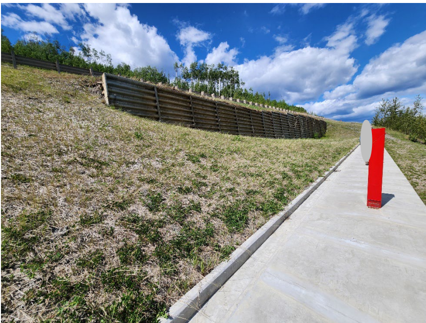
Photo 9 Binwall and middle pile wall on east (downslope) side of Hwy 40:36. Photo taken June 2, 2025, facing north.
