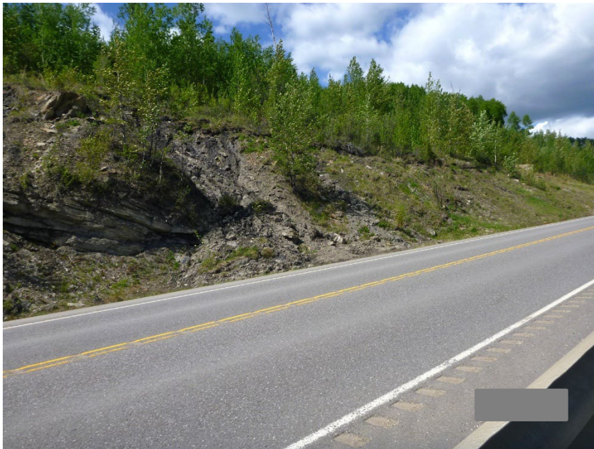
Photo 13 Rock slope along west (upslope) side of Hwy 40:36. Note thin cover of soil over bedrock, which is slumping likely due to saturation. Photo taken June 2, 2025, facing north.
