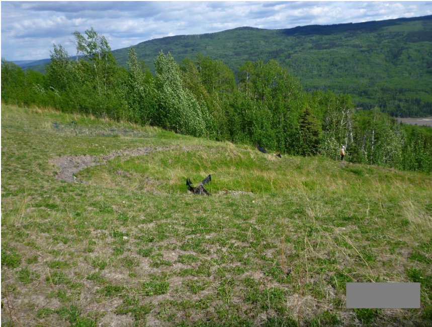
Photo 7 Slide scarp on east (downslope) side of Hwy 40:36. Note slide scarp is unvegetated indicating recent movement. Photo taken June 2, 2025, facing southwest.
