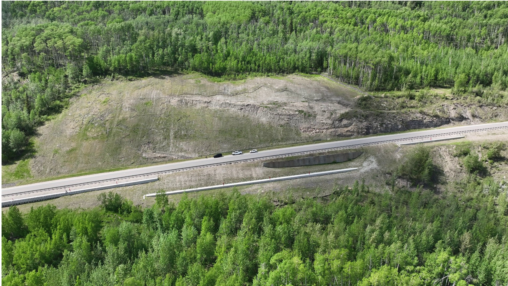
Photo 4 North portion of site. Note binwall and three pile walls on east (downslope) side of Hwy 40:36, and slumping and toe rolls on west (upslope) side of Hwy 40:36. UAV photo taken June 2, 2025, facing northwest.
