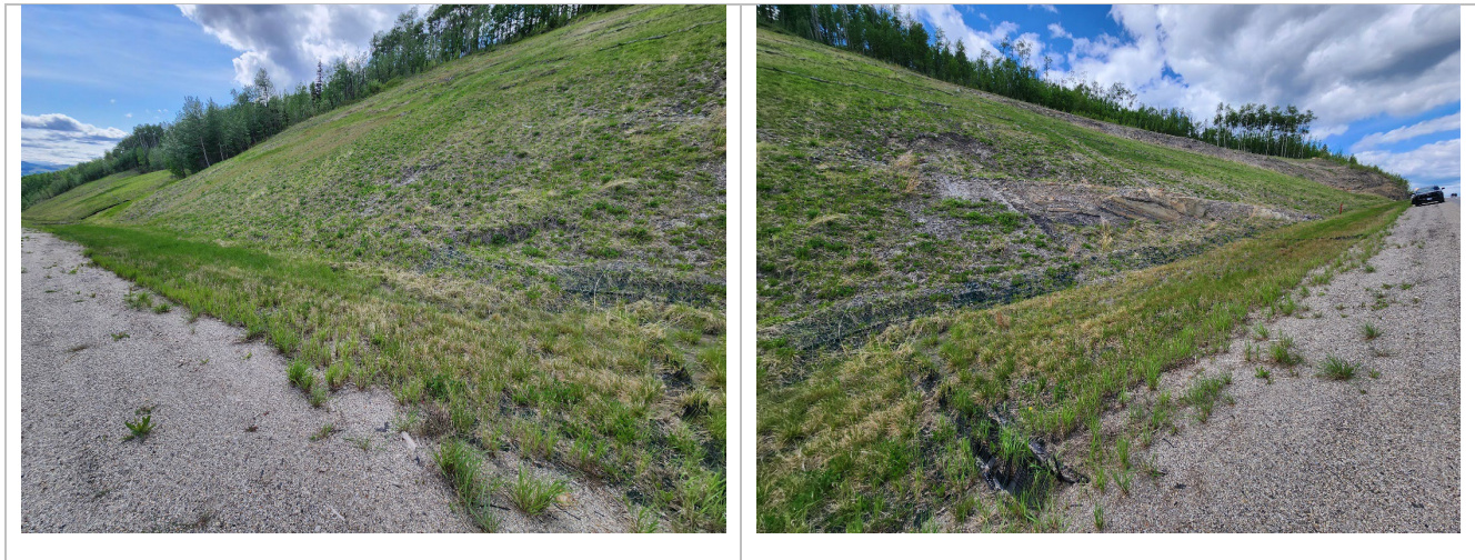
Photo 13 Rock slope along west (upslope) side of Hwy 40:36. Note thin cover of soil over bedrock, which is slumping likely due to saturation. Photo taken June 2, 2025, facing north.
