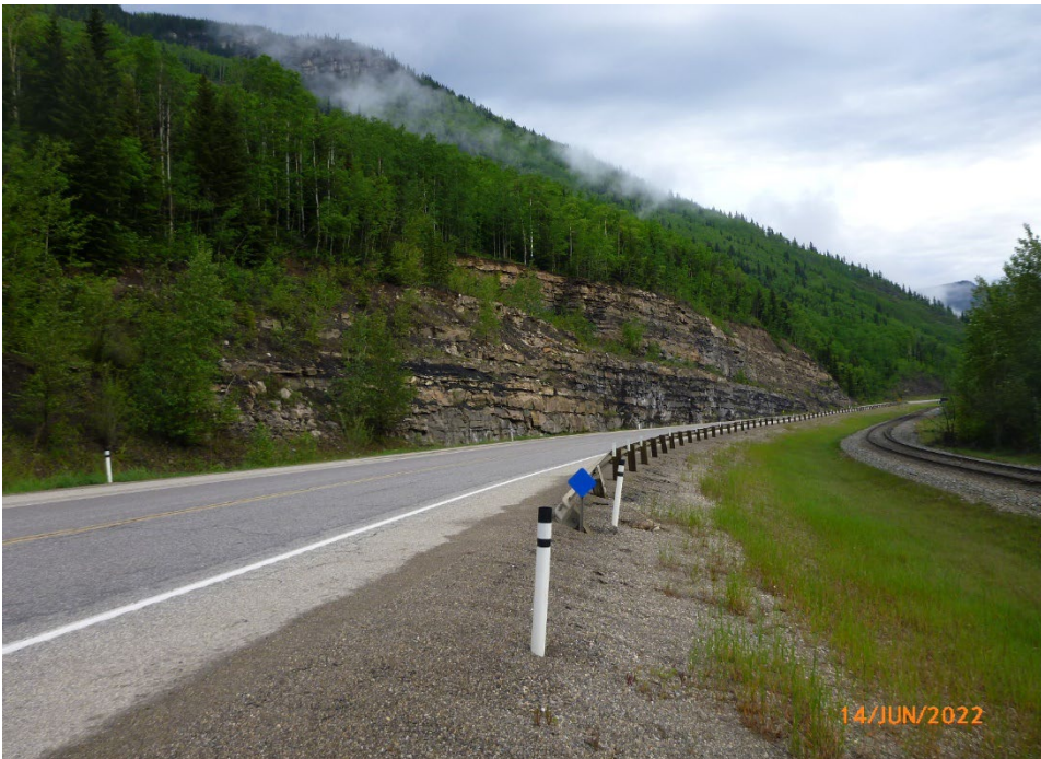
Photo 6 Near horizontal bedding of rock cut slope. Rock below mid-slope bench is massively bedded and competent. While rock above mid-slope bench is heavily fractured. Photo taken June 14, 2022, facing northwest.
