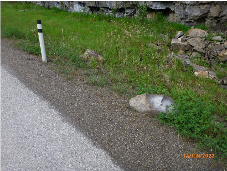
Photo 10 Rockfall particle near edge of southbound lane. Photo taken June 14, 2022 facing southwest.
