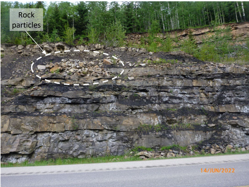
Photo 8 Talus materials and rockfall particles along mid-slope bench. Photo taken June 14, 2022, facing west.
