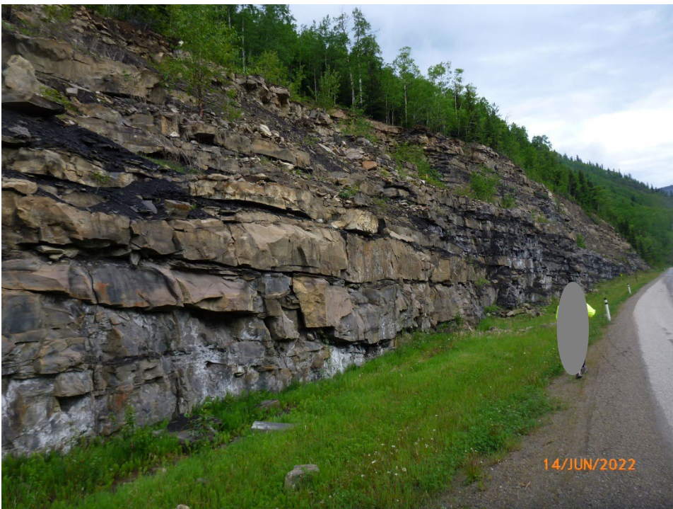
Photo 6 Near horizontal bedding of rock cut slope. Rock below mid-slope bench is massively bedded and competent. While rock above mid-slope bench is heavily fractured. Photo taken June 14, 2022, facing northwest.
