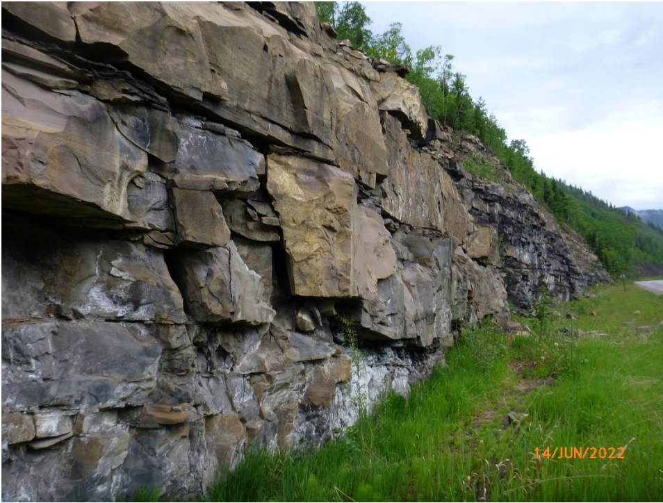
Photo 8 Talus materials and rockfall particles along mid-slope bench. Photo taken June 14, 2022, facing west.
