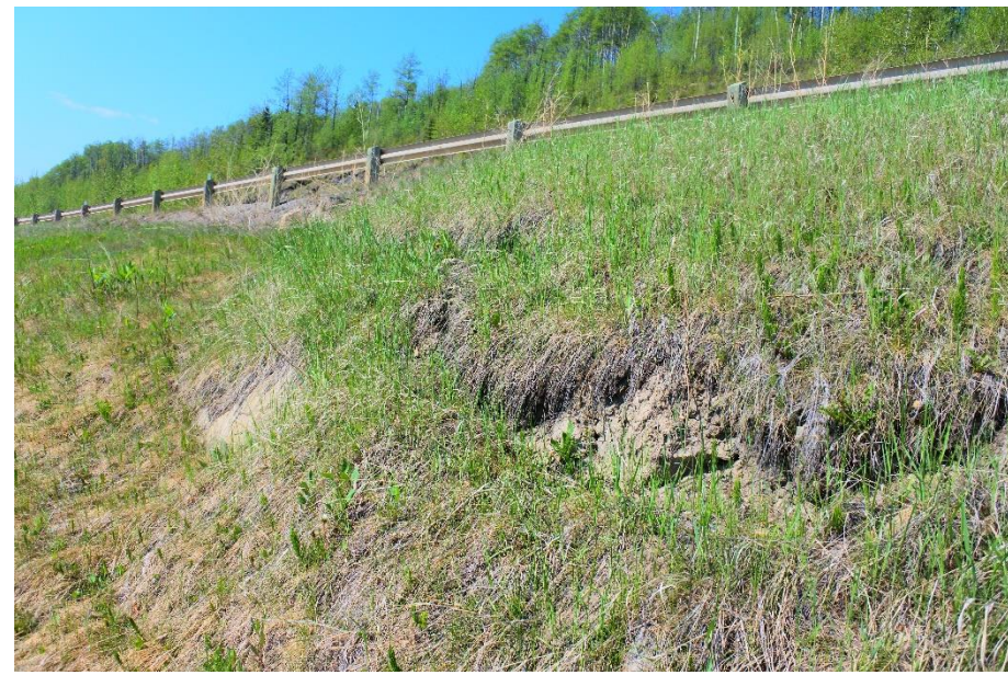
Photo 2. Looking southwest at scarp heading towards guardrail.
