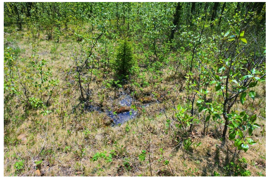
Photo 5. Looking south of the bin wall at ponded water downslope of scarp.
