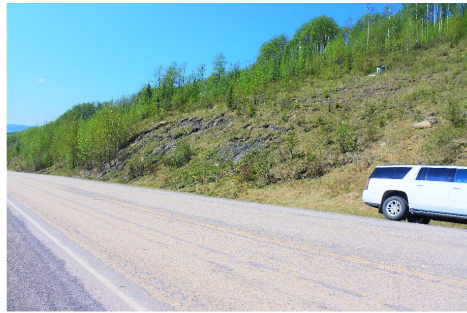
Photo 4. Looking west towards the backslope and at manhole.
