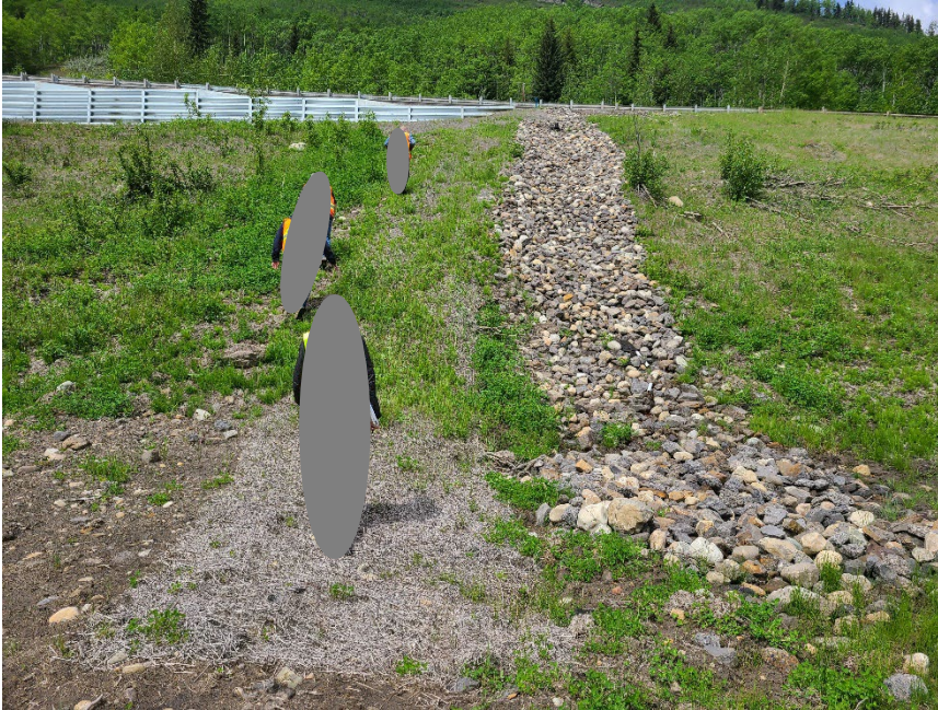
Photo 6 Connection between asphalt ditch between guardrail and binwall, and top of riprap-lined channel at north end of binwall. Photo taken June 14, 2022, facing south.
