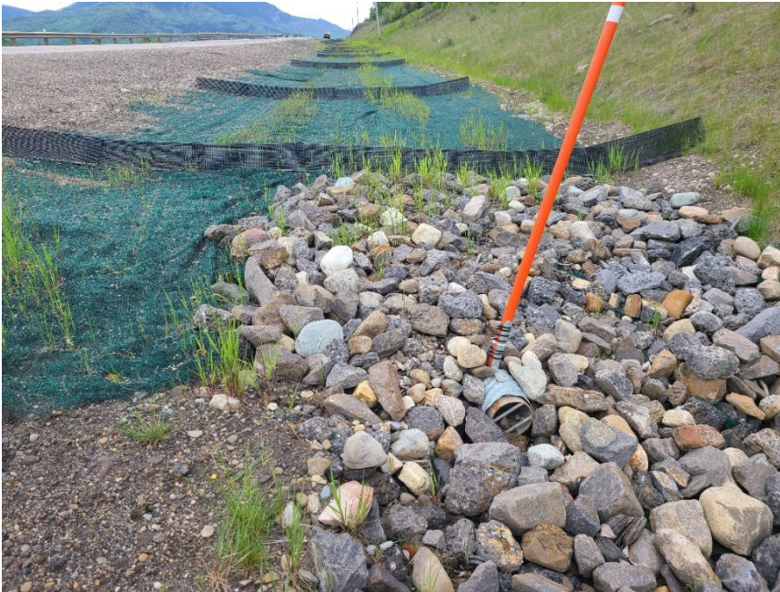
Photo 10 Inlet of CSP drainage gallery in upslope/west ditch of Hwy 40:36. Note inlet of CSP drainage gallery sticks up approximately 0.5 m above ditch bottom and is a potential roadside hazard to motorists who go off highway. Insulation around inlet is also deteriorating. Photo taken June 14, 2022, facing northeast.
