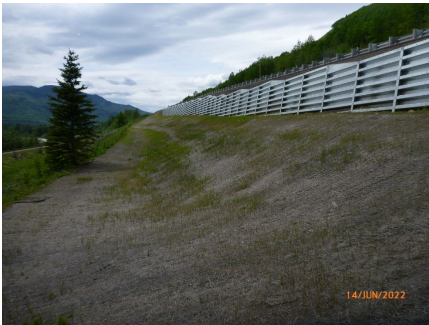
Photo 4 Binwall and mid-slope bench along downslope/east side of Hwy 40:36. Vegetation still establishing on slope and mid-slope bench. Photo taken June 14, 2022 facing southwest.
