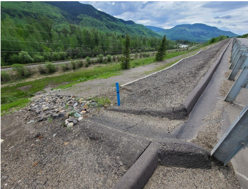
Photo 6 Connection between asphalt ditch between guardrail and binwall, and top of riprap-lined channel at north end of binwall. Photo taken June 14, 2022, facing south.
