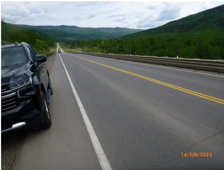
Photo 8 Some cracking in pavement surface of Hwy 40:36 likely due to binwall taking up load from slide mass. Photo taken June 14, 2022, facing north.
