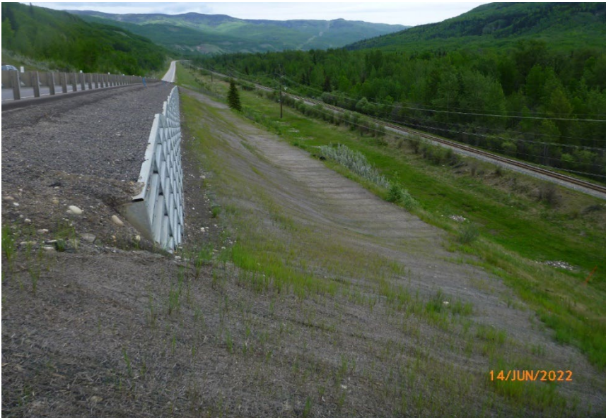
Photo 2 Toe of slope below highway and binwall. Photo taken June 14, 2022, facing northeast.
