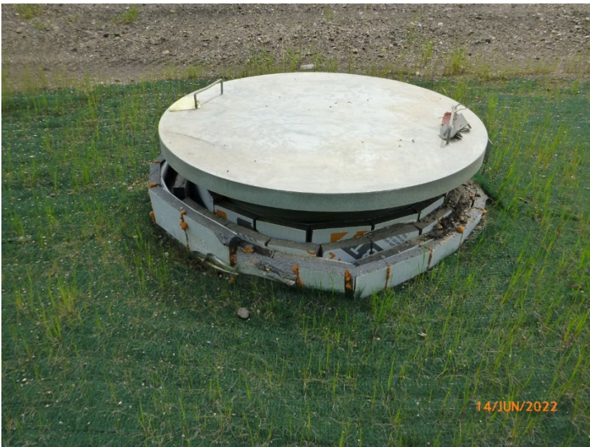
Photo 10 Inlet of CSP drainage gallery in upslope/west ditch of Hwy 40:36. Note inlet of CSP drainage gallery sticks up approximately 0.5 m above ditch bottom and is a potential roadside hazard to motorists who go off highway. Insulation around inlet is also deteriorating. Photo taken June 14, 2022, facing northeast.
