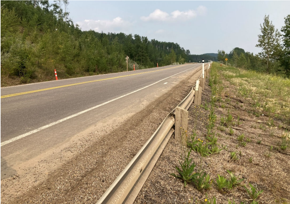
Photo 8 An area of the site that is regularly patched (shown in Photo 7) where the asphalt surface is near the top of the guardrail. Photo taken July 20, 2021 facing north.
