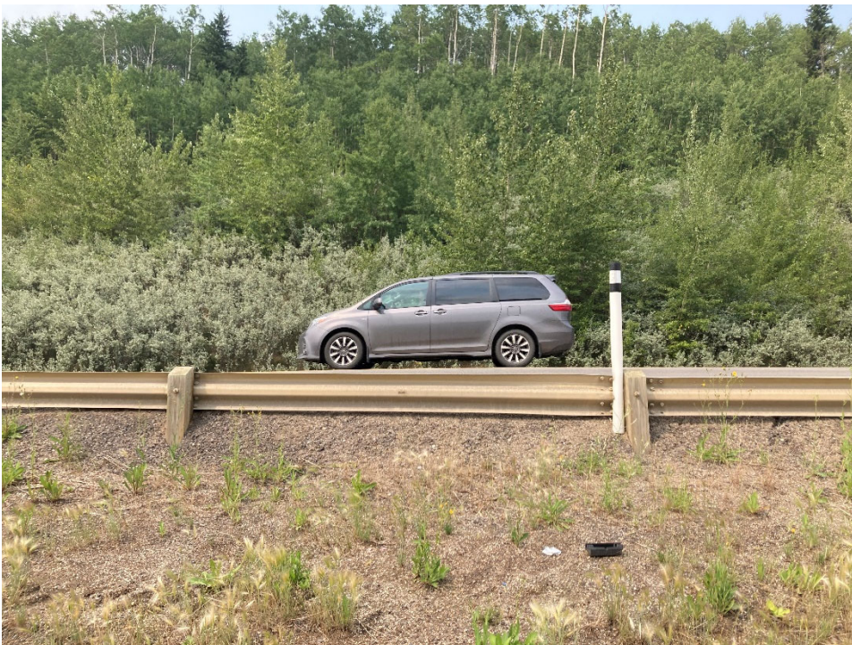
Photo 8 An area of the site that is regularly patched (shown in Photo 7) where the asphalt surface is near the top of the guardrail. Photo taken July 20, 2021 facing north.
