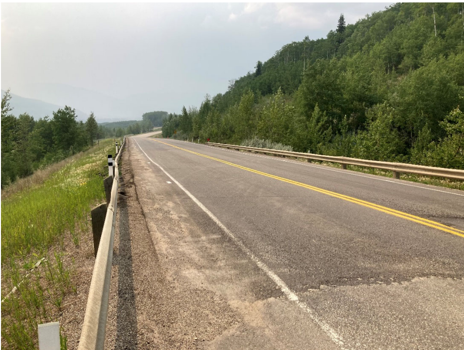
Photo 6 Asphalt patch near the east extent of the site that is typically repaved on an annual basis. Photo taken July 20, 2021 facing southwest.
