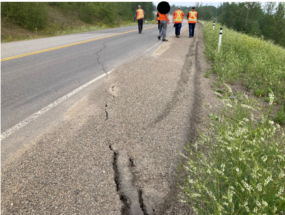
Photo 3 Asphalt cracking observed in the south (northbound) lane that extends from the edge of the highway to the centreline. Photo taken July 20, 2021 facing northeast.
