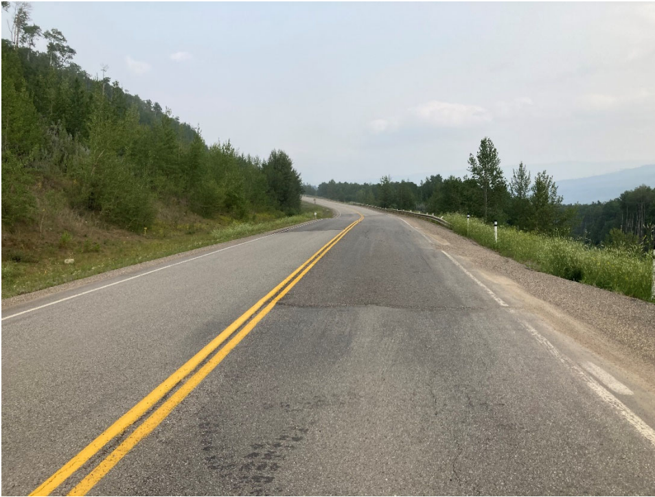
Photo 3 Asphalt cracking observed in the south (northbound) lane that extends from the edge of the highway to the centreline. Photo taken July 20, 2021 facing northeast.
