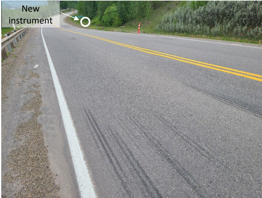
Photo 8 Seepage spot (circled in white) in southbound lane of Hwy 40:36 at eastern site limit. Photo taken June 14, 2022, facing south.
