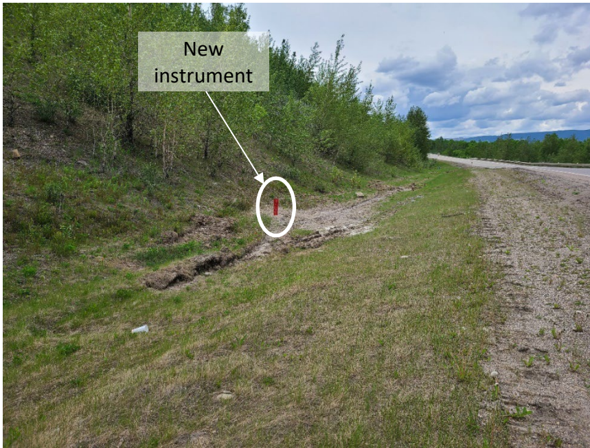
Photo 4 Sinkhole along fiber optics line (circled in white) in upslope/north ditch of Hwy 40:36 at WP208. Photo taken June 14, 2022, facing east.
