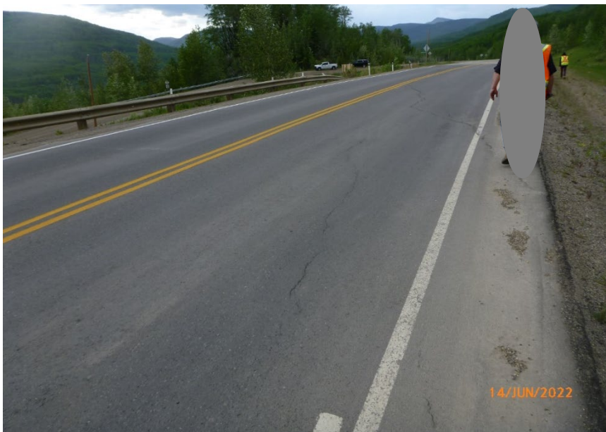
Photo 2 Cracking in recent pavement patch of Hwy 40:36 near western site limit. Photo taken June 14, 2022, facing southwest towards intersection with Wanyandie Road.
