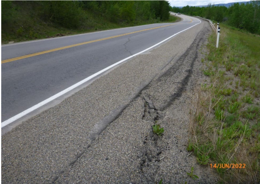
Photo 2 Cracking in recent pavement patch of Hwy 40:36 near western site limit. Photo taken June 14, 2022, facing southwest towards intersection with Wanyandie Road.
