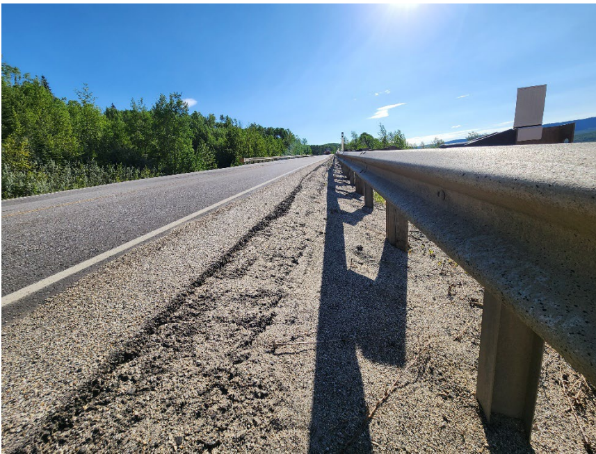
Photo 8 Guardrail on south side of Hwy 40:36 at east end of GP007 site is low and located far from highway. Photo taken June 2, 2025, facing east.
