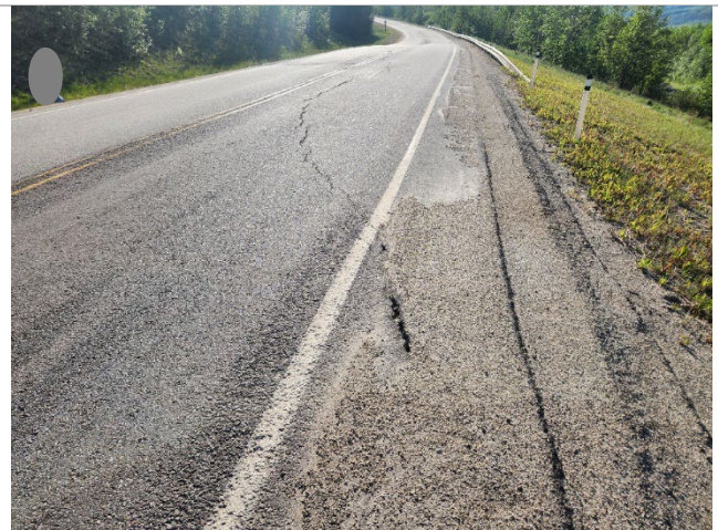
Photo 2 Cracking and settlement across pavement surface of Hwy 40:36 near west end of GP007 site. Photos taken June 2, 2025, facing southwest and east, respectively.
