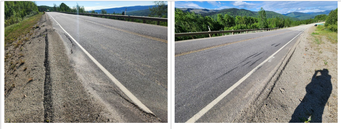
Photo 8 Guardrail on south side of Hwy 40:36 at east end of GP007 site is low and located far from highway. Photo taken June 2, 2025, facing east.
