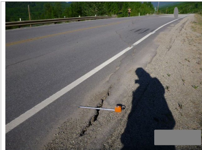
Photo 2 Cracking and settlement across pavement surface of Hwy 40:36 near west end of GP007 site. Photos taken June 2, 2025, facing southwest and east, respectively.
