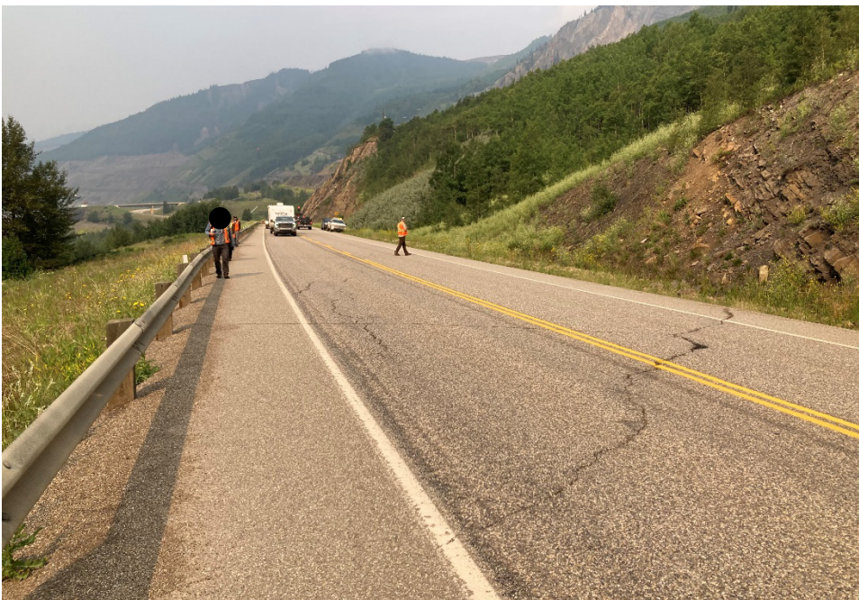
Photo 6 Asphalt cracking at the North Slide site approximately 150 m east of the debris flow site, extending from the edge of the eastbound lane to the edge of the westbound lane. Photo taken July 21, 2021 facing west.
