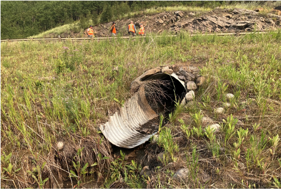
Photo 8 Riprap lined outlet channel for the 900 mm diameter CSP culvert. Photo taken July 21, 2021 facing south.
