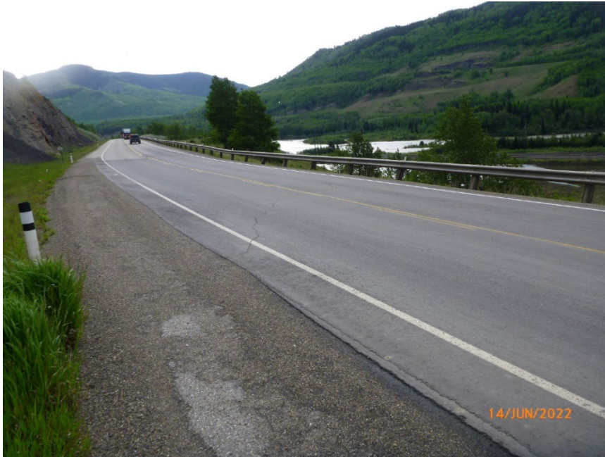
Photo 4 Cracking in pavement surface/patch of Hwy 40:36 above middle slide area at WP193. Photo taken June 14, 2022, facing west.
