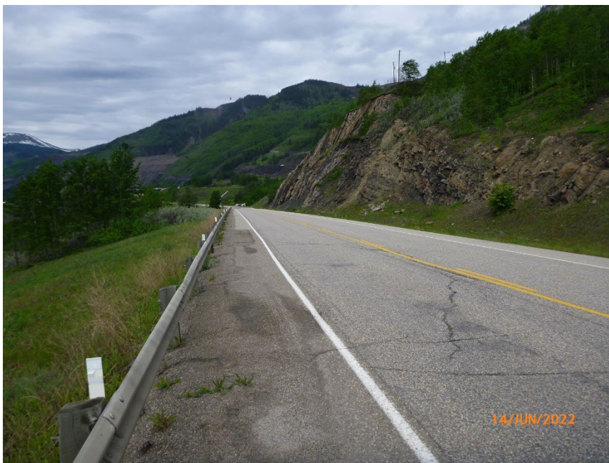
Photo 4 Cracking in pavement surface/patch of Hwy 40:36 above middle slide area at WP193. Photo taken June 14, 2022, facing west.
