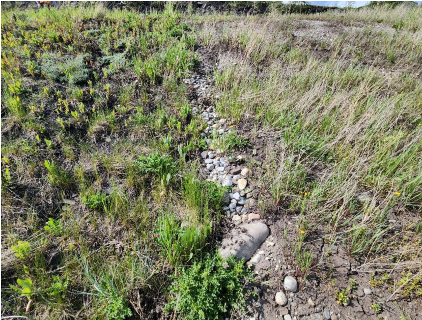
Photo 12 Slope between repaired ATCO slide and rail line. Note outlet of drainpipe (circled in white) installed in 2024 to convey flow from within the slide zone. Photos taken June 2, 2025, facing southeast and southwest, respectively.
