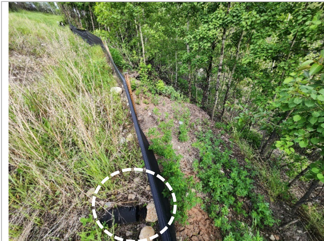
Photo 12 Slope between repaired ATCO slide and rail line. Note outlet of drainpipe (circled in white) installed in 2024 to convey flow from within the slide zone. Photos taken June 2, 2025, facing southeast and southwest, respectively.
