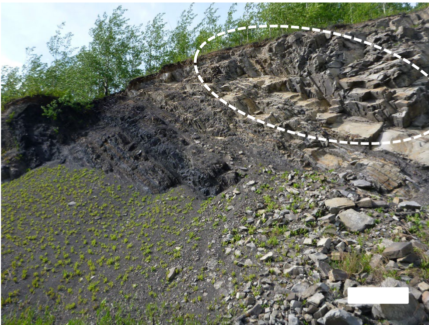
Photo 8 Rock slope along north side of Hwy 40:36 at GP053-II site. Note overhanging rock blocks (circled in white). Photo taken June 2, 2025, facing northwest.
