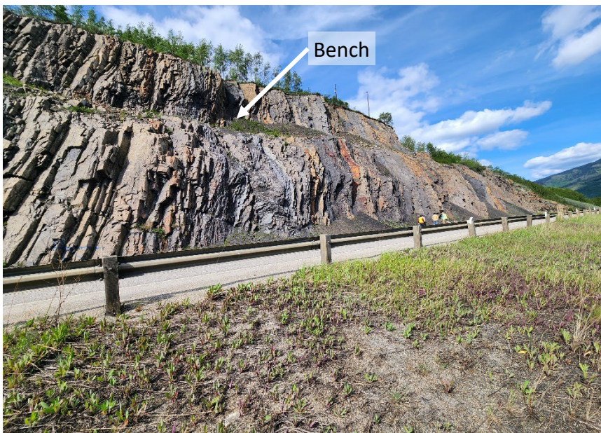
Photo 2 Rock slope along north side of Hwy 40:36 at GP053-I site. Note bench which could launch rockfall particles from upper slope. Photo taken June 2, 2025, facing northeast.
