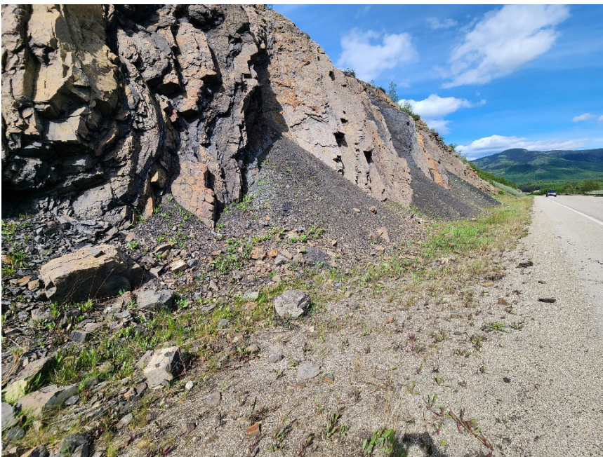
Photo 4 Rock slope along north side of Hwy 40:36 at GP053-I site. Note talus material mainly from coal seams in highway ditch. Photo taken June 2, 2025, facing northeast.
