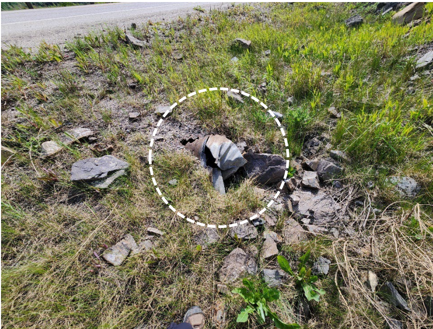
Photo 6 Culvert inlet (circled in white) in west ditch of Hwy 40:36 damaged and partially blocked with rocks. Photo taken June 2, 2025.
