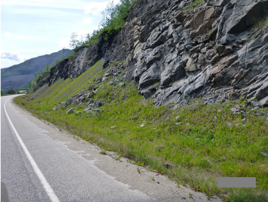
Photo 8 Rock slope along north side of Hwy 40:36 at GP053-II site. Note overhanging rock blocks (circled in white). Photo taken June 2, 2025, facing northwest.
