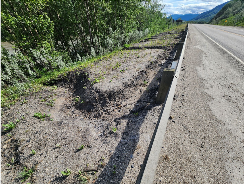
Photo 6 Subgrade exposed and edge of pavement partially undermined on east side of Hwy 40:36. Some guardrail posts also unsupported. Photo taken June 2, 2025, facing southwest.
