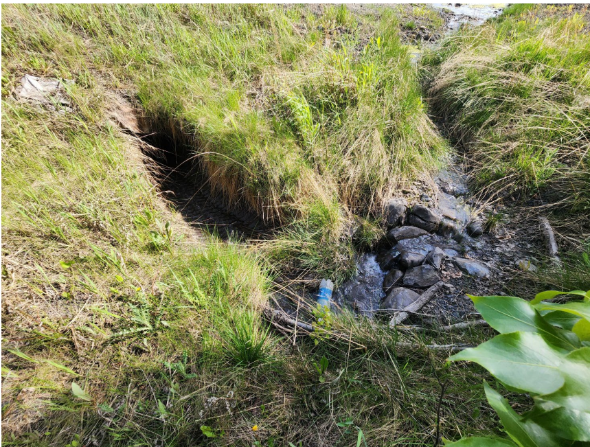
Photo 4 Inlet of culvert that conveys flow from west side to east side of Hwy 40:36. Photo taken June 2, 2025, facing south.
