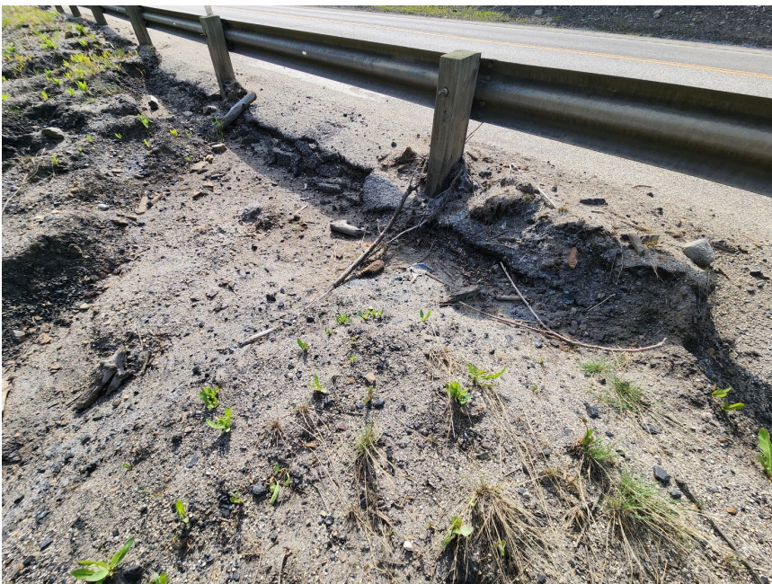
Photo 6 Subgrade exposed and edge of pavement partially undermined on east side of Hwy 40:36. Some guardrail posts also unsupported. Photo taken June 2, 2025, facing southwest.
