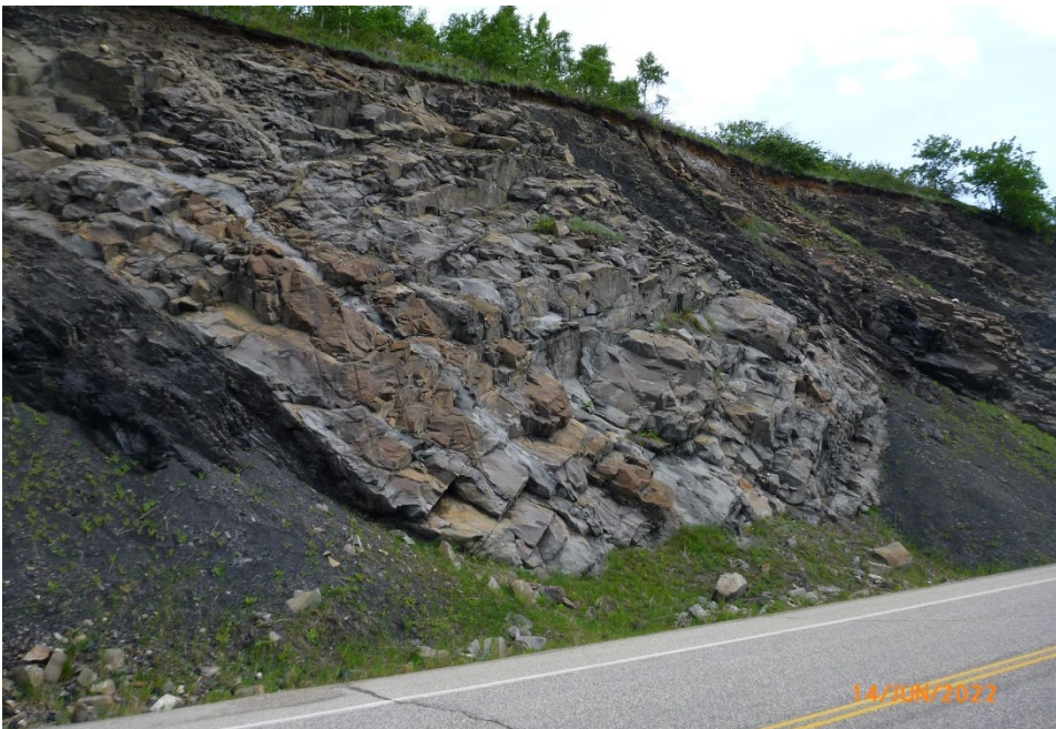
Photo 11 Rock cut slope near WP195 and middle of site. Note rockfall particles in upslope/north highway ditch, which is narrow and shallow. Photo taken June 14, 2022, facing northeast.
