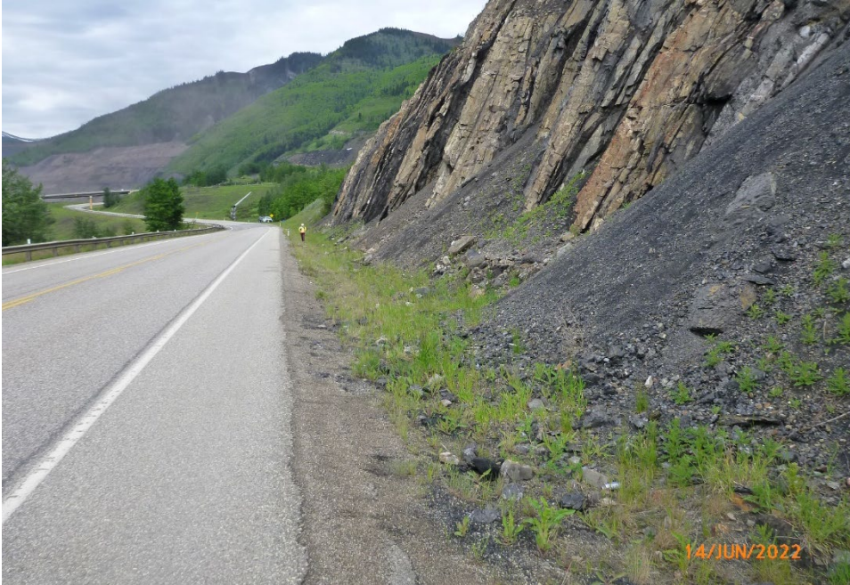
Photo 5 Toe of rock cut slope between WP190 and WP191 at south/western site limit. Note rockfall particles in upslope/north highway ditch. Photo taken June 14, 2022, facing east.
