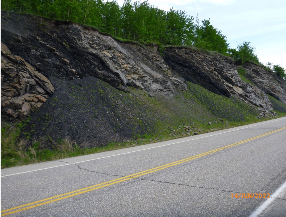
Photo 11 Rock cut slope near WP195 and middle of site. Note rockfall particles in upslope/north highway ditch, which is narrow and shallow. Photo taken June 14, 2022, facing northeast.
