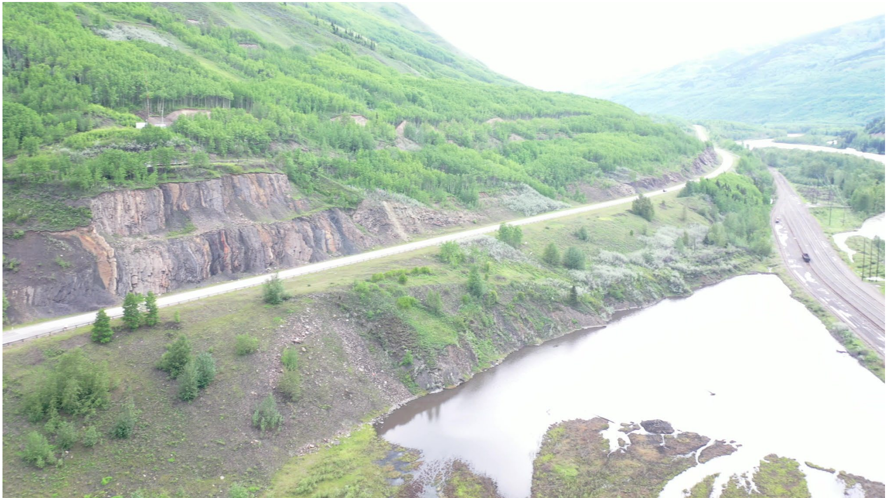
Photo 1 Overview of rockfall corridor along west side of Hwy 40:36 north of McIntyre Mine. Photo taken June 14, 2022, with unmanned aerial vehicle (UAV) facing northeast.
