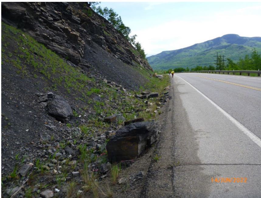
Photo 13 Large rockfall particle in upslope/west ditch between WP195 and WP196 near northern site limit. Photo taken June 14, 2022, facing east.
