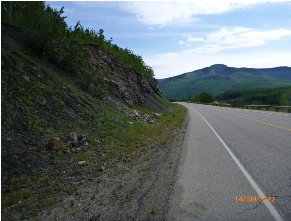
Photo 9 Rock cut slope near WP195 and middle of site. Note talus (coal) materials and rockfall particles in upslope/north highway ditch, which is narrow and shallow, and hanging rock blocks. Photo taken June 14, 2022, facing north.
