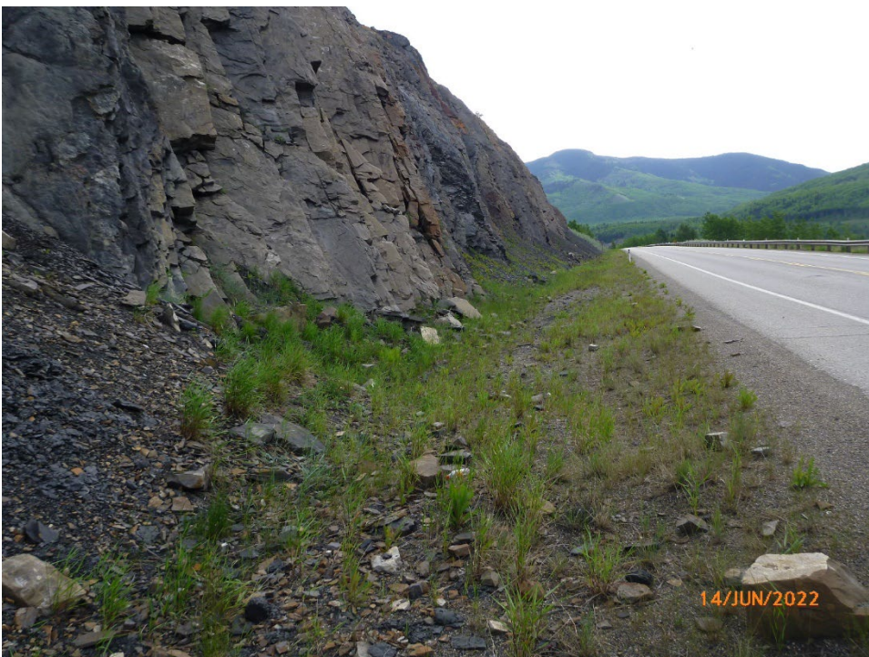
Photo 5 Toe of rock cut slope between WP190 and WP191 at south/western site limit. Note rockfall particles in upslope/north highway ditch. Photo taken June 14, 2022, facing east.
