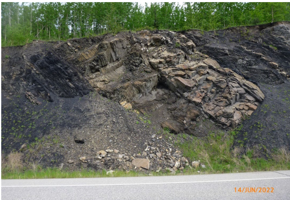
Photo 9 Rock cut slope near WP195 and middle of site. Note talus (coal) materials and rockfall particles in upslope/north highway ditch, which is narrow and shallow, and hanging rock blocks. Photo taken June 14, 2022, facing north.
