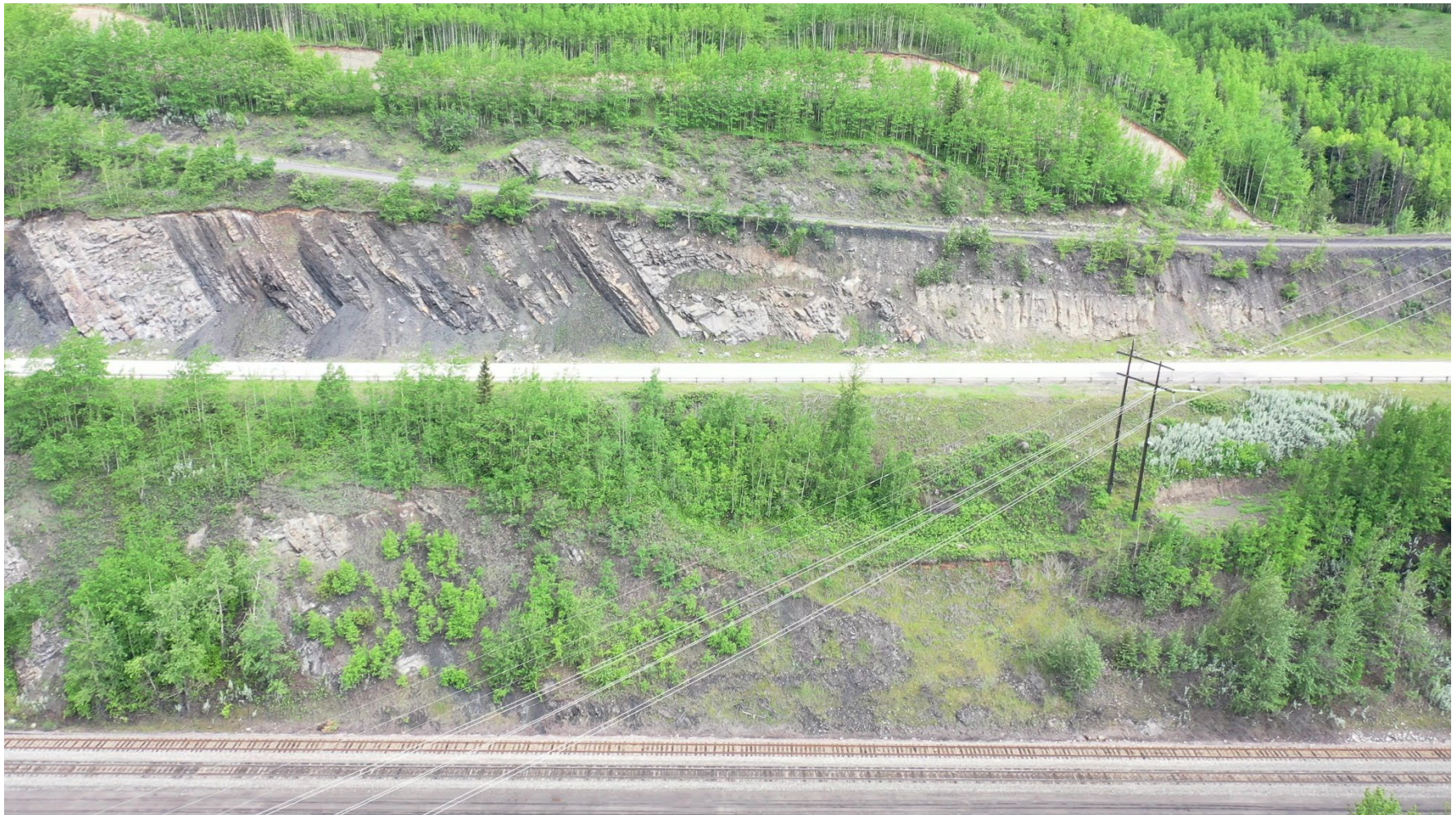
Photo 3 Rock cut slope along west side of Hwy 40:36 at WP 197 at north/eastern site limit. Note talus (coal) deposits and rockfall particles in upslope/north highway ditch. Photo taken June 14, 2022, with UAV facing north.
