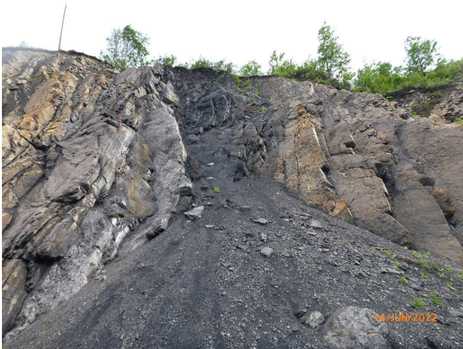
Photo 7 Talus material from coal seam in rock cut slope between WP190 and WP191 at south/western site limit. Photo taken June 14, 2022, facing north.
