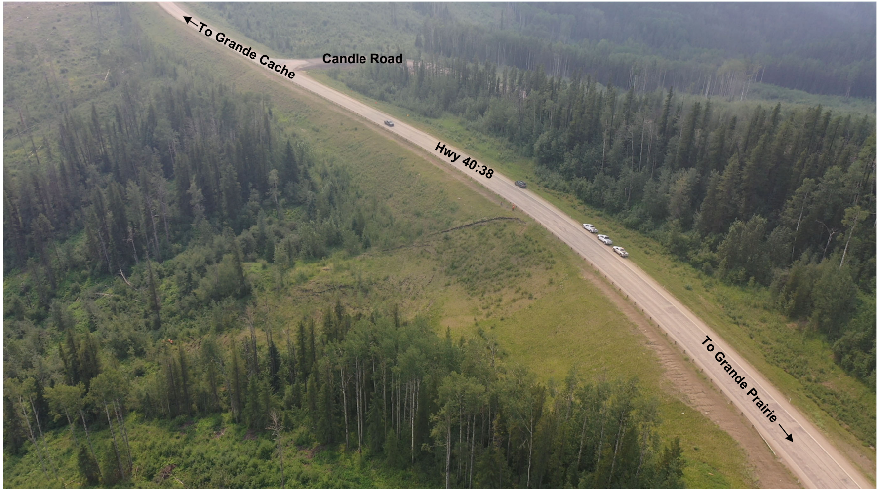
Photo 1 Overview of the GP002 site, indicating Hwy 40, Candle Road. Photo taken July 20, 2021 facing south.
