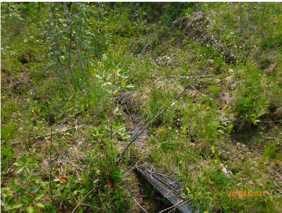
Photo 3 Exposed silt fencing near the toe of the slide (Waypoint 94). Photo taken July 20, 2021 facing north.
