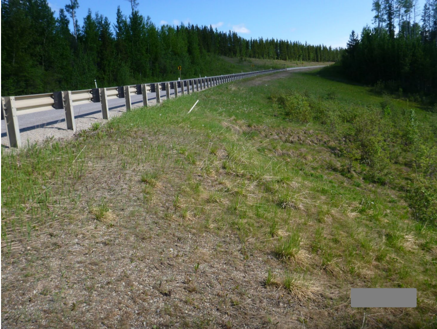
Photo 2 Slide backscarp on east side of Hwy 40:38. Photo taken June 3, 2025, facing south.
