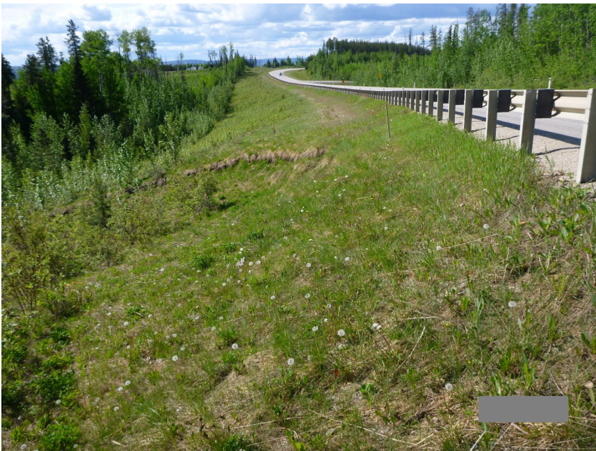
Photo 2 Slide backscarp on east side of Hwy 40:38. Photo taken June 3, 2025, facing south.
