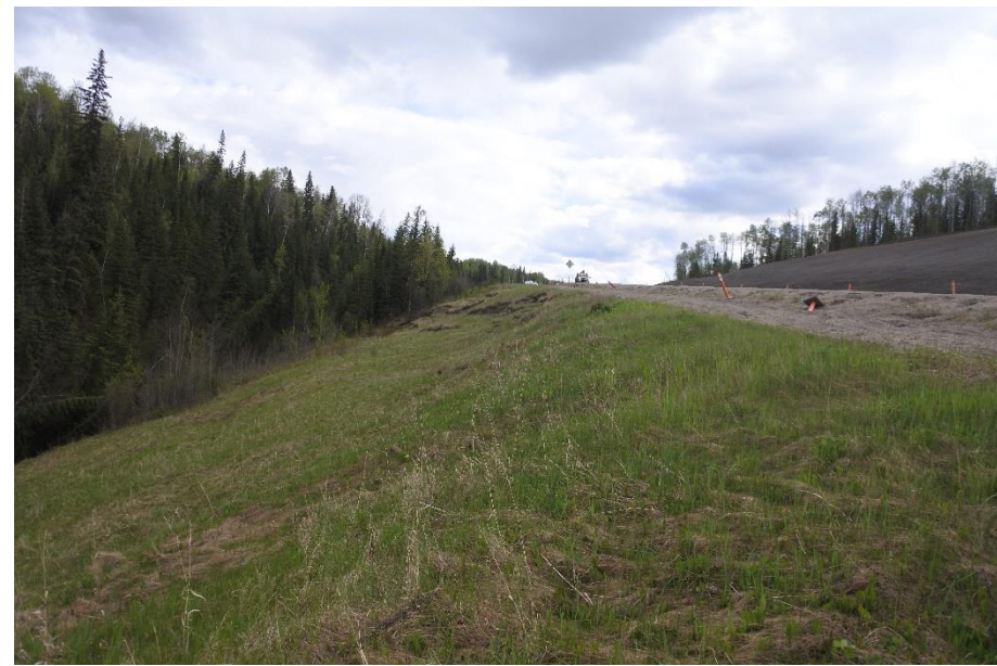
Photo 6. Looking south towards middle of the site where tilted trees are present.
