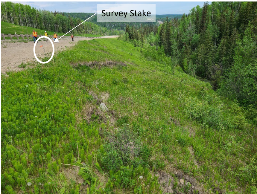
Photo 11 Slides scarps between Hwy 40:38 and Roseham Creek). Note reference/survey stake with flagging (circled in white) placed 1.0 m upslope of slide scarp to monitor retrogression at WP221. Photo taken June 15, 2022, facing north.
