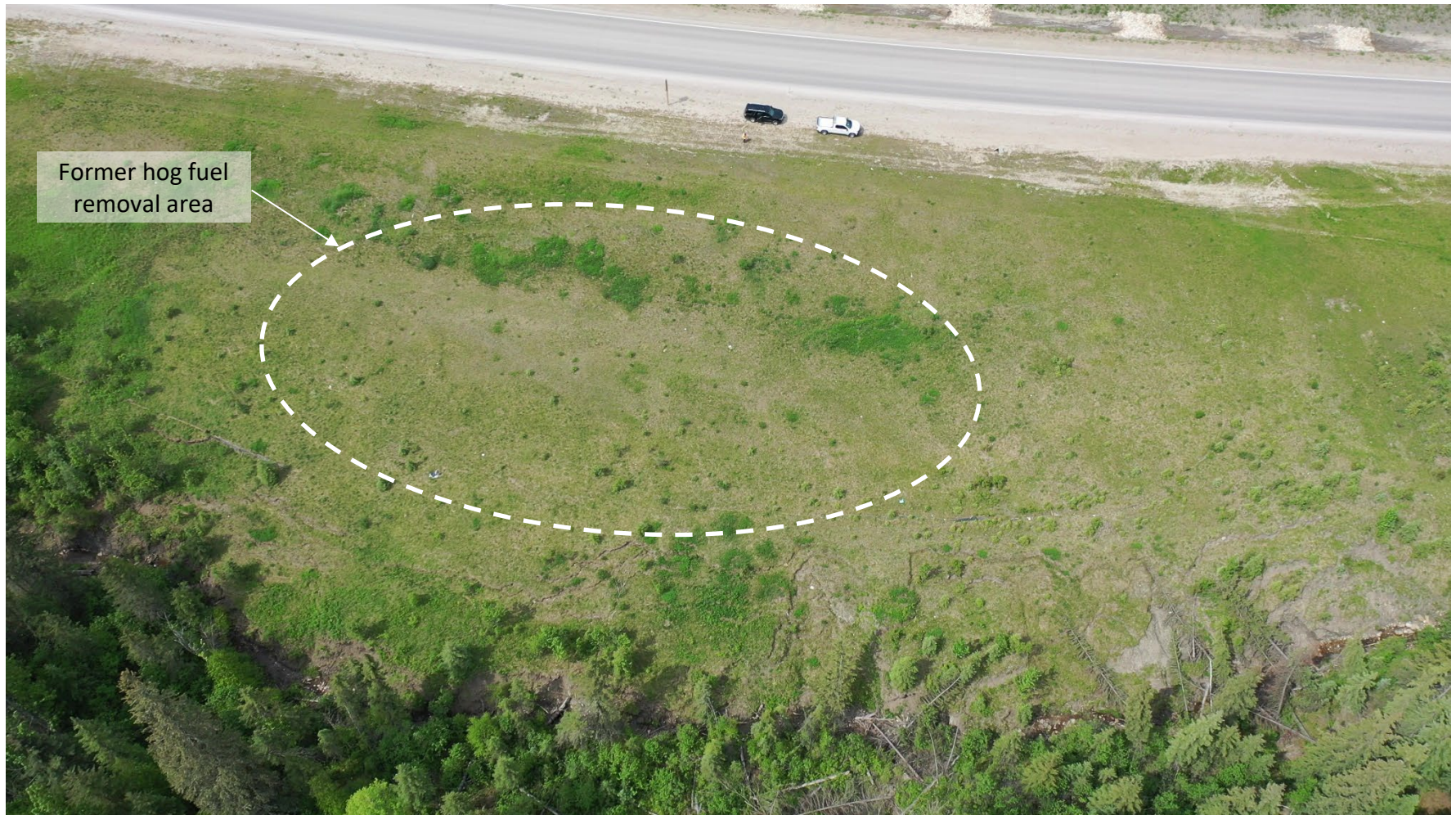
Photo 3 Former hog fuel removal area (circled in white) downslope/east of Hwy 40:38 and WP214. Series of slides along Roseham Creek. Photo taken June 15, 2022, with UAV facing down/west.
