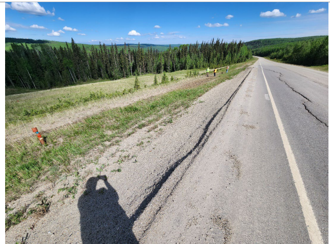
Photo 2 Cracking through pavement surface of Hwy 40:38. Photos taken June 2, 2025, facing southwest and northwest, respectively.
