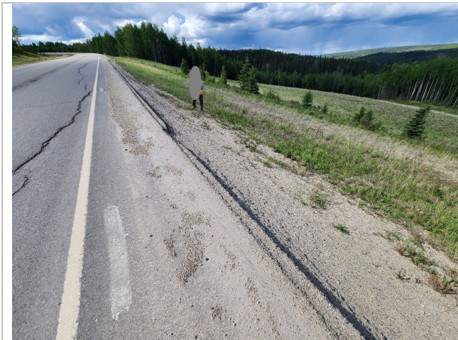
Photo 2 Cracking through pavement surface of Hwy 40:38. Photos taken June 2, 2025, facing southwest and northwest, respectively.
