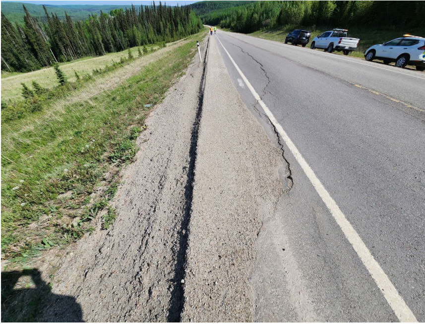
Photo 2 Cracking through pavement surface of Hwy 40:38. Photos taken June 2, 2025, facing southwest and northwest, respectively.
