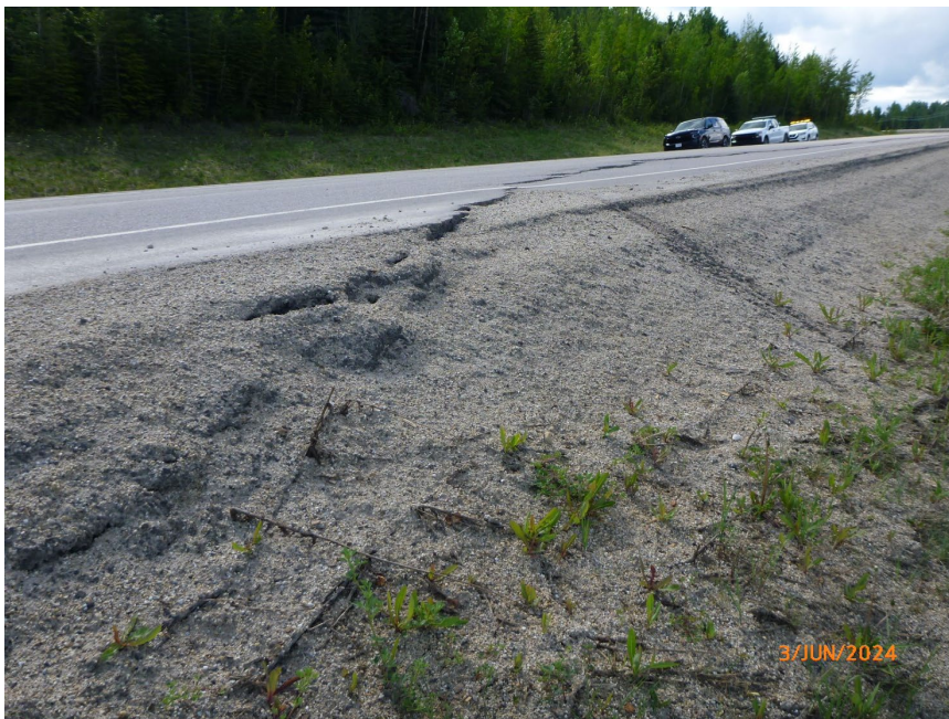
Photo 4 Cracking through pavement surface of Hwy 40:38. Photo taken June 2, 2025, facing southeast.
