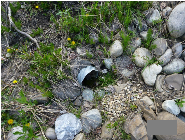
East drain at toe of toe berm.
