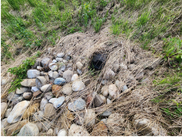
East drain at toe of toe berm.
