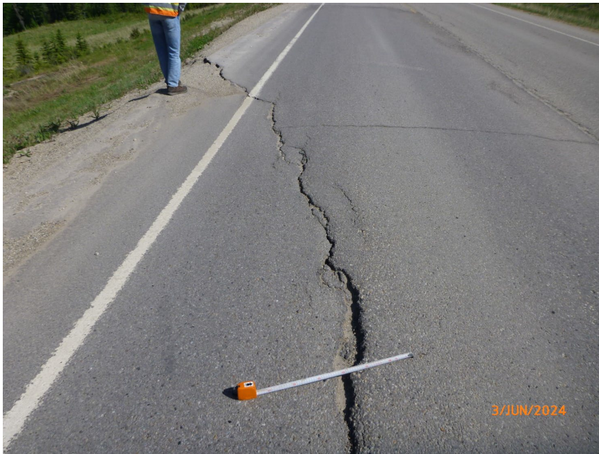
Photo 4 Cracking through pavement surface of Hwy 40:38. Photo taken June 2, 2025, facing southeast.
