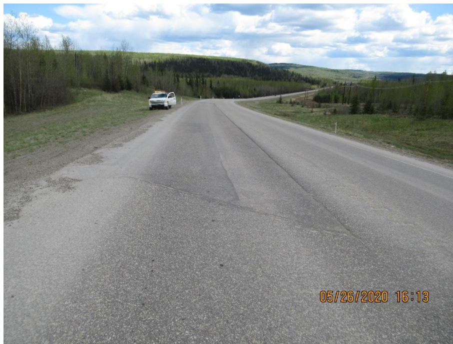
Photo 3. Looking south at most recent ACP patch where slide was repaired.
