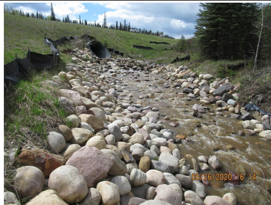
Photo 5. Looking west at the 3 m diameter SPCSP outlet, plunge pool, and east highway embankment.
