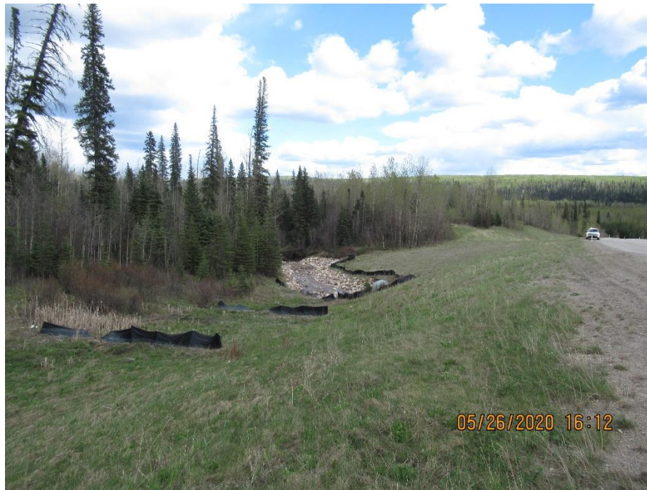
Photo 1. Looking south at culvert outlet and where slide has been replaced with fill and new ACP patch.
