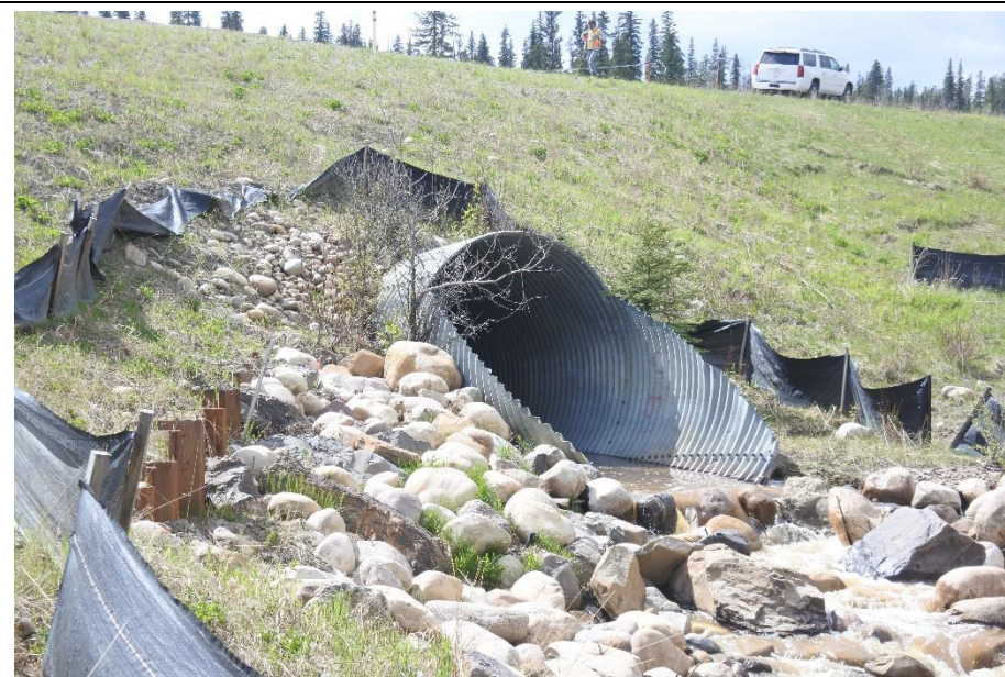
Photo 6. Looking west at the 3 m diameter SPCSP outlet, riprap and top of sheet pile wall.
