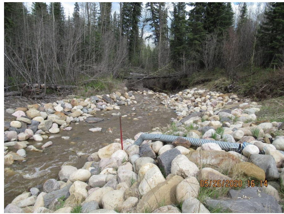
Photo 7. Looking east at where the subdrain pipe has disconnected.
